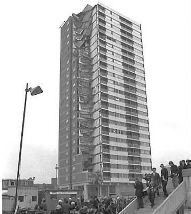
Figure 2.4: Ronan Point Collapse
