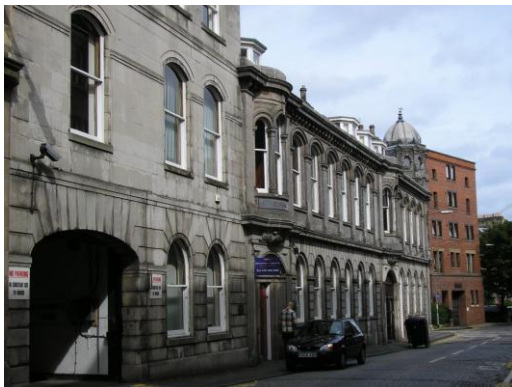
Figure 45 – Converted warehouse on Maritime Street (L on Map 15) (photo: author).
