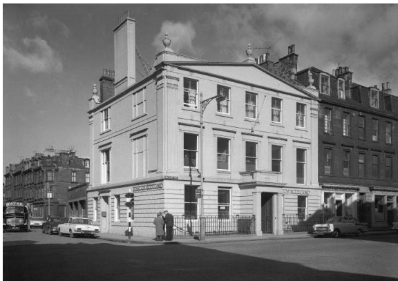
Figure 28 – Late 18 th century merchant's house on Constitution Street ( Y on Map 15 ). With its rusticated ground floor and giant Corinthian pilasters topped with urns, this was the grandest late 18th-century house in Leith (SCRAN, 2009) (photo: c. 1970s © RCAHMS, Licensor www.scran.ac.uk ).
