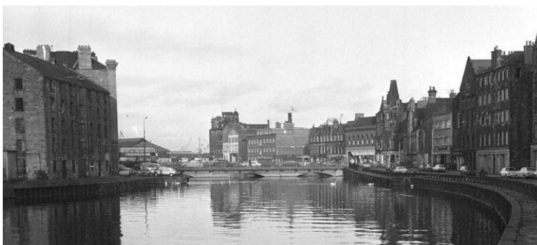
Figure 33 – View of the Shore in 1975. This view shows a tall continuous frontage displaying a variety of building forms and styles (photo: Stan Warburton, 1975 © RCAHMS, Licensor www.scran.ac.uk).
