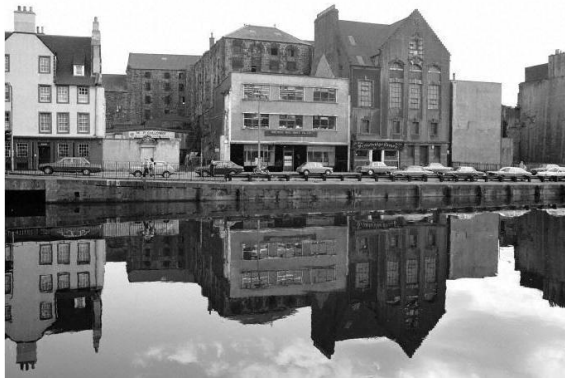
Figure 31 - Two existing gap sites on the Shore in the late 1970s. The one to the left still retained the ground floor of an early 18 th century tenement (SCRAN, 2009) (photo: John Hume, c. 1970 © RCAHMS, Licensor www.scran.ac.uk).
