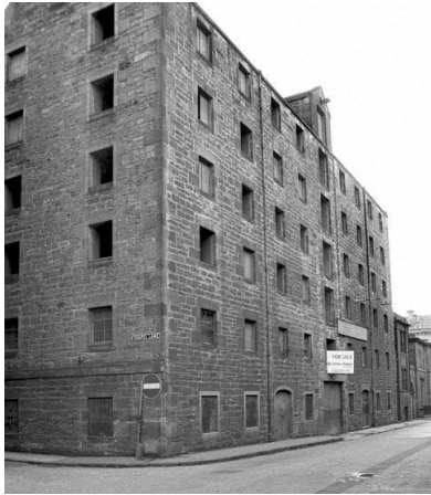
Figure 10 – Early to mid 19 th century warehouse on Chapel Lane and Maritime Street ( H on Map 15 ). This very large rubble-built warehouse was constructed as a grain store in the early-to-mid 19 th century (SCRAN, 2009) (photo: John Hume, 1970 © RCAHMS, Licensor www.scran.ac.uk ).
