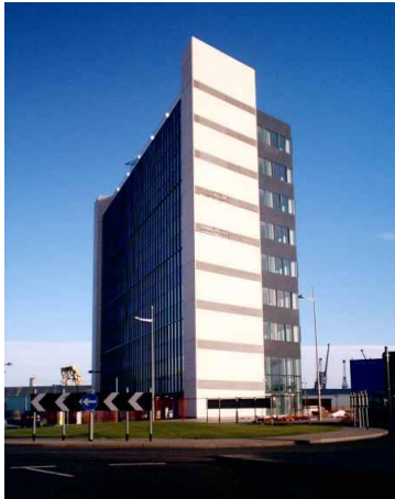
Figure 71 – Ocean Point office development next to Ocean Terminal (U on Map 22) (photo: Adrian Welch, © Edinburgh Architecture).
