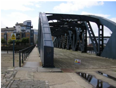
Figure 73 – Restored swing-bridge and winches at the entrance to the Old East Dock (C on Map 17) (photos: author).
