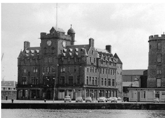
Figure 29 – Sailors' Home on the Shore ( Z on Map 15 ). This grand Scottish Baronial building was built in 1885 to provide accommodation for sailors while they were in the port (SCRAN, 2009) (photo: John Hume, 1969 © RCAHMS, Licensor www.scran.ac.uk ).
