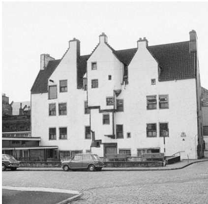
Figure 7 – Lamb's House, Water's Close ( E on Map 15 ). This merchant's house and warehouse was constructed in the early 17 th century. Its harling and crow-stepped gables are typical of late 16 th and early 17 th century merchants' houses in Scotland. It was restored in the mid 20 th century and converted into an old people's day centre (SCRAN, 2009) (photo: John Hume, 1970 © RCAHMS, Licensor www.scran.ac.uk ).
