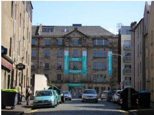
Figure 44 – Converted warehouse on Water Street (J on Map 15) (photo: author).
