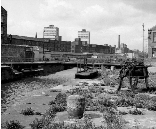
Figure 34 – Gate of the entrance lock at the Old East Dock, with the swing bridge beyond and associated winches and capstans in the foreground (C on Map 17). Both gate and bridge were installed in 1842-4 as replacements for John Rennie's originals. The East and West Docks were filled in c. late 1960s – early 1970s, but this lock and bridge survived (SCRAN, 2009) (Photo: John Hume, 1969 © RCAHMS, Licensor www.scran.ac.uk).
