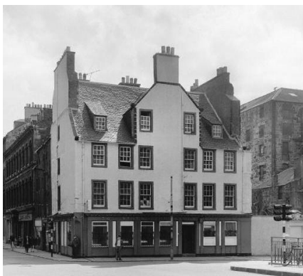
Figure 5 – King's Wark, the Shore (C on Map 15). This site was originally a food store and arsenal built for King James I in the 15 th century. In the 1970s, it was occupied by this early 18 th century tenement and public house (SCRAN, 2009) (photo: c. 1970s © RCAHMS, Licensor www.scran.ac.uk).
