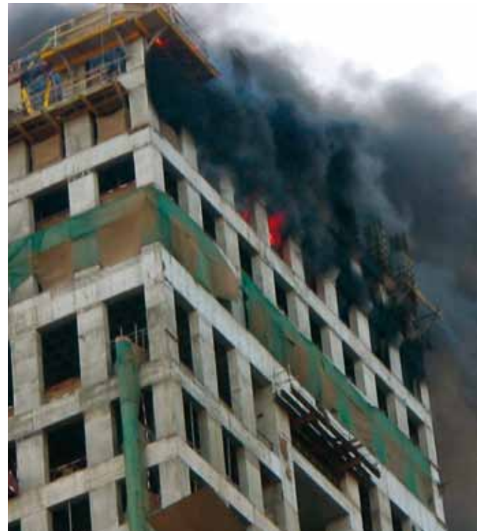
In a travelling fire, only a portion of a floor plate is fully involved in flames, which then move to other areas of the floor as burnout occurs
