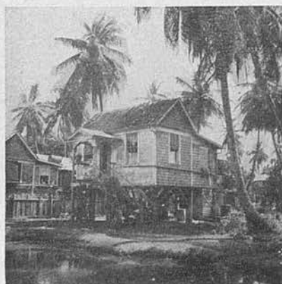
FIGURE 2. Types of Georgetown, B.G. Houses in Which Experiment on DDT Control Was Carried Out.
