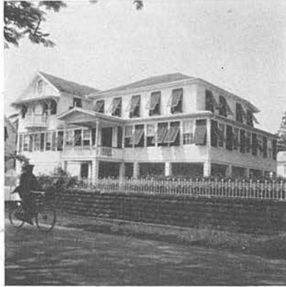
FIG. 1. TYPICAL LARGE HOUSE SHOWING ROOF-GUTTERS
