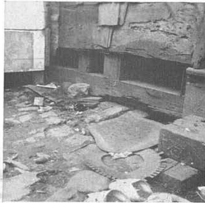
FIG. 11. UNDER THIS WOODEN FLOOR A LARGE GROUND POOL WAS FOUND
