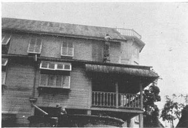
FIG. 5. CLEANING A ROOF-GUTTER
