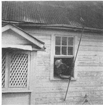
FIG. 4. INSPECTING A ROOF-GUTTER WITH A PERISCOPE MIRROR
