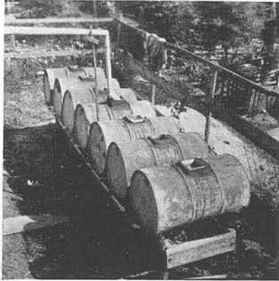
FIG. 7. DRUMS FOR WATER STORAGE
