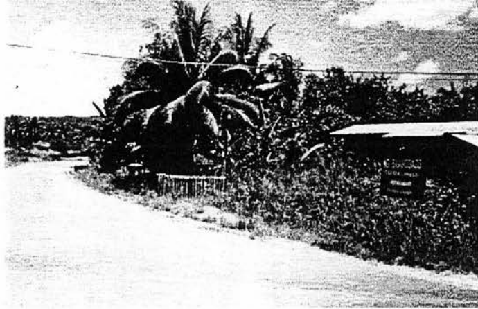
Signboard to Bavanggazo from the Kota Kinabalu-Kudat main road. Below, the rough gravel and stony road before the road works in late December 1996
