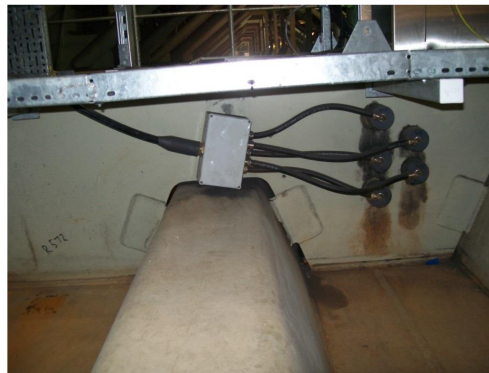
(c) Steel deck temperature sensors
