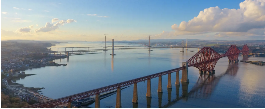
(a) The Forth Bridges ( www.theforthbridges.org )
