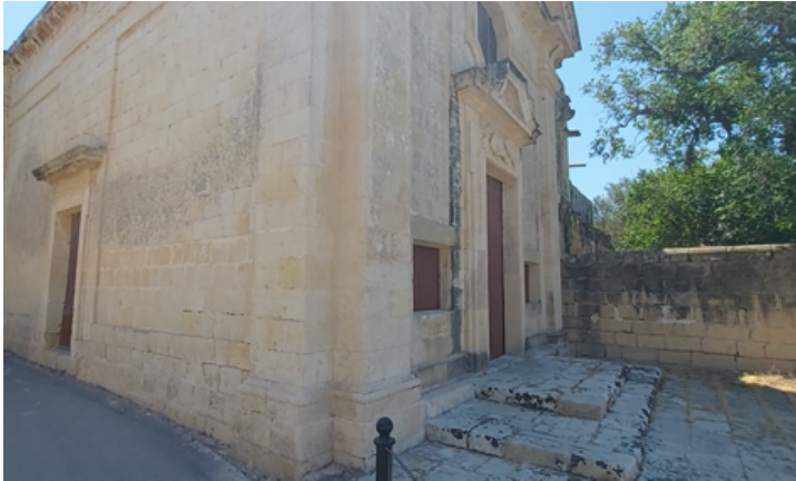
Figure 45: The chapel at Wied Qirda, Ғаз-Ғеббуғ.
