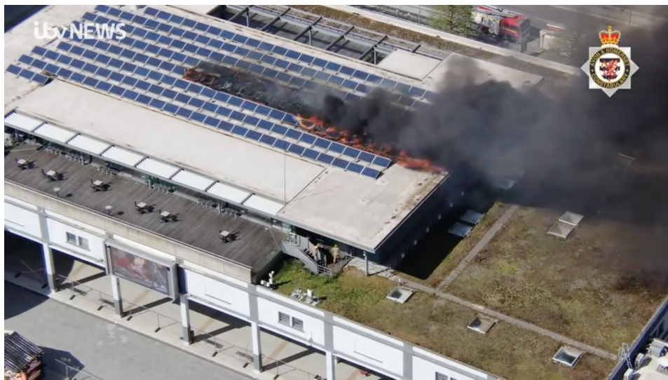
Figure 1.4: Video frame from drone video of the PV-related fire on the museum We The Curious in Bristol 2022. (Video: Avon and Somerset Police, from: [59])
