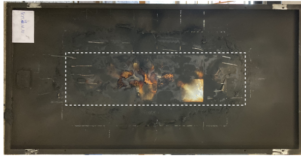
(a) Backside of PV module type 2 (see Table 3.2). The dotted line indicates the dimensions (37 cm times 118 cm) and the location of the roof construction mock-up below the module. Most of the polymer back sheet inside the dotted square was burned, and the white area was the transparent glass front sheet. The remaining part of the module was sooted, and the areas near the edge of the dotted lines were charred.
