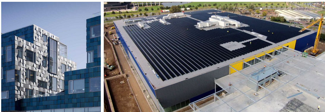
(c) PV integrated in façade. (d) Building applied PV system on top of IKEA warehouse in Zwolle (from: [27]) (NL). (from: [28])
