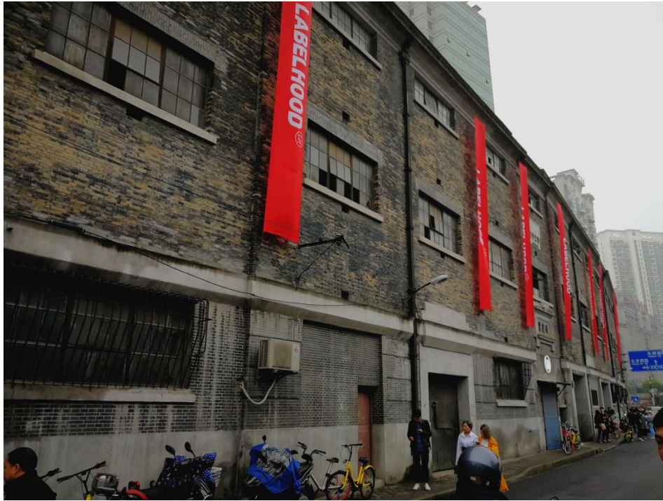
Figure 4.27: The 1929 British warehouse repurposed as the main venue for Labelhood since the Spring/Summer 2017 season (photographed by Wang, 2017)
