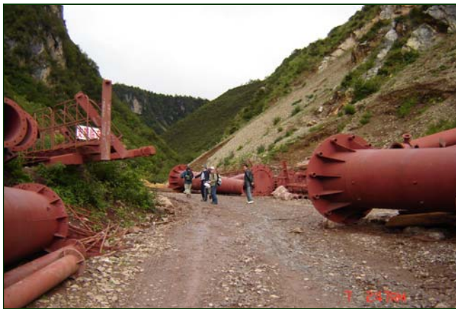
Photo 6 Building of a chairlift, Zhongdian Plateau
