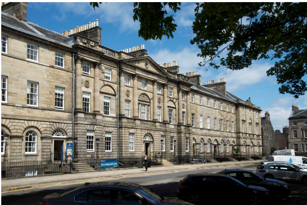
Figure 24. The north side of Charlotte Square in 2013 with leftmost dormer removed. Source: D. Henrie.
