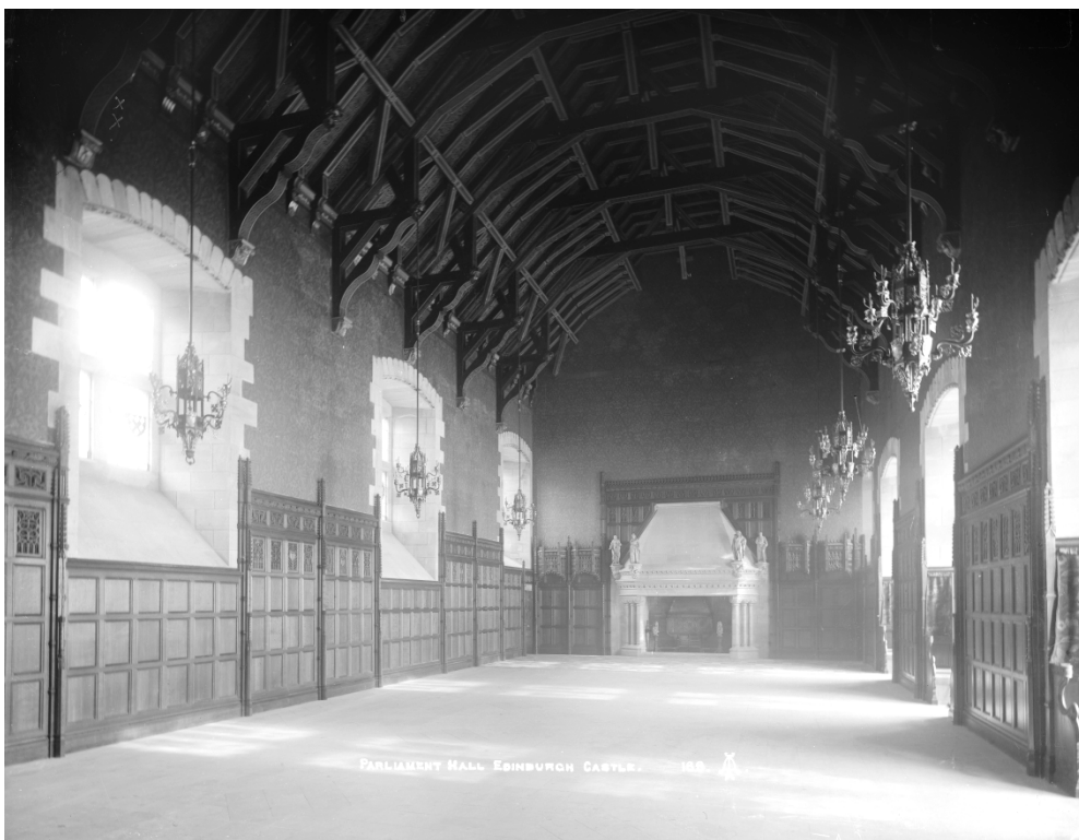
Figure 20. Edinburgh Castle, Great Hall in 1888 after restoration and before dressing. Source: RCAHMS SC 1201267.
