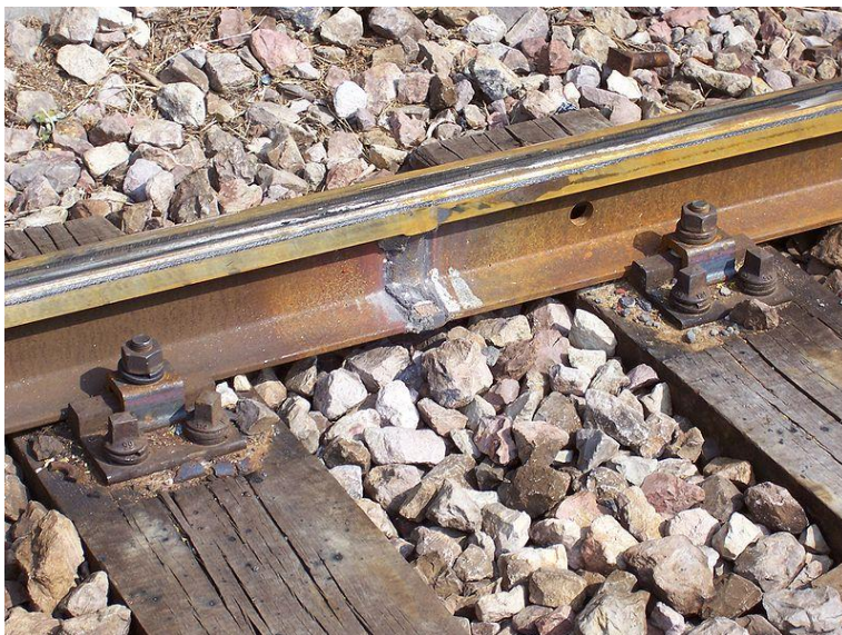
Figure 1.6 Continuous welded rail (Wikipedia, 2010)
