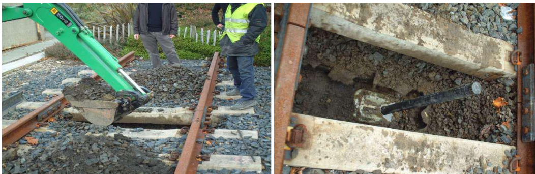
Figure 2.3 University of Edinburgh railway track excavation
