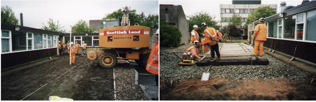
Figure 2.2 University of Edinburgh railway track construction
