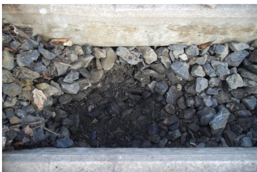
Figure 2.10 Crib 7: Some fines; built mixed
