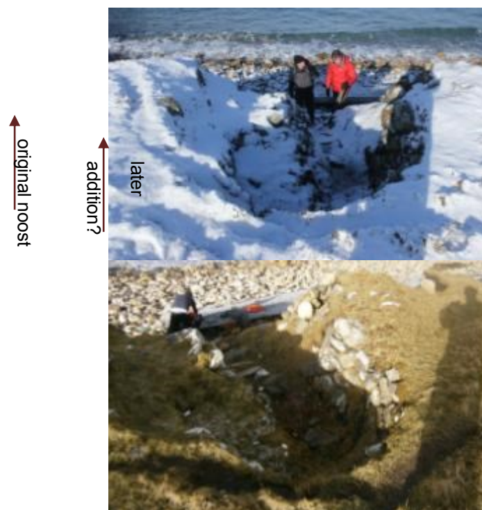
Figure 2-4: Photographs showing the modified noost (noost 1) on the foreshore of Underhoull Bay; illustrating the late construction of an internal wall to reduce the size of the primary noost. The vertical step from the noost floor to the current beach indicates significant erosion, beach instability and a possible reason for the noosts to fall into disuse.
