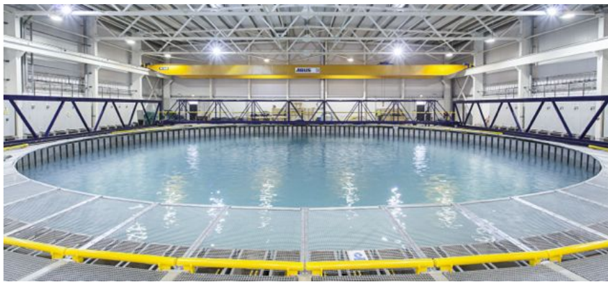
Figure 3.5: The FloWave Ocean Energy Research Facility.
