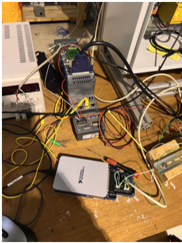
(c) Data acquisition system hardware.
