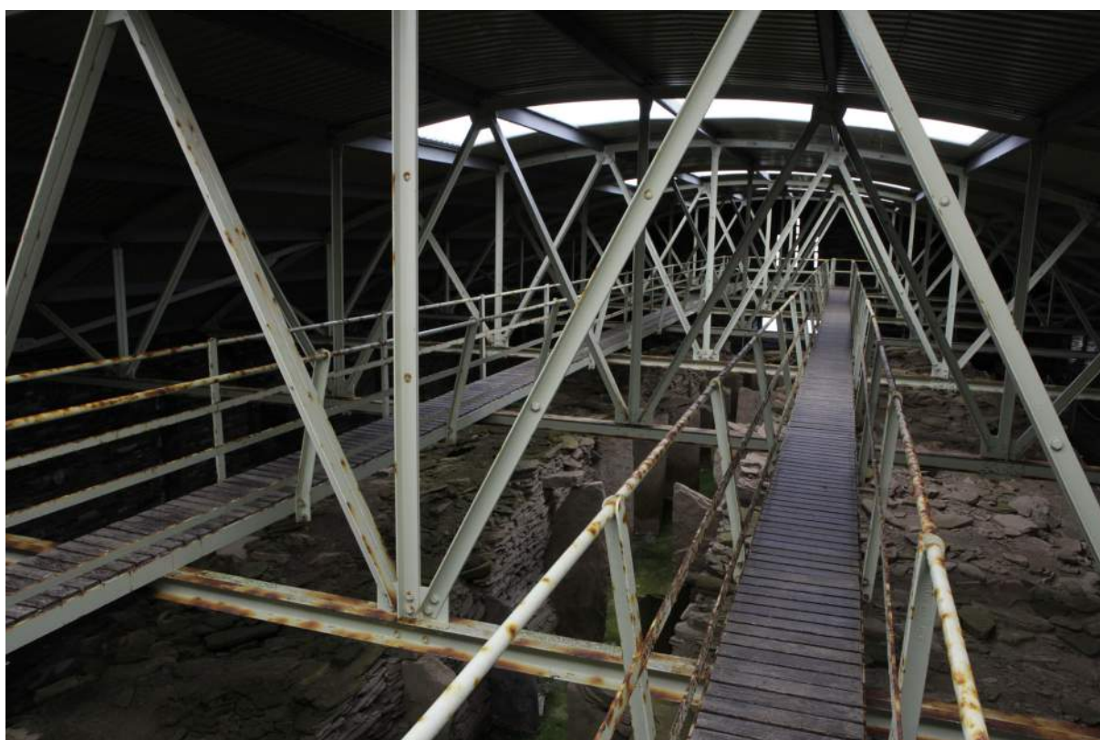
Figure A1: Free-standing protective steel enclosure over Midhowe, with elevated gangways from which to view the interior of the tomb.
