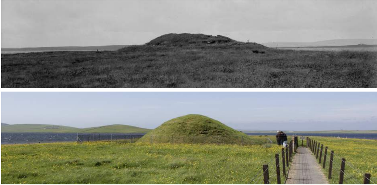
Figure 2.12: The mound of Unstan pre-installation of the HMMOW concrete dome, and now. Their forms were thought to be “inconspicuous” and “in harmony” with their monuments below. Top image courtesy of RCAHMS CANMORE archive, no date
