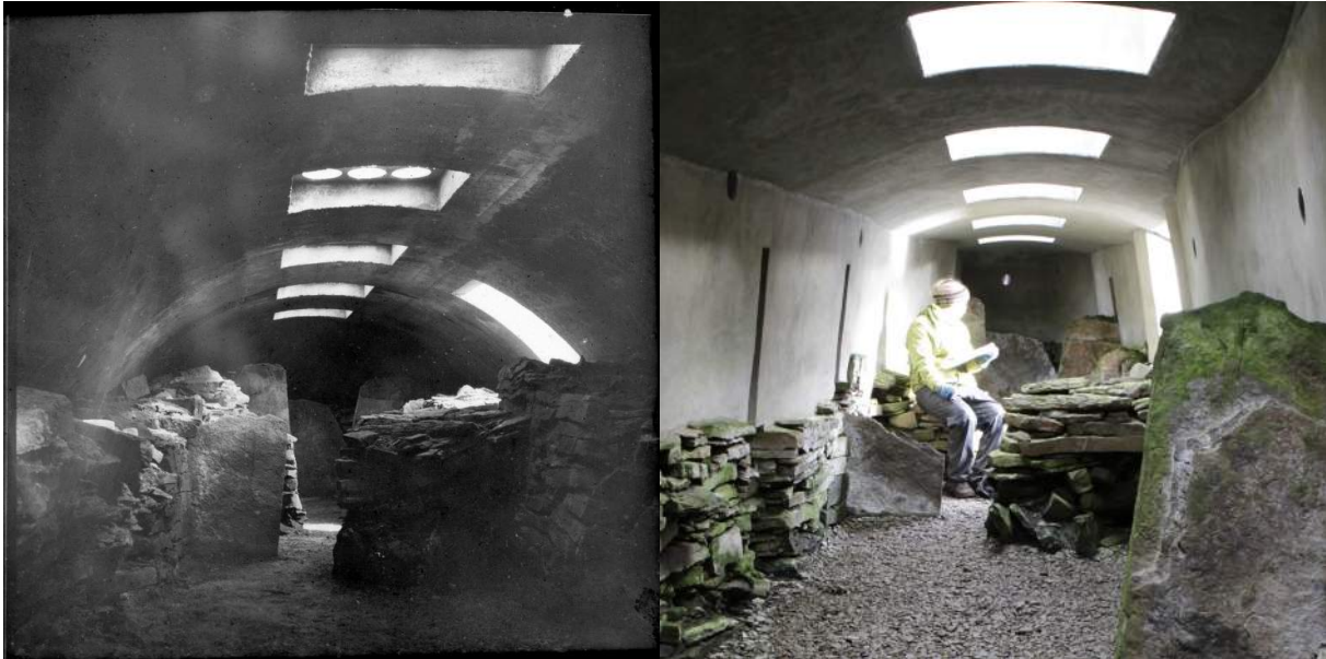
Figure 5.5a-c The dome at Blackhammer itself appears to have undergone modification, Image on Left shows the reinforced concrete dome as it was initially installed with a barrel-vaulted profile and the impression of the shuttering still visible. Image courtesy of RCAHMS CANMORE archive, No date. In contrast, the image on the right shows the current configuration of the roof having undergone substantial alterations, now with a smoother surface and far steeper sides which project deeper over the wallheads below
