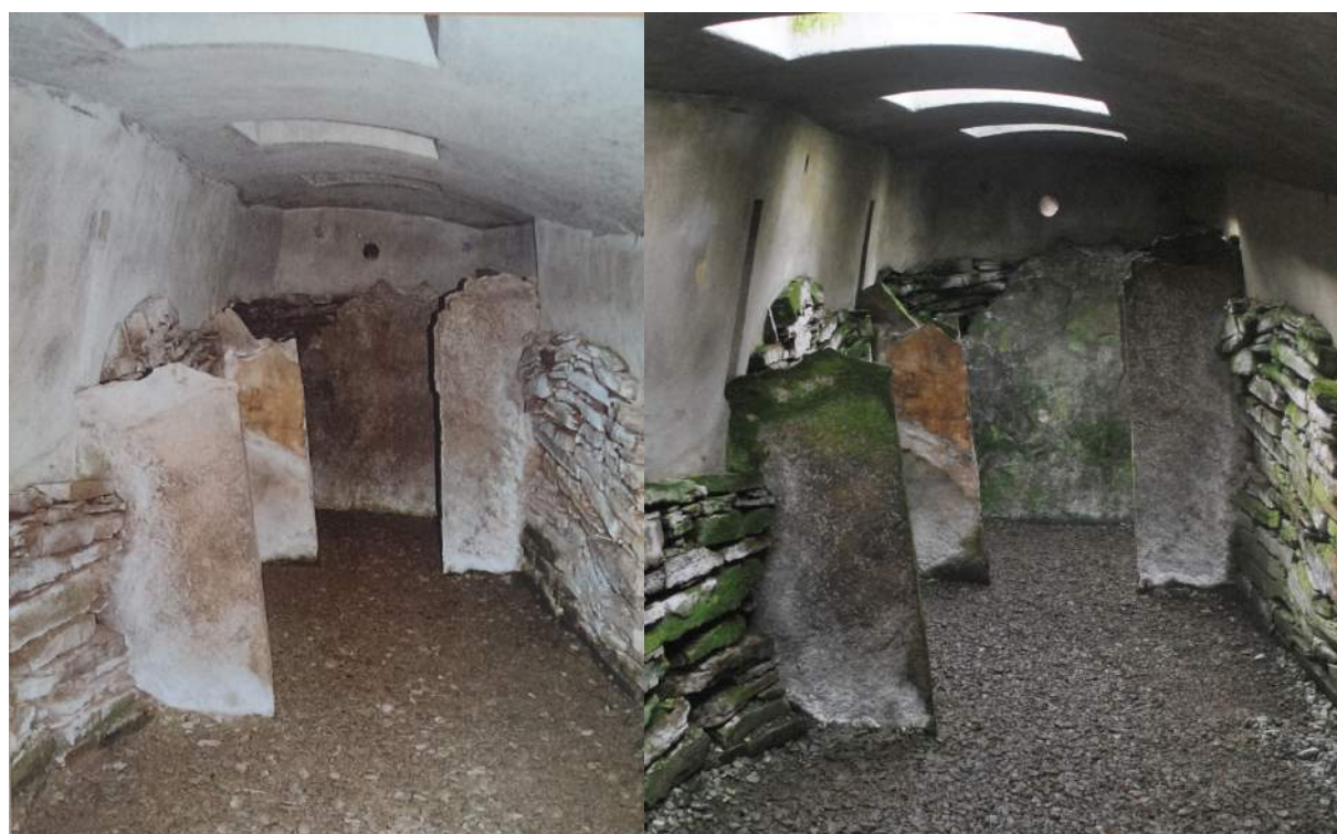
Figure 5.4a-b Above: Comparison of condition of stonework in Blackhammer between 1994 and now, revealed few changes beyond increased algal growth Left Image courtesy of RCAHMS photographic archive, 1994
