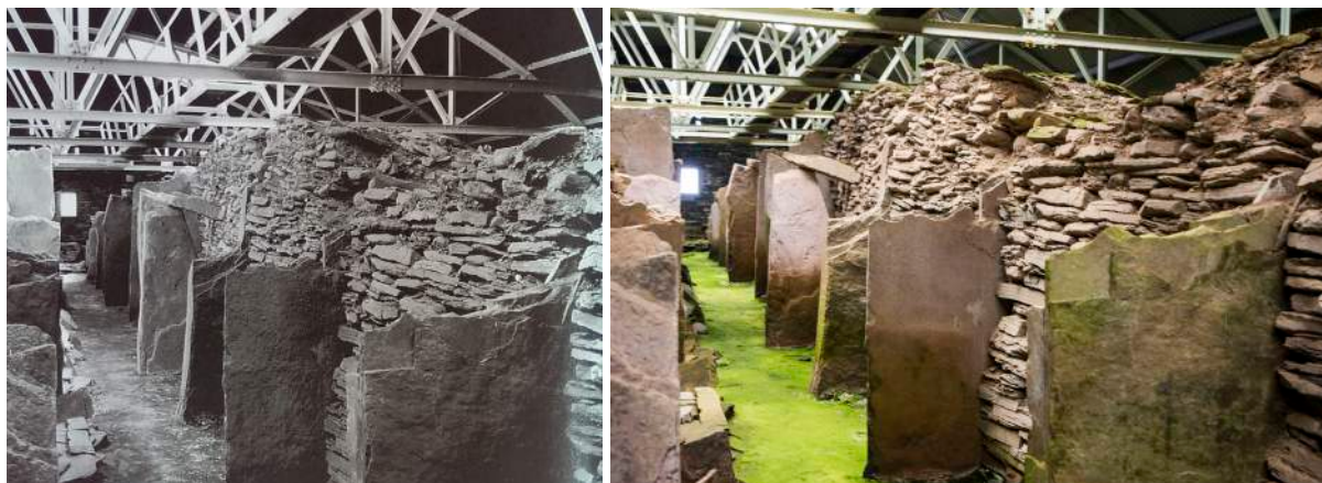
Figure 5.3a-b Above: Comparison of condition of stonework in Midhowe between 1956 and now, revealed few changes, Left Image courtesy of RCAHMS photographic archive, 1956
