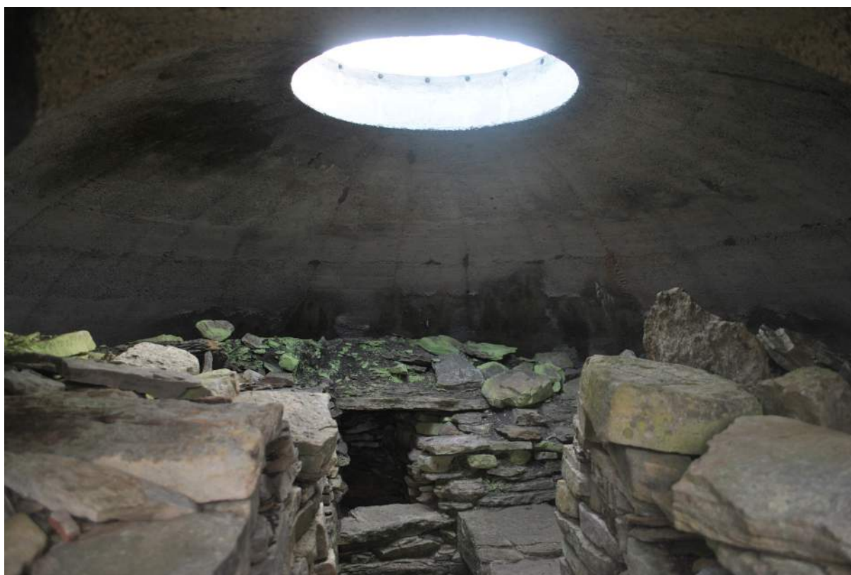
Figure 2.10: The upper storey of Taversoe Tuick was capped by a reinforced concrete dome with a circular skylight in 1937
