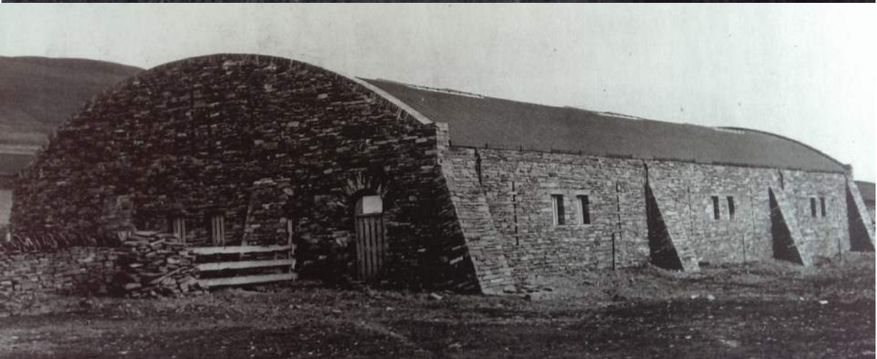
Figure 2.9a-e: This and previous page: Images of Midhowe cover house under construction, Undated but likely between 1935-1936
