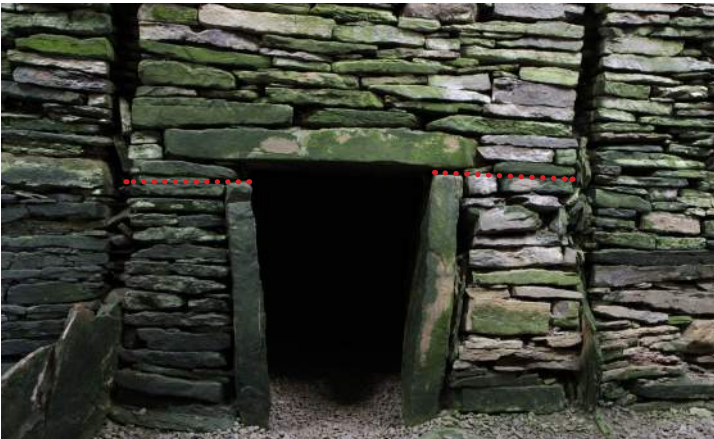
Figure 4.3a & b : Before the “small mural cell was made good”, and condition now: red line shows line of rebuild, Top Image Courtesy of RCAHMS photographic archive, No Date
