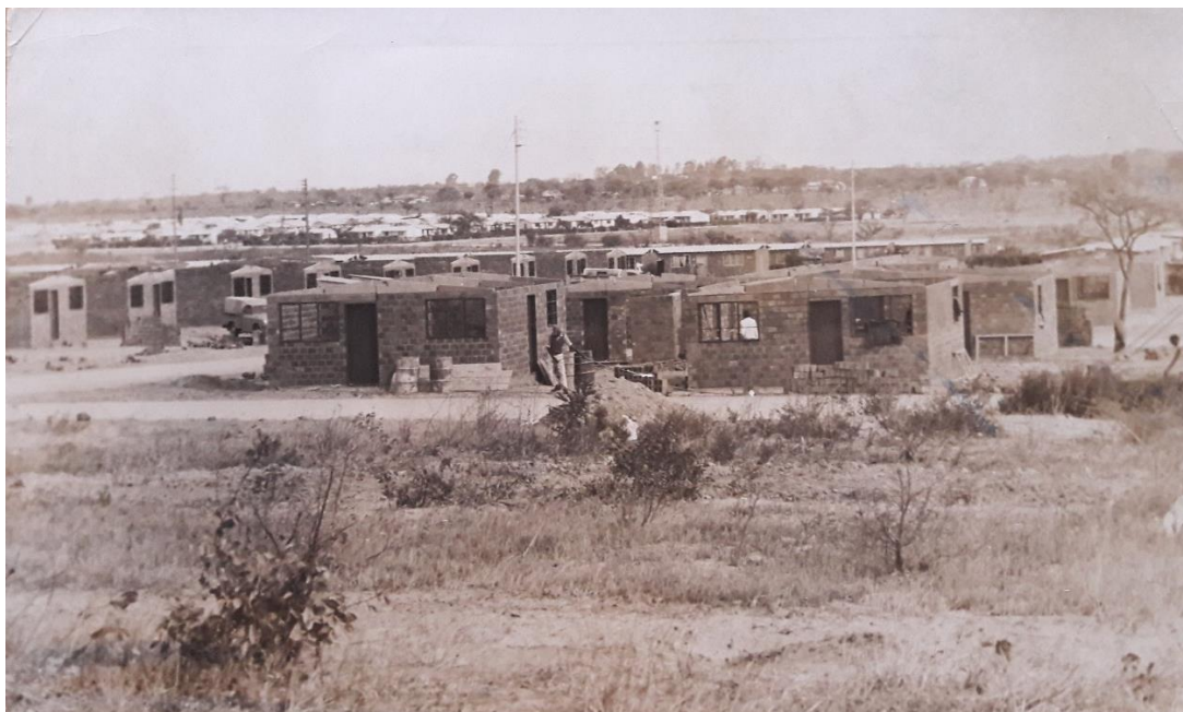
Figure 20: Magwegwe houses under construction. [Source: Chronicle, 10 Sept., 1968.]
