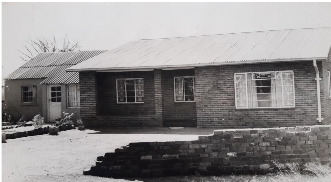
Figure 25: Rebuilt house in Barbour Fields, 1976 [Source: Chronicle, Chronicle, 23 Aug, 1976]
