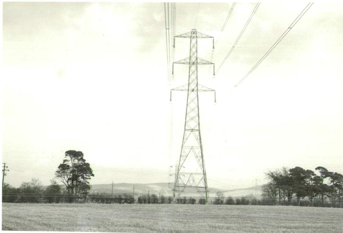
FIG. 31. 60 YD. - WIDE GAP IN A SHELTERBELT FOR ELECTRICITY TRANSMISSION TOWER & DISTRIBUTION LINE POLE
