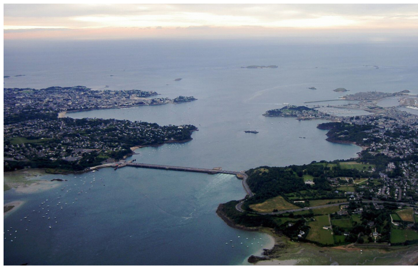
Figure 3.8: La Rance tidal barrage
