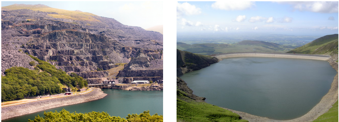
(a) Low reservoir and intake/outlet (Photo by Denis Egan)
