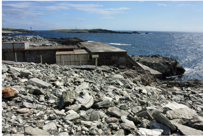
Figure 3.5: The Limpet oscillating water column (Photo by Peter Church)
