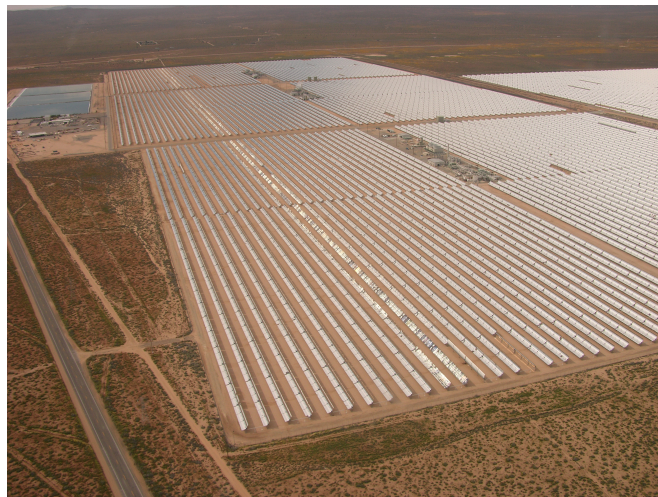
Figure 3.14: Solar Energy Generating Systems' concentrating solar troughs in the Mojave Desert, California (Photo by Alan Radecki)
