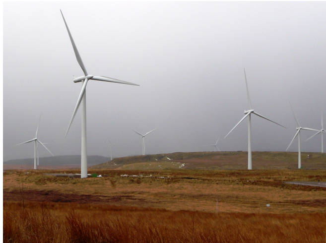
Figure 3.3: Whitelee wind farm
