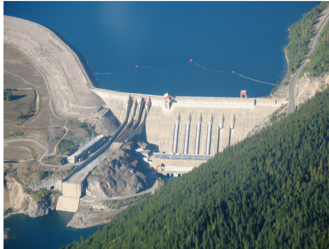
Figure 3.11: Revelstoke hydroelectric dam and generating station, BC, Canada (Photo by Kelownian Pilot at en.wikipedia)
