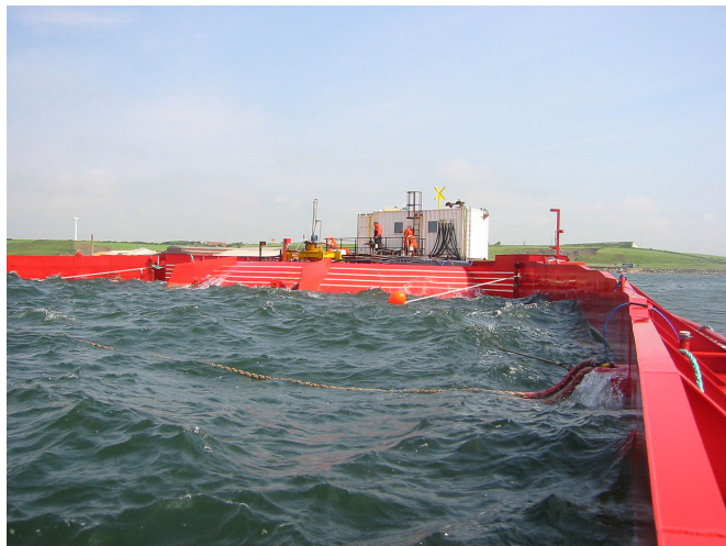
Figure 3.7: The Wave Dragon floating overtopping wave energy converter (Photo by Erik Friis-Madsen at en.wikipedia)
