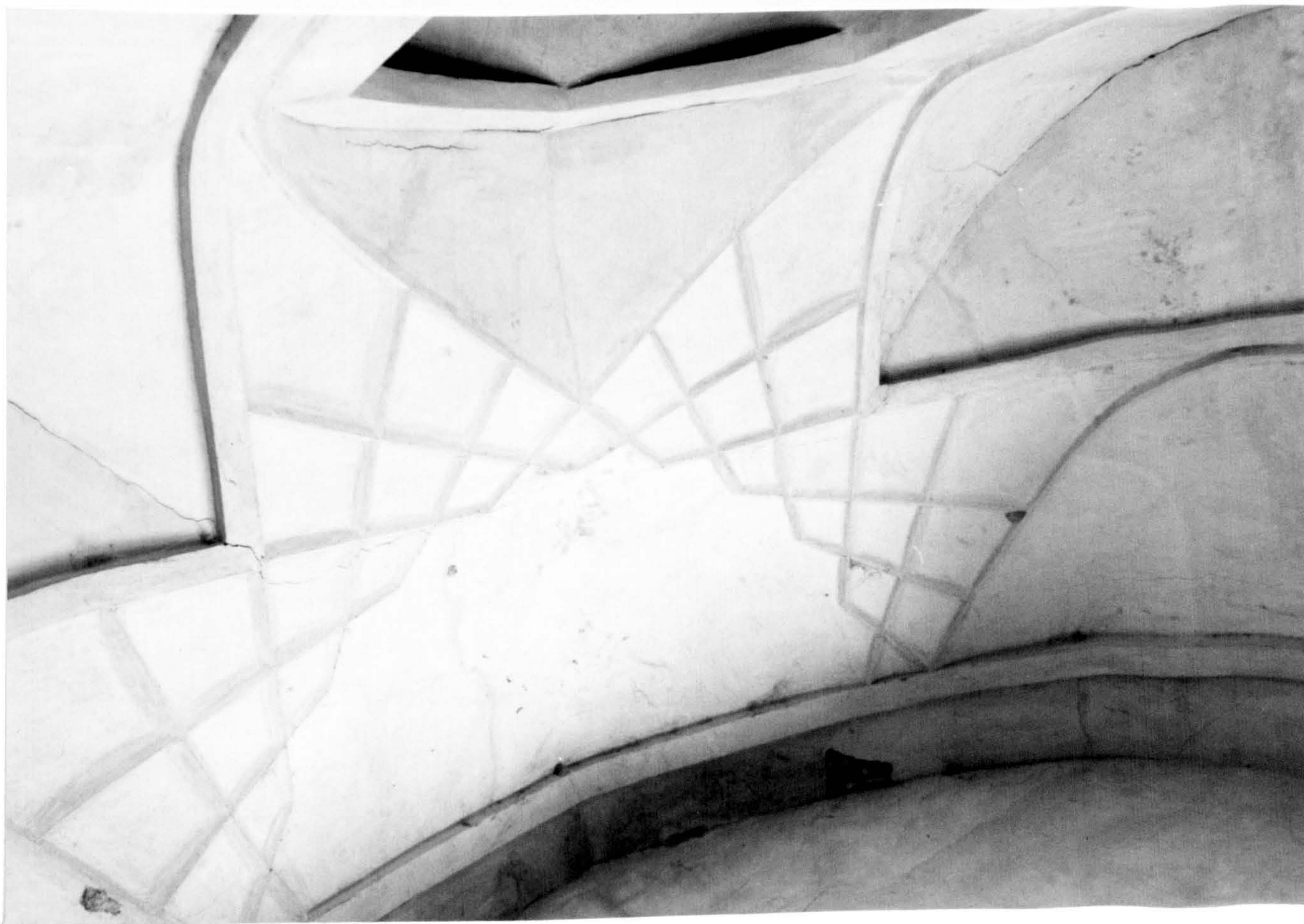
221) Gāzur Gāh: Zamīgār Khāna, vaulting above original S entrance
