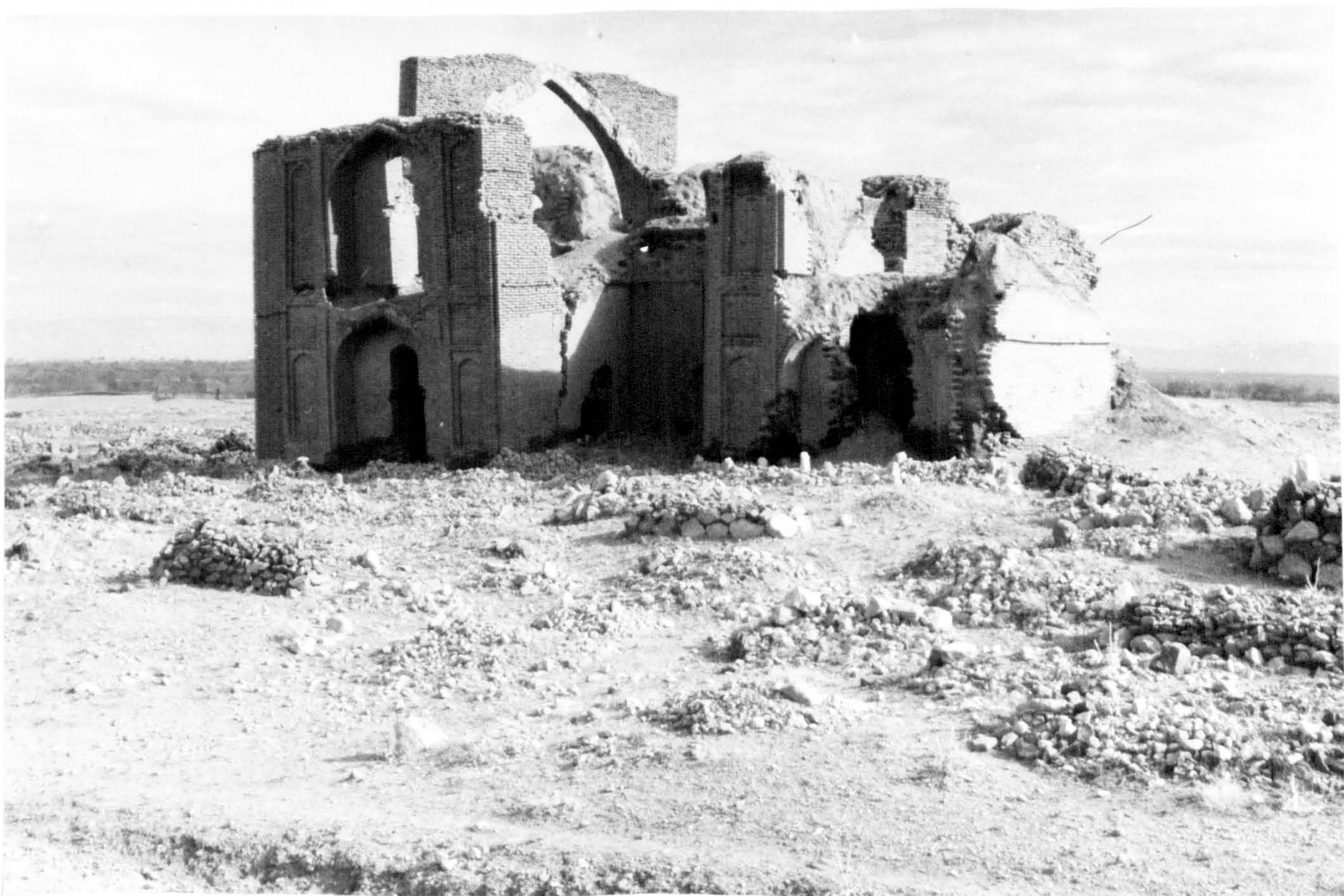
228) Ziyāratgāh: Khanqah of Mullā Kālān, exterior, general view, from SW
