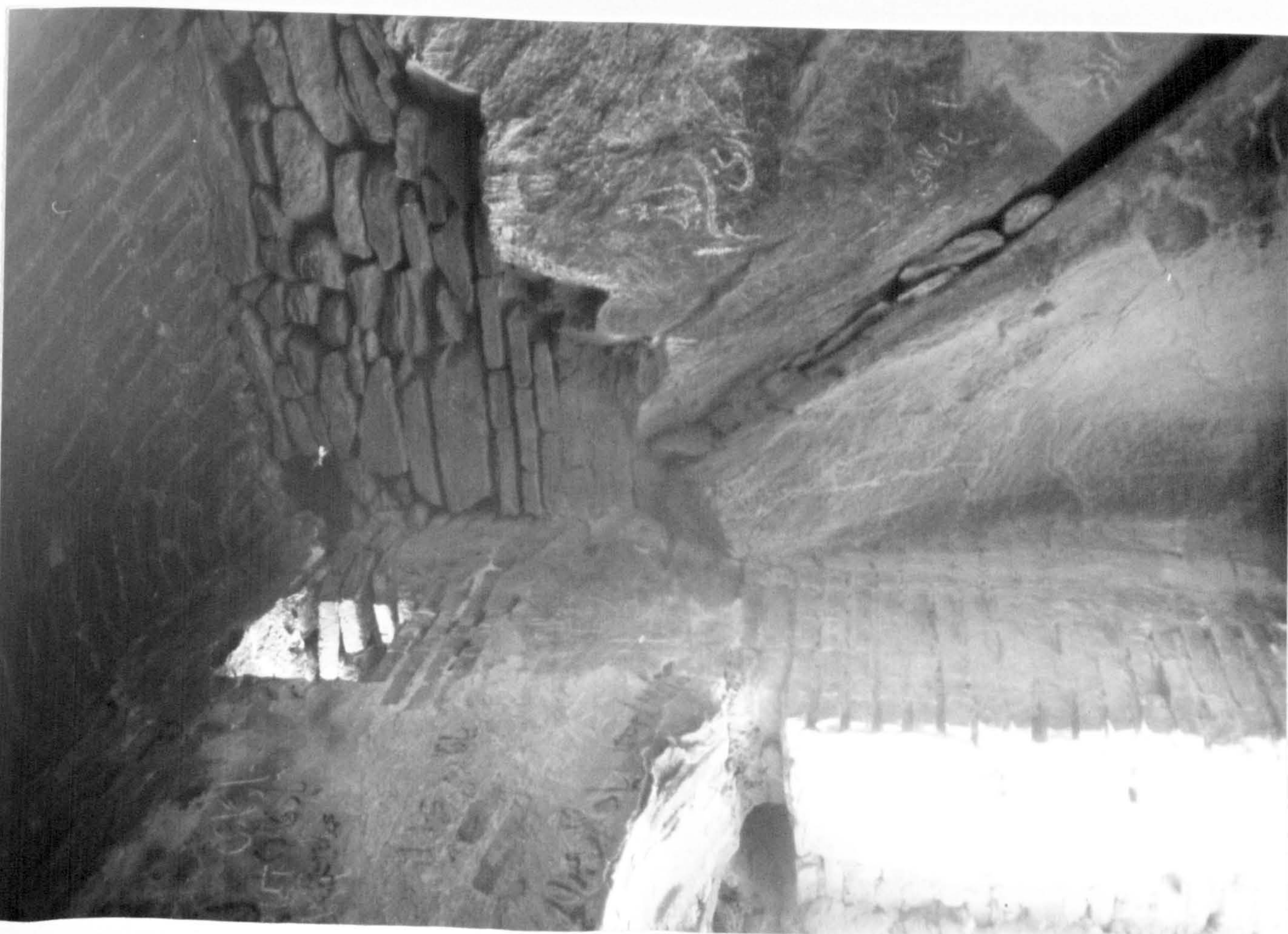
274) Herat: Ghār-i Darvīshān, interior, showing squinch vault
