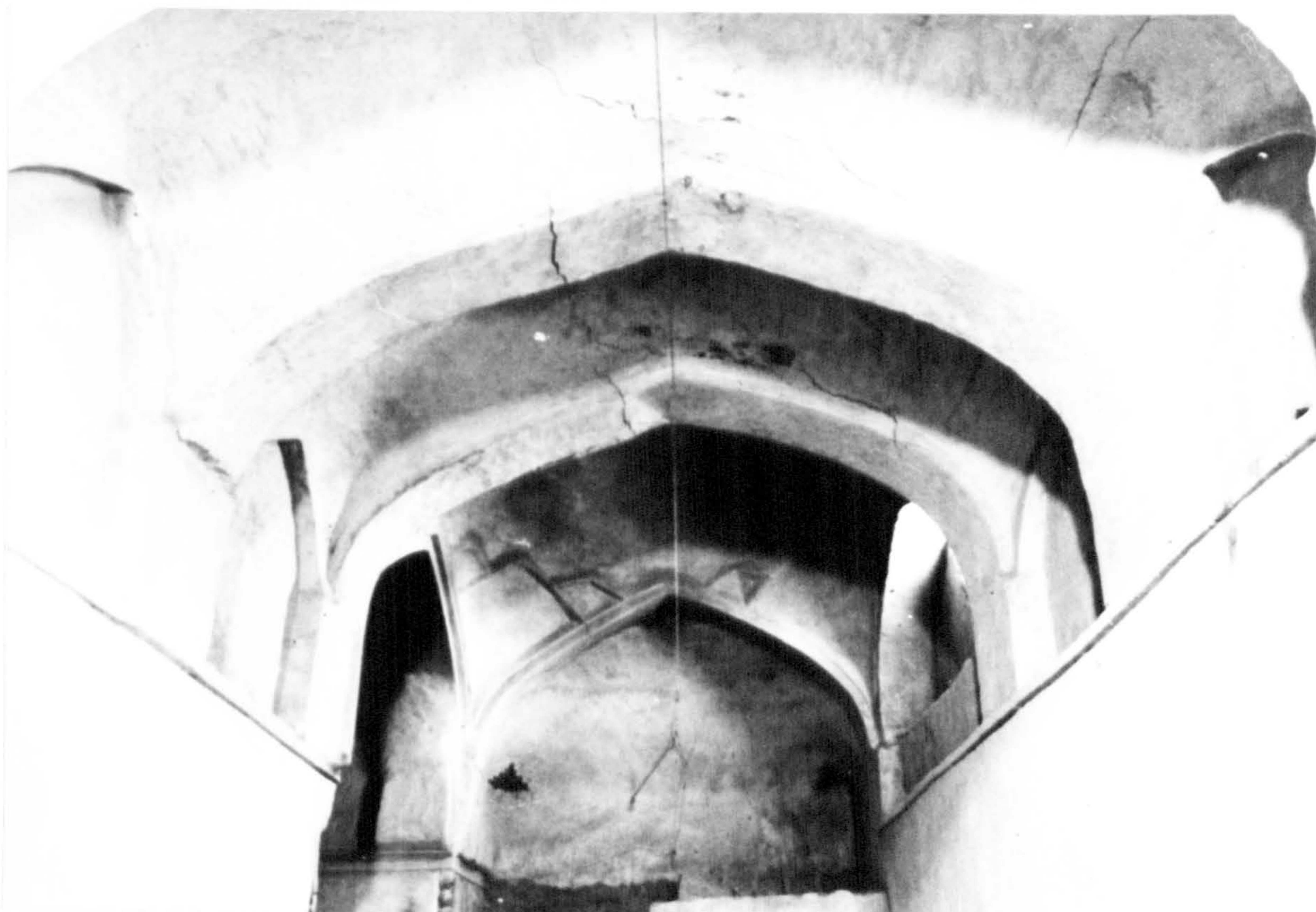
145) Khvāf: Masjid-i Jami c , transverse vaulting in hall beside aivan (after Golombek)
