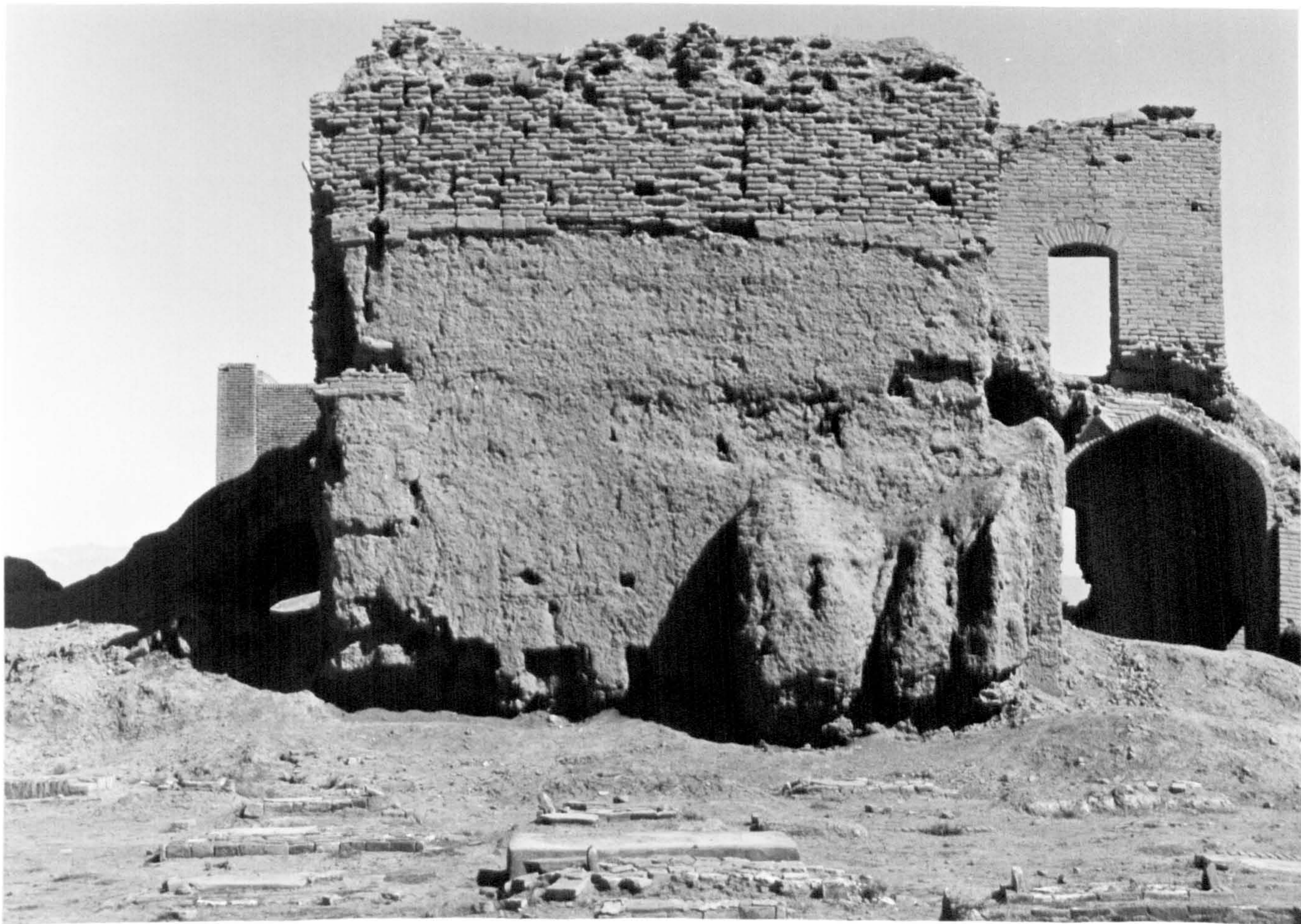
224) Turbat-i Jām: 'Īdgāh, rear facade
