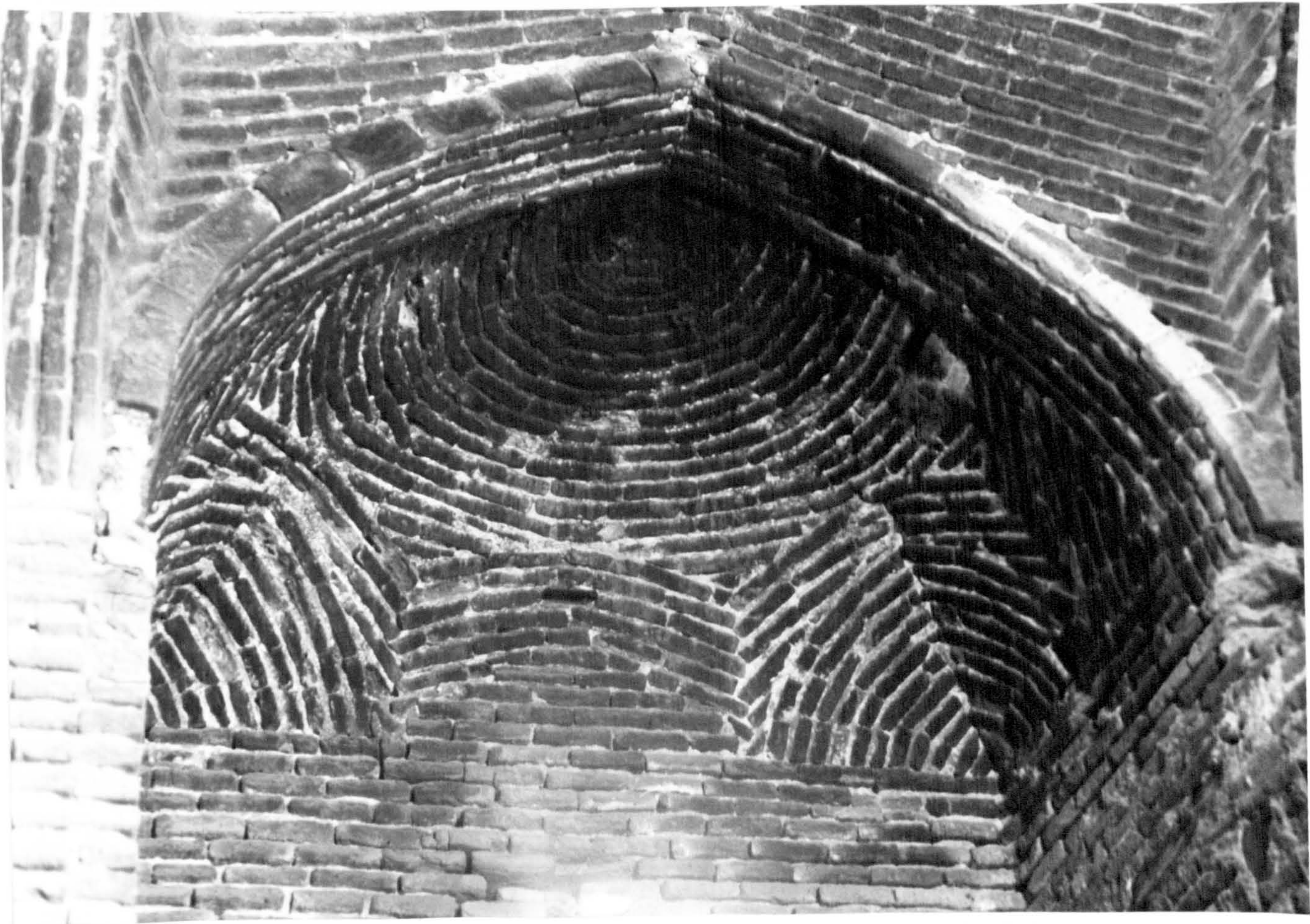
280) Kadkan: Mazar-i Nizām al-Mulk, vaulting in niche in gallery of shabistān
