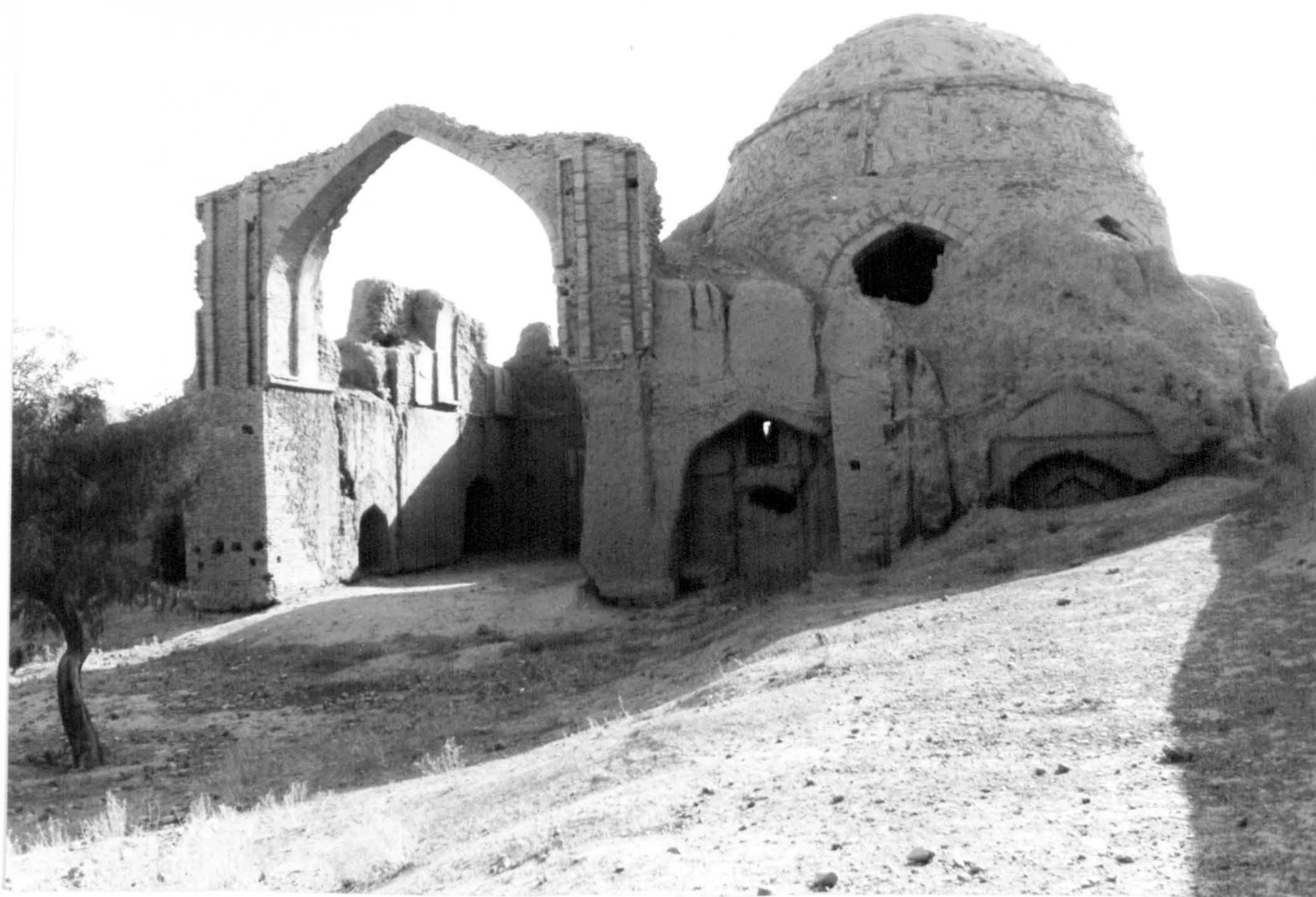
135) Rushkhvār: Masjid-i Jami C , aivan and dome chamber, from courtyard
