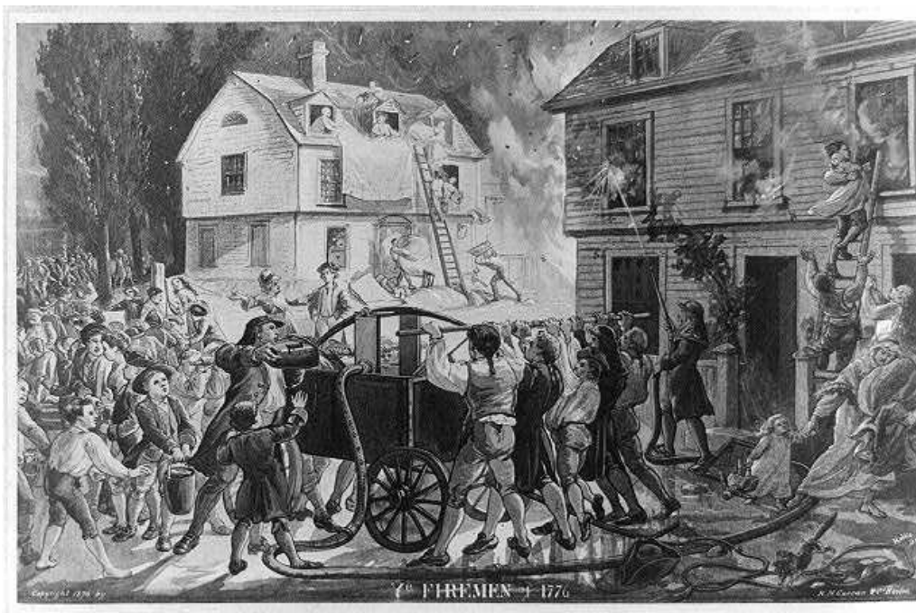
Figure 1.1. Depiction of 18 th Century fire-fighting in tenement buildings typical of the time [12].
