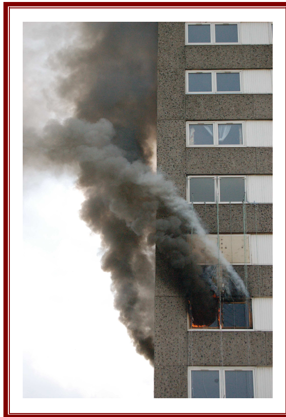
- The External Plume during Dalmarnock Fire Test One -
