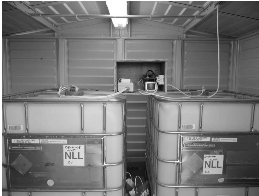
Fig 12. Tanks installed in shed
