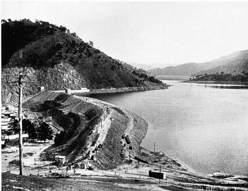
FIG. 1. Eildon Reservoir. General view of bank during remedial work 1929-30. From lower slopes of Mt. Pinniger
