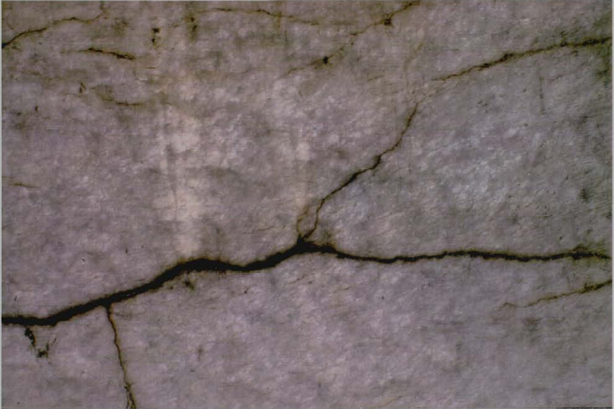
2. Detail of alabaster window, Sana'a'.
