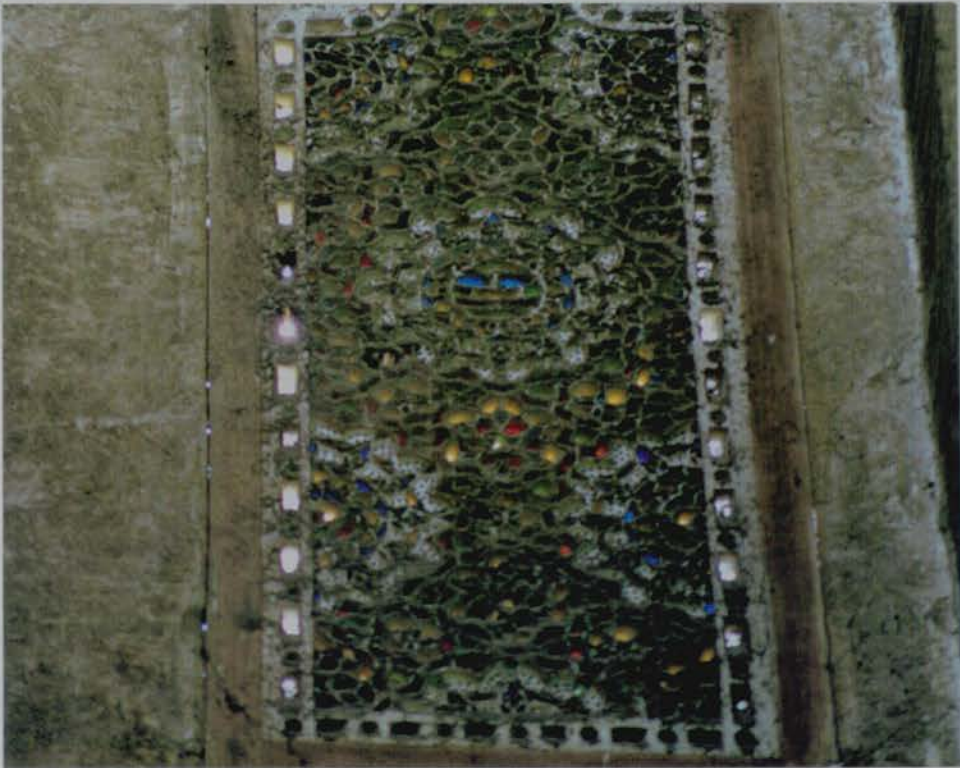
80. Detail of a qamariyya in the north-western wall of the mausoleum, madrasa of Īnāl al-Yūsufī .
