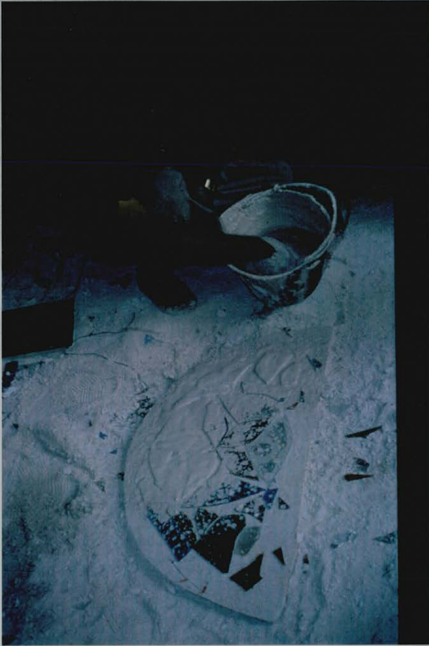
148. Making an 'aqd - laying the second layer of plaster (photograph M. Mutahir).
