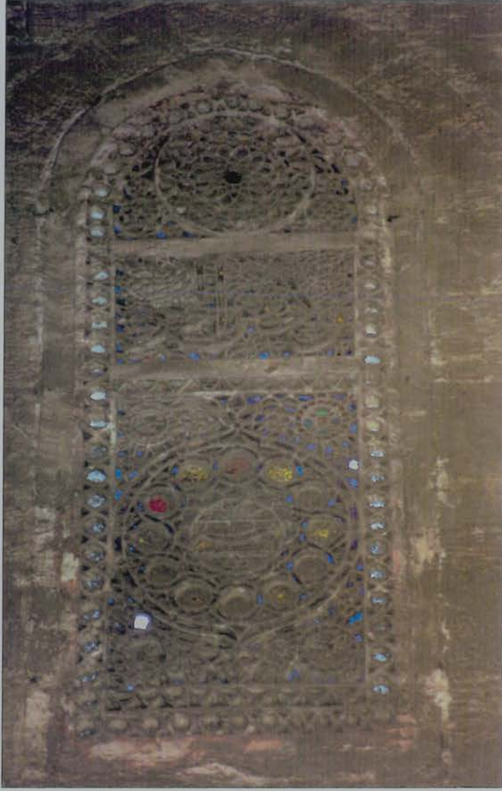
82. Qamariyya in the the north-eastern iwan , Madrasa of Jamāl al-Dīn Yūsuf al-Ustādār, Cairo.
