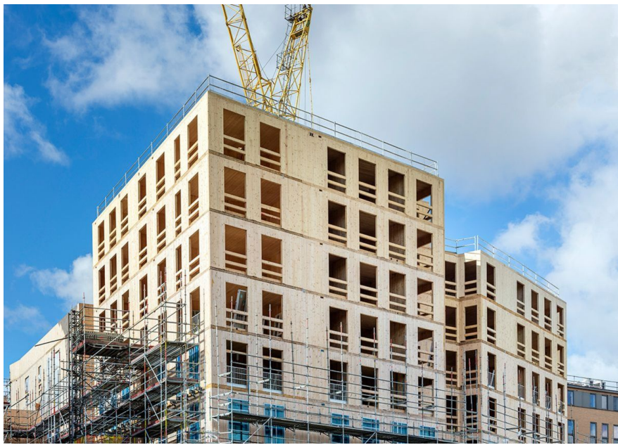
Figure 2.2. Construction site of a mass timber building in London, UK [50].
