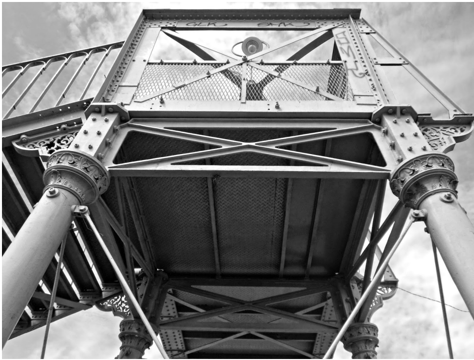
Figure 3–144. Pergamino footbridge made by Handyside. Source: Ibid.
