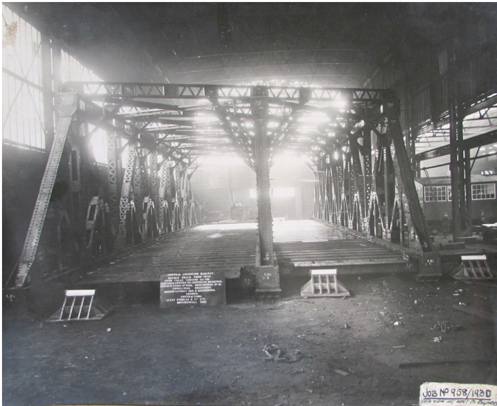
Figure 3–152. Railway Bridge for Calle Cervino. Alex Findlay and Co. Source: Alex Findlay Company records, NLA
