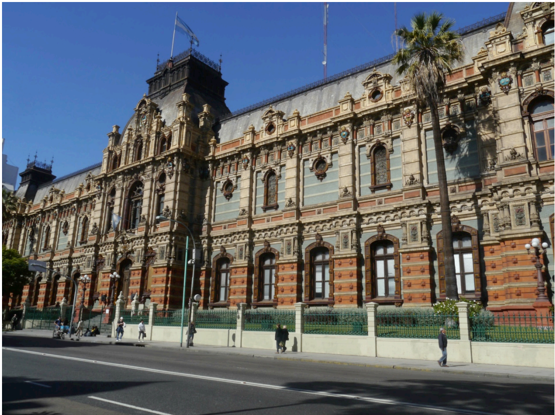
Figure 3–177. Façade of the Palace of Running Waters. Source: Photo Lucia Juarez
