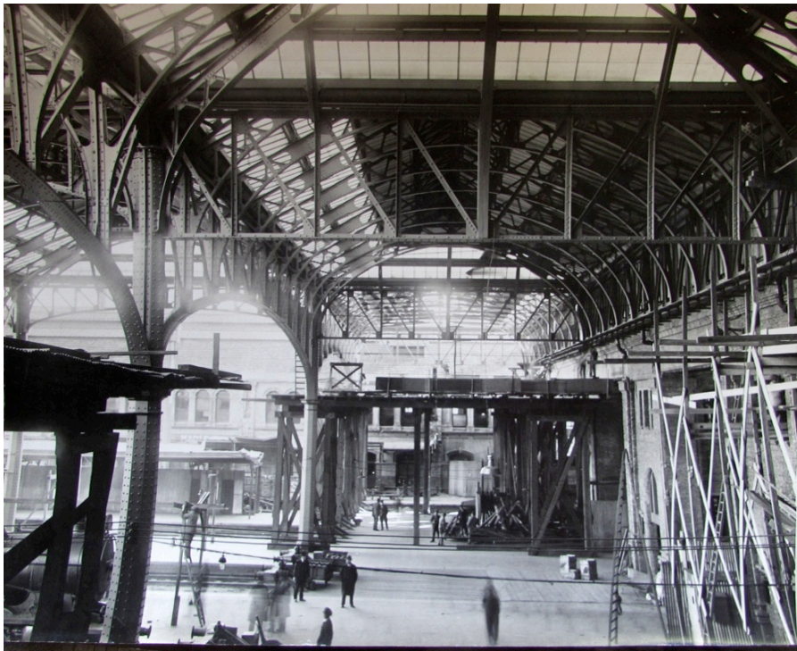
Figure 3–31. Iron train shed being re-assembled on site in Plaza Constitucion IV. Source: Alex Findlay Company records. NLA
