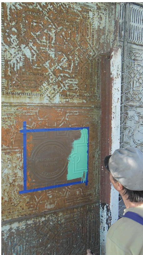
Figure 3–106. Macfarlane cast-iron urinals at Tornquist Station (FCS), panel detail. Source: Pablo Marzilio
