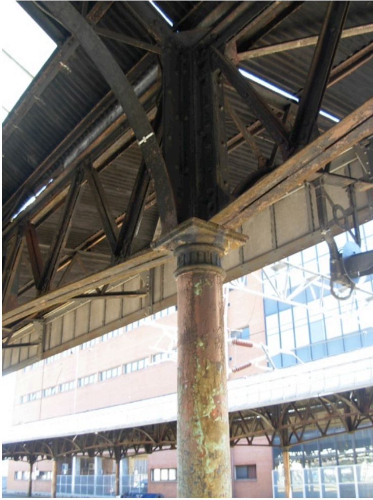
Figure 3–29. External platforms showing combination of types of iron. Source: Photo Lucia Juarez
