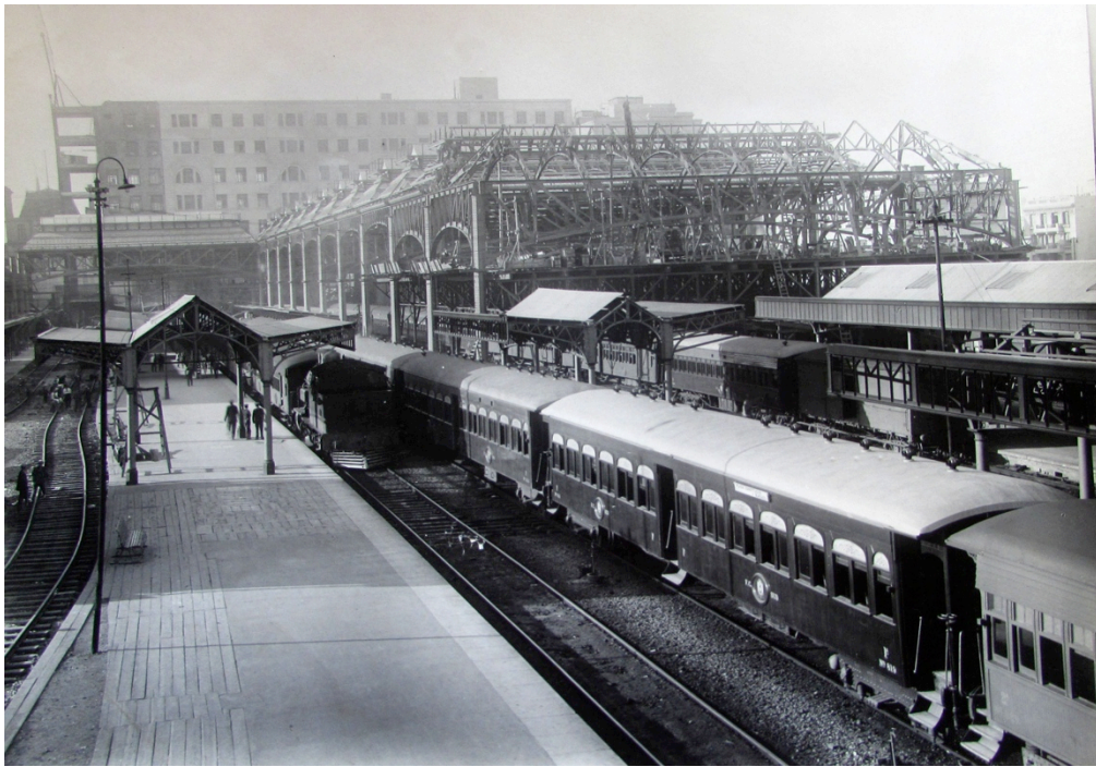
Figure 3–27. Plaza Constitucion IV under construction. Source: Alex Findlay Company Records, NLA
