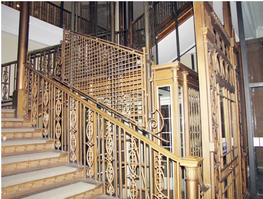
Figure 3-361. Carron stair and lift case. Source: Photo Monica Ferrari 2013
