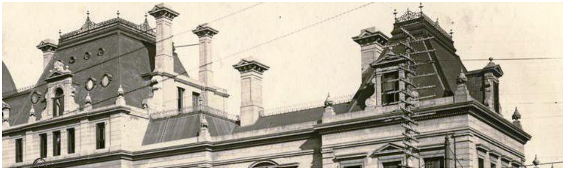
Figure 3–13. Roof railings Plaza Constitucion III. Source: AGN
