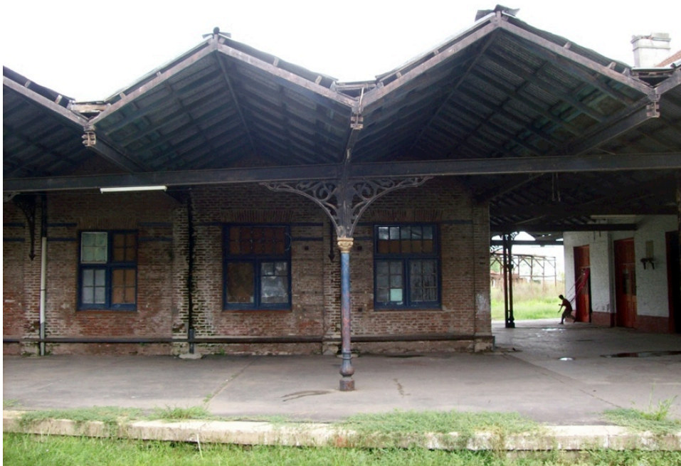
Figure 3–99. Lobos Junction station. Cast-iron brackets and columns. Source: Photo Luis Benitez
