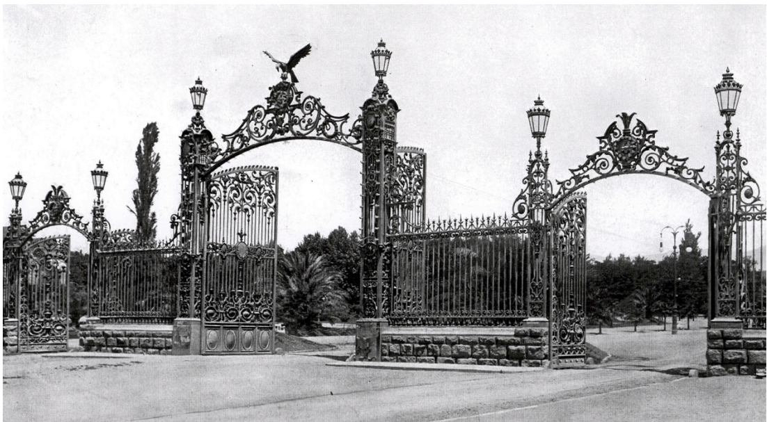
Figure 3–300. Walter Macfarlane gate in San Martin Park just after it was installed. Source: Ironwork Foundation
