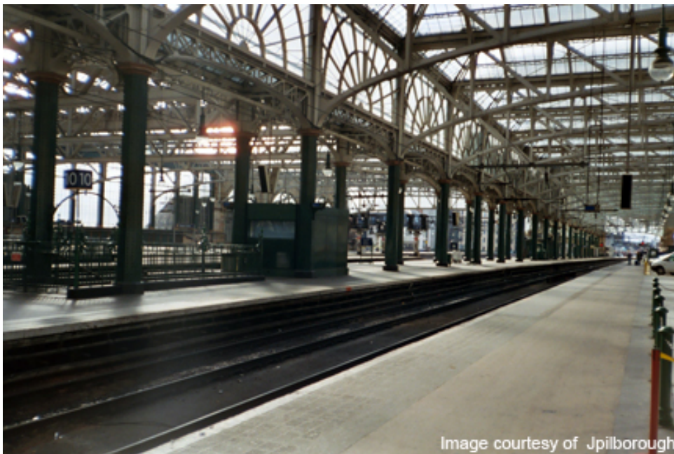
Figure 3–38. Train shed Glasgow Central Station. Source: ‘Glasgow Central Station, United Kingdom’, http://www.railway-technology.com/projects/glasgowcentralstatio/glasgowcentralstatio3.html (accessed September 12, 2017).
