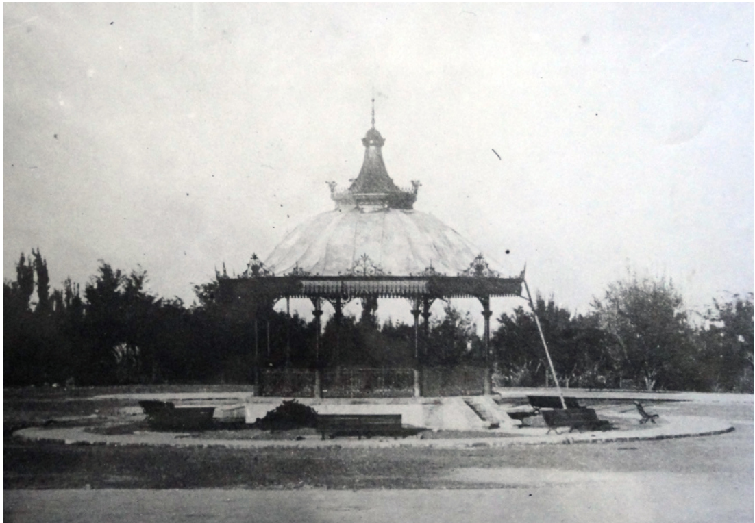
Figure 3–293. J. & A. Law bandstand after installation, and beginnings of work around the rotonda. Source: Ibid, p. 54
