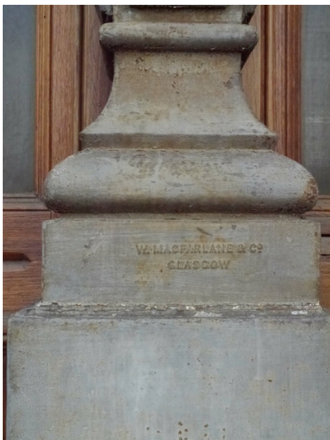
Figure 3–195. Cast-iron caryatides base showing nameplate. Source: Photo Lucia Juarez
