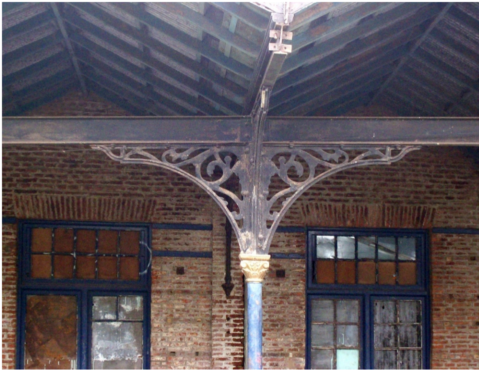
Figure 3–98. Lobos Junction station. Detail of cast-iron brackets. Source: Photo Luis Benitez
