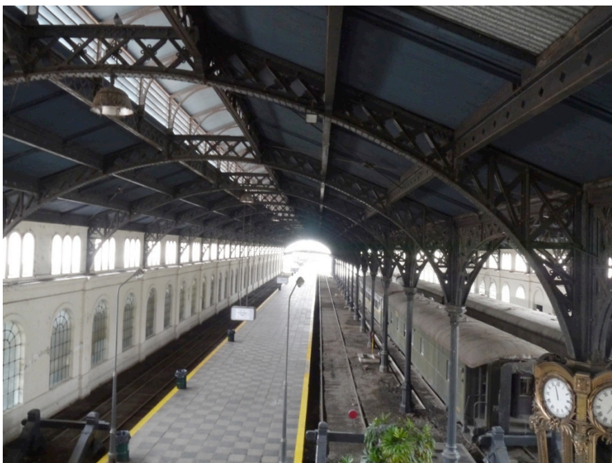
Figure 3–51. Mitre Station. Train shed structure. Source: Photo Lucia Juarez
