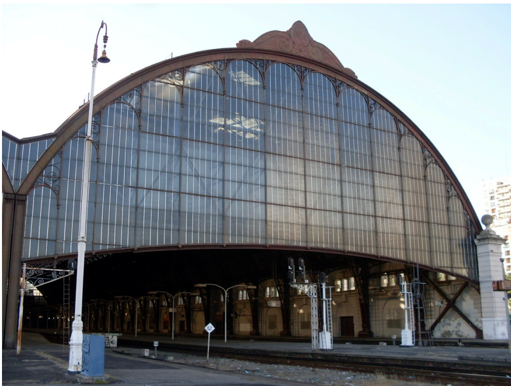
Figure 3–40. Retiro Station FFCA, rear façade. Macfarlane lamp. Source: Photo Pablo Marzilio
