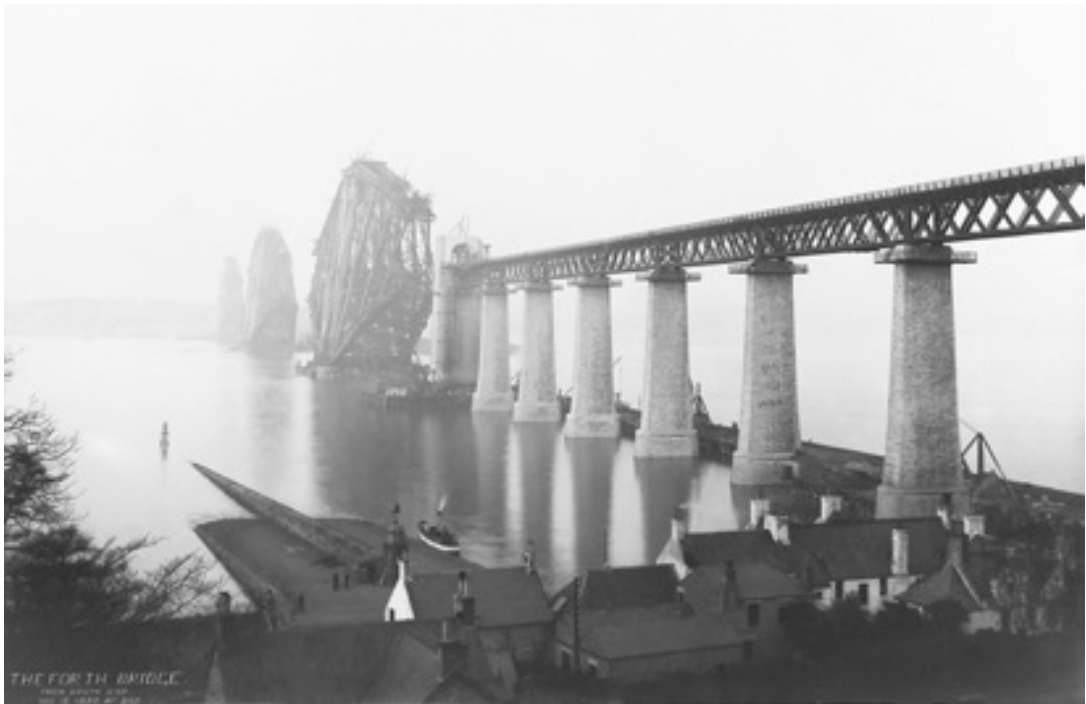
Figure 1–8. Forth Bridge. View from south side of south approach viaduct and progress on piers, 18 Dec 1888. Source: NRS
