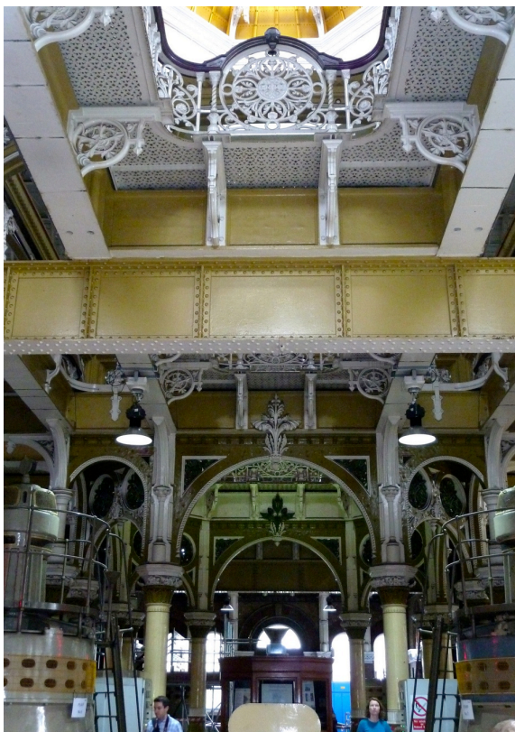
Figure 3–205. Interior of Abbey Mill Pumping Station. Source: Photo Adrian Dunn. https://www.flickr.com/photos/adriandunn/15288805636/in/photostream/
