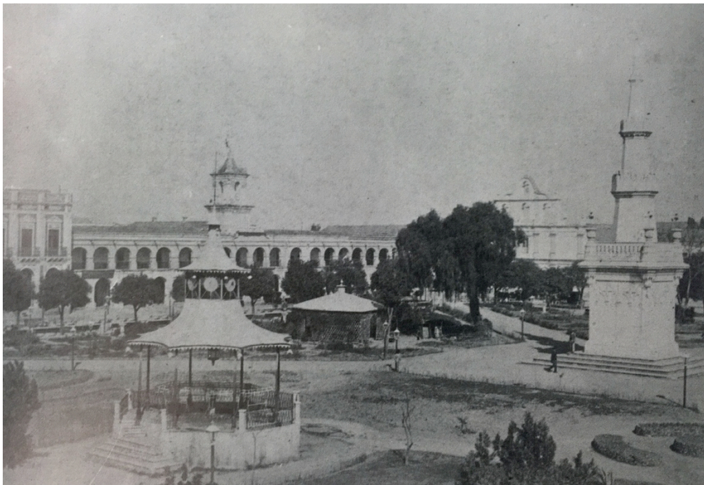
Figure 3–218. Bandstand in Salta. Source: AGN
