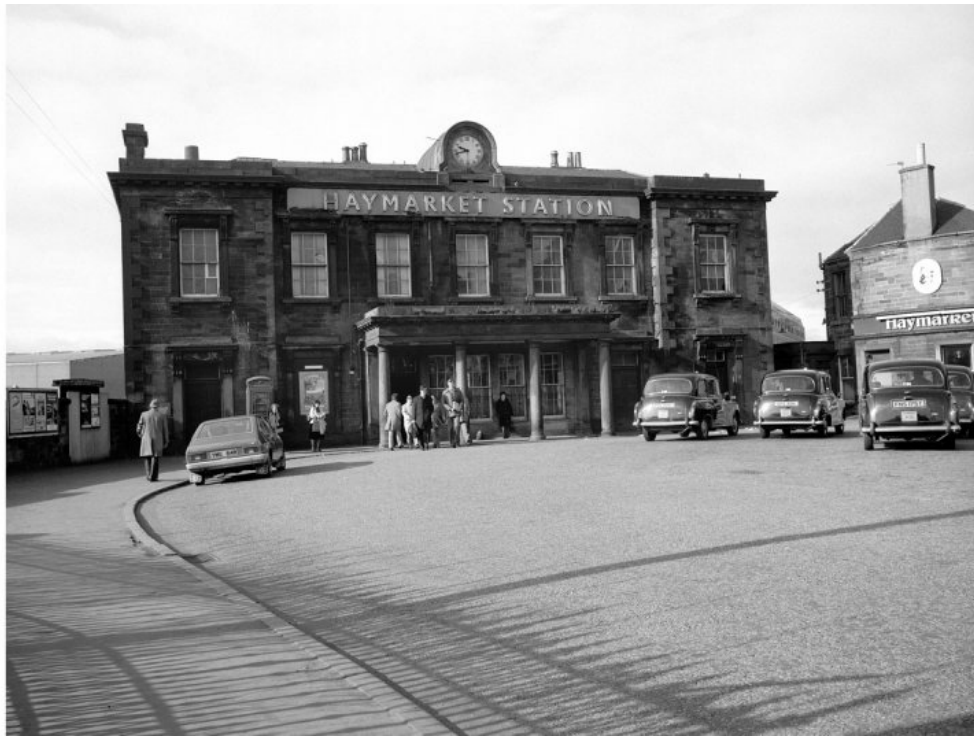
Figure 3–54. Haymarket Station in Edinburgh. Source: RCAHMS
