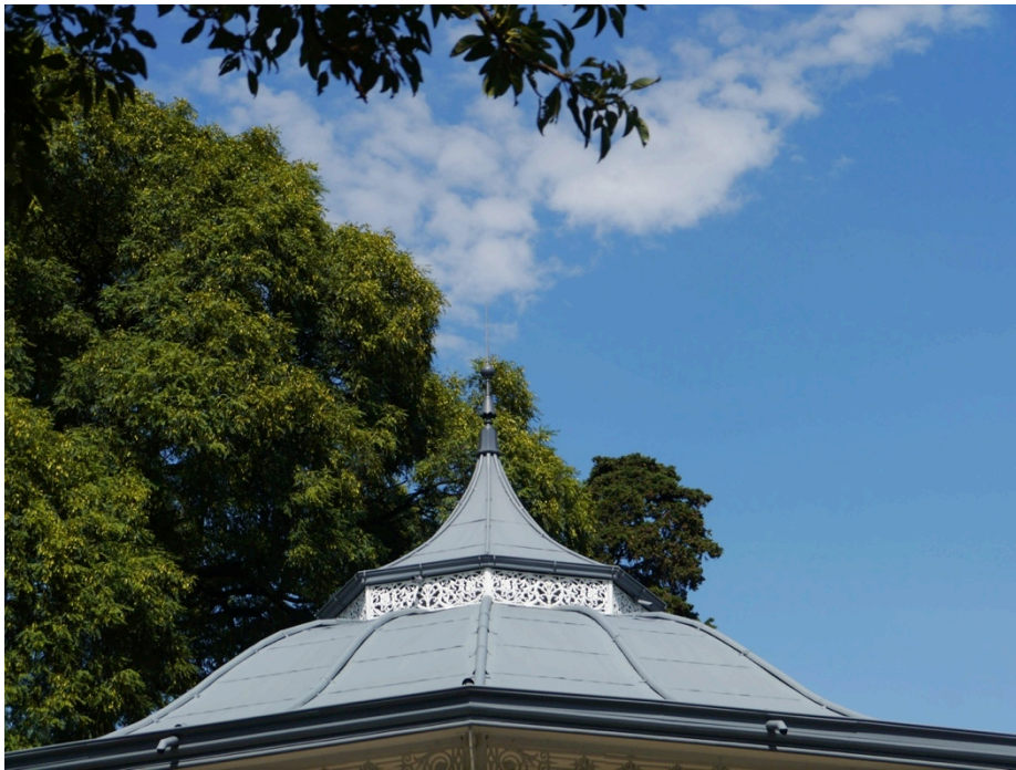
Figure 3–282. Roof detail, Walter Macfarlane bandstand in Buenos Aires Zoo. Source: Photo Lucia Juarez
