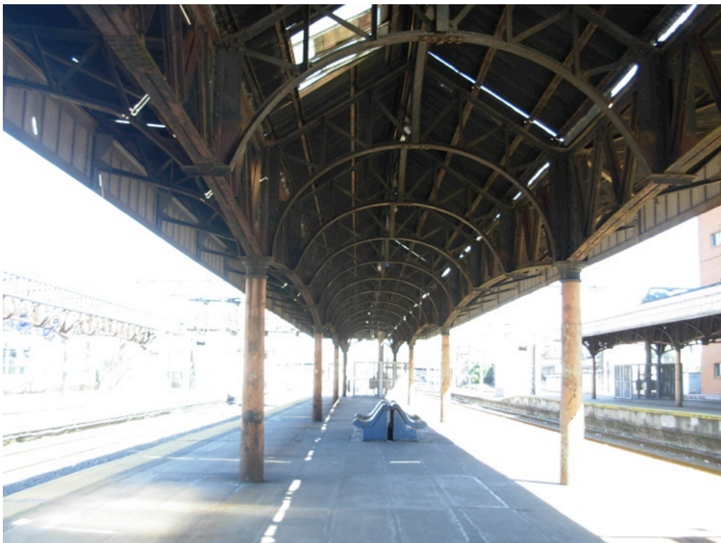
Figure 3–28. External platforms. Source: Photo Lucia Juarez
