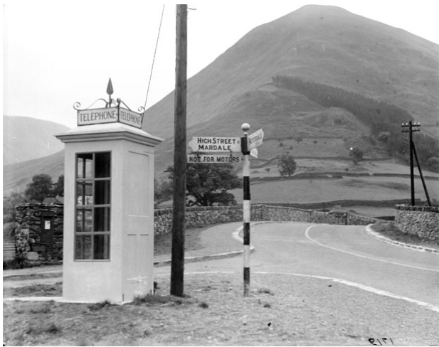
Figure 3–319. K1 designed in 1921 by the Post Office. Source: BT Archives, H. Bouckley, ‘The stamp-selling Vermilion Giant, Gilbert Scott’s classic K6 and more: The history of the red call box’, http://home.bt.com/tech-gadgets/history-of-the-red-telephone-box-kiosk-11364141615834 (accessed March 15, 2017).
