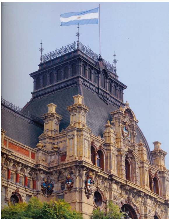
Figure 3-179. Cast-iron blind arcades and railings on roof. Source: Ibid., p. 189
