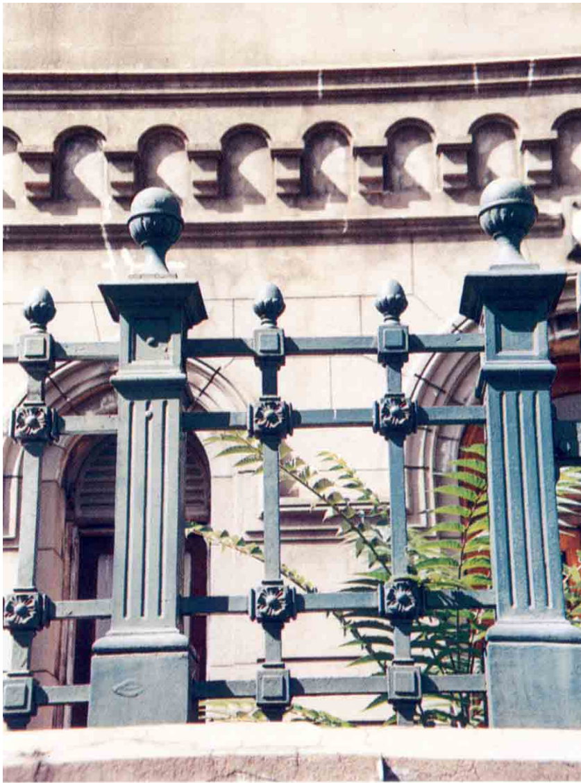
Figure 3–201. Macfarlane gate at Caballito Reservoir. Source: Jorge Tartarini
