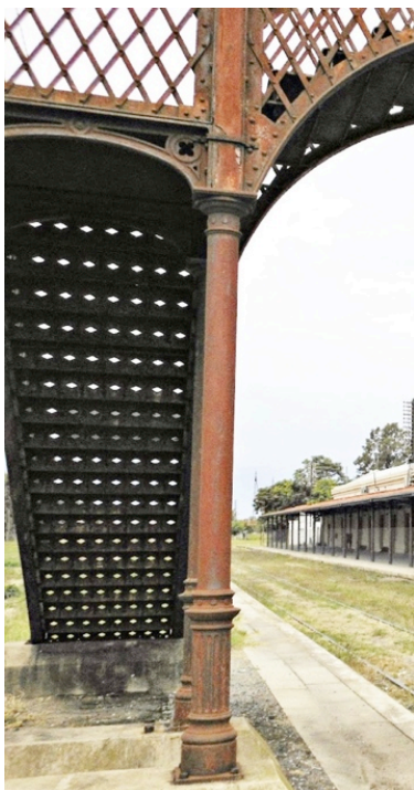
Figure 3–141. Detail of cast-iron column Pergamino footbridge made by Arrol Brothers. Source: Ibid.
