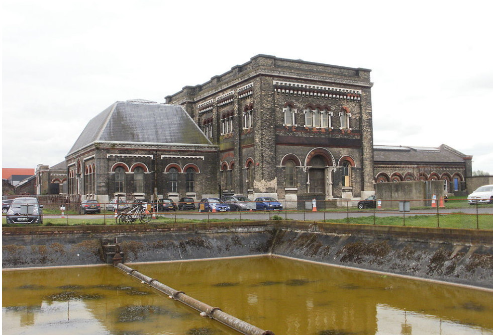
Figure 3–202. Exterior of Crossness Pumping Station. Source: Ethan Doyle White, CC BY-SA 3.0, https://commons.wikimedia.org/w/index.php?curid=44443562
