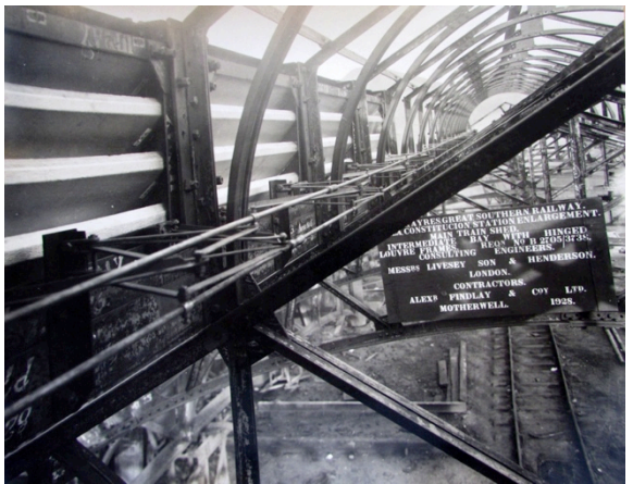
Figure 3–30. Train shed sections being assembled in the Alexander Findlay and Co. workshop before shipment to Argentina. Source: Alex Findlay Company records, NLA
