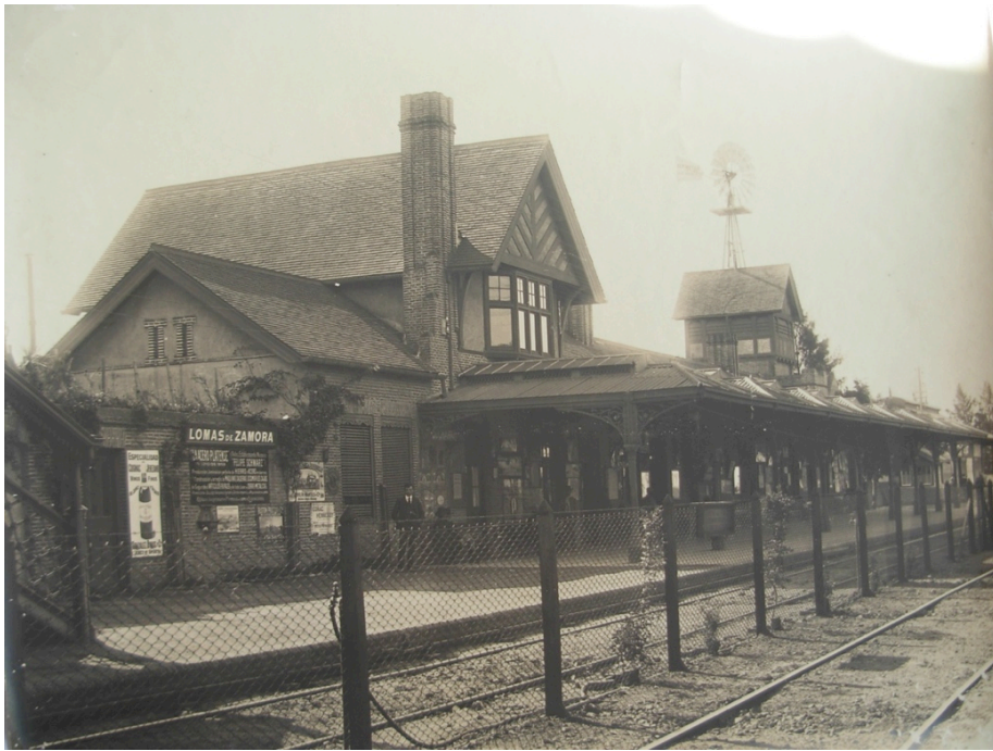
Figure 3–59. Lomas de Zamora Station (FCS). Source: FMF
