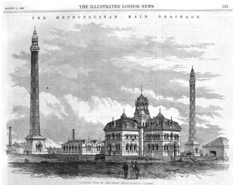
Figure 3–204. Abbey Mills Pumping Station in 1868. Source: The Illustrated London News , taken from: P. Dobraszcyk, ‘Architecture, Ornament and Excrement: The Crossness and Abbey Mills pumping stations’, Journal of Architecture , vol. 12, no. 4 (2007)
