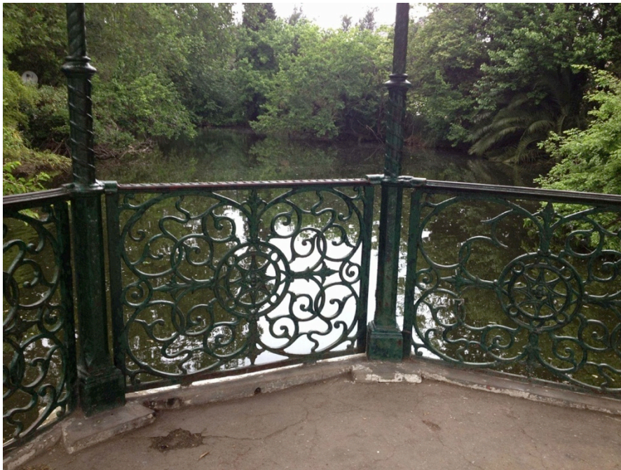
Figure 3–265. Railing detail of gazebo made by George Smith in 3 de Febrero Park. Source: Photo Lucia Juarez
