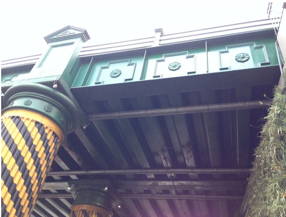
Figure 3–149. Handiside railway bridge. Detail of cast-iron columns. Source: Photo Lucia Juarez
