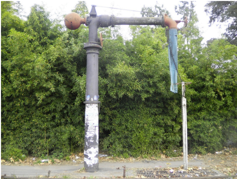
Figure 3–77. Water crane at Escobar Station made by Brandon Bridge Building. Source: Pablo Marzilio
