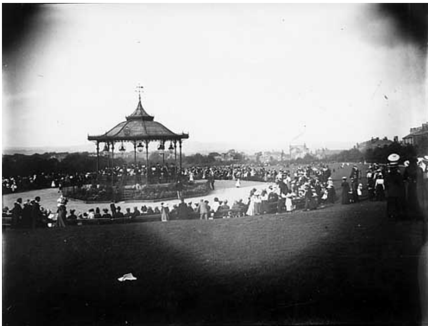
Figure 3–290. Walter Macfarlane bandstand no. 249 at Bramley Park, Leeds, England. Source: ‘Bramley Park’, http://www.leodis.net/display.aspx?resourceIdentifier=2003217_58524722&DISPLAY=FULL . (accessed August 13, 2017).
