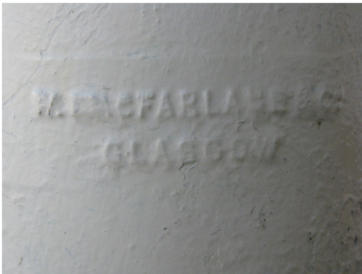
Figure 3–117. Alta Cordoba Station. Macfarlane stamp on cast-iron columns. Source: Monica Ferrari
