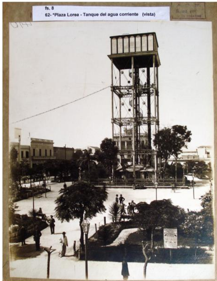
Figure 3–160. Plaza Lorea water tank. Source: AGN
