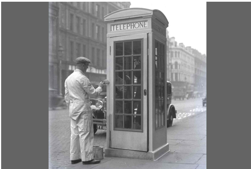
Figure 3–322. Painting a K3 telephone kiosk outside Belfast General Post Office, 1936. Source: Ibid.
