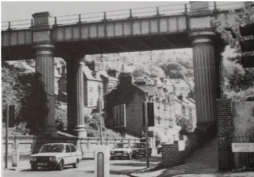
Figure 3–151. Queens Road railway bridge in Hastings, England. Source: Biddle and Nock, The Railway Heritage of Britain: 150 Years of Railway Architecture and Engineering , p. 196
