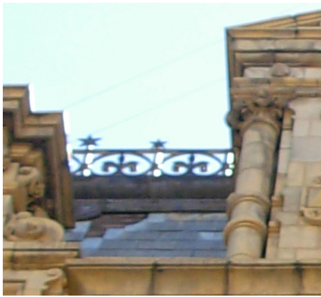
Figure 3–184. Example of a Macfarlane railing model no. 148. Source: Photo Lucia Juarez
