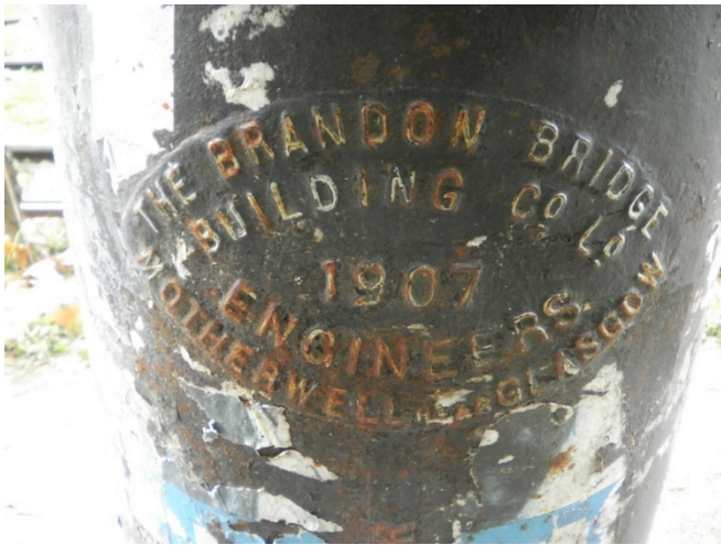
Figure 3–78. Nameplate on water crane. Escobar Station. Source: Pablo Marzilio
