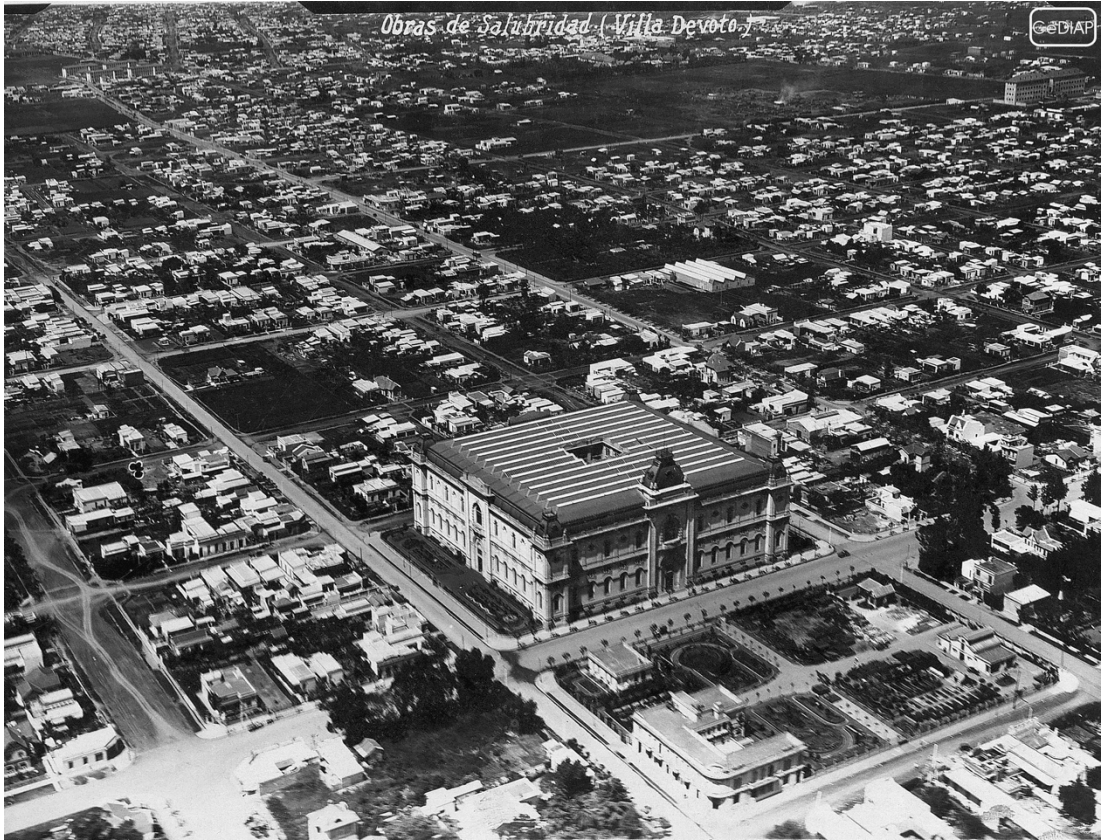
Figure 3–200. Aerial view of Devoto Great Reservoir. Source: Aysa
