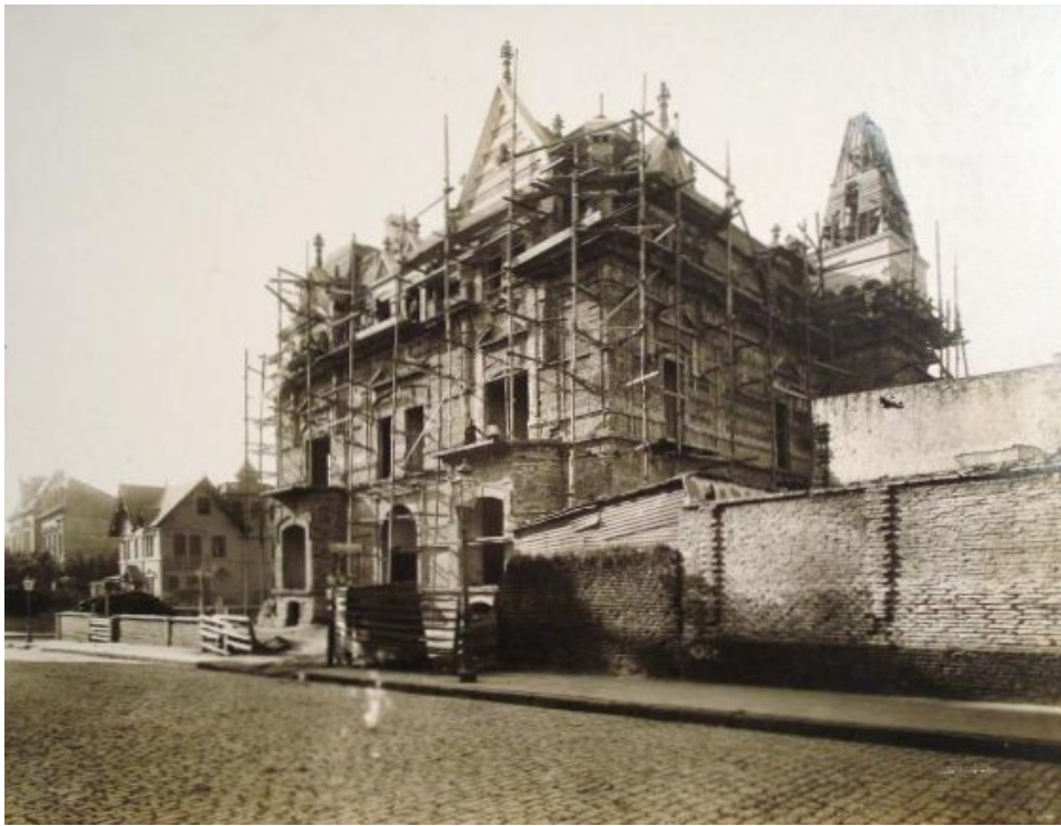
Figure 3–335. Hume Palace under construction 1891. Source: AGN
