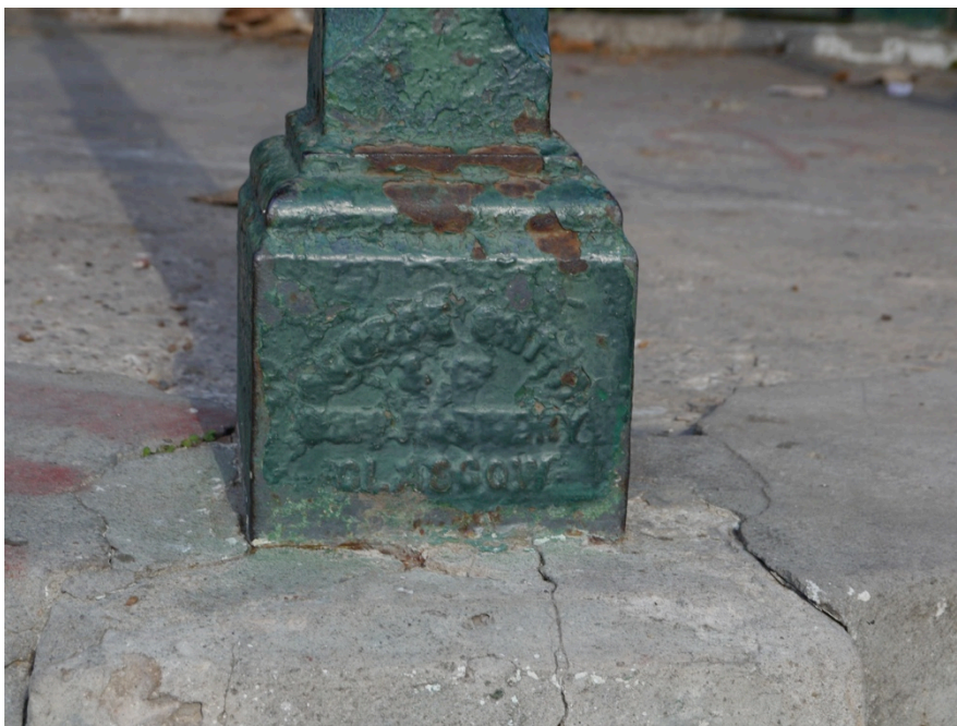
Figure 3–268. Nameplate on column base in gazebo made by George Smith in 3 de Febrero Park. Source: Photo Lucia Juarez
