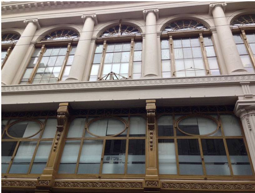
Figure 3–357. Detail of cast-iron front in façade, Maple Store in Buenos Aires. Source: Photo Lucia Juarez
