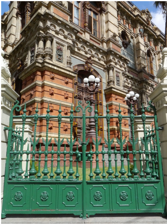
Figure 3–188. Macfarlane gate using railing model no. 28. Source: Photo Lucia Juarez
