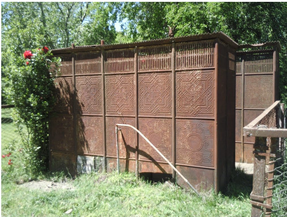
Figure 3–108. Macfarlane cast-iron urinal. Iraola Station. Source: Photo Federico Guerrero
