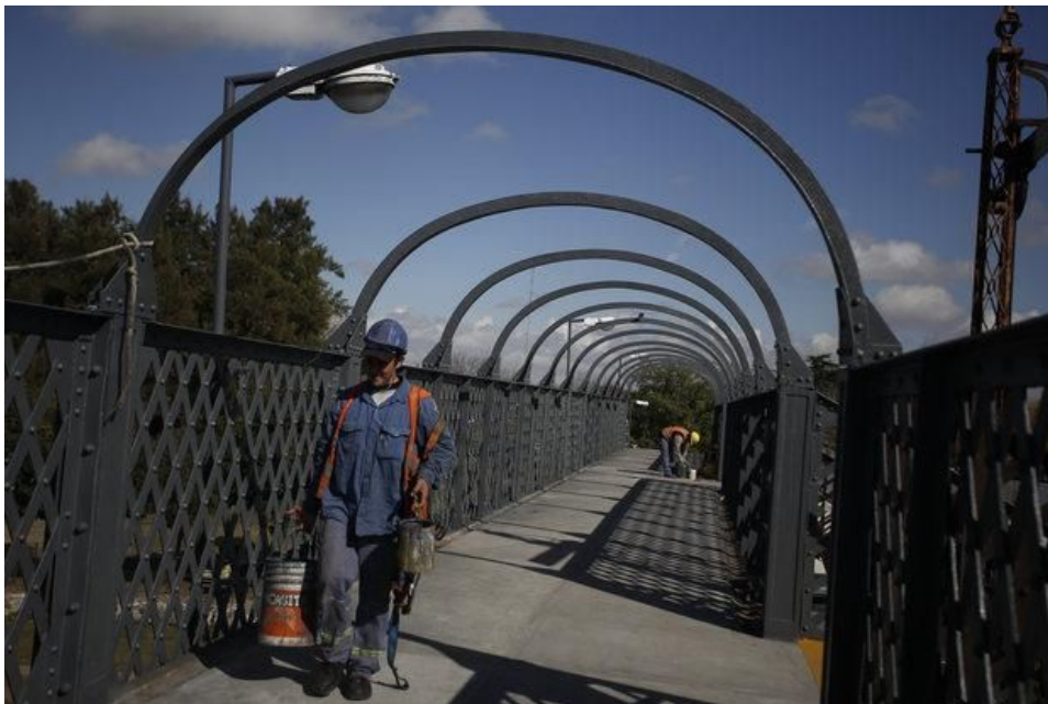
Figure 3–147. Tolosa footbridge in process of restoration. Source: ‘Recuperan el emblemático puente ferroviario de Tolosa’, http://www.eldia.com/nota/2015-5-11-recuperan-el-emblematico-puente-ferroviario-de-tolosa (accessed September 12, 2017).
