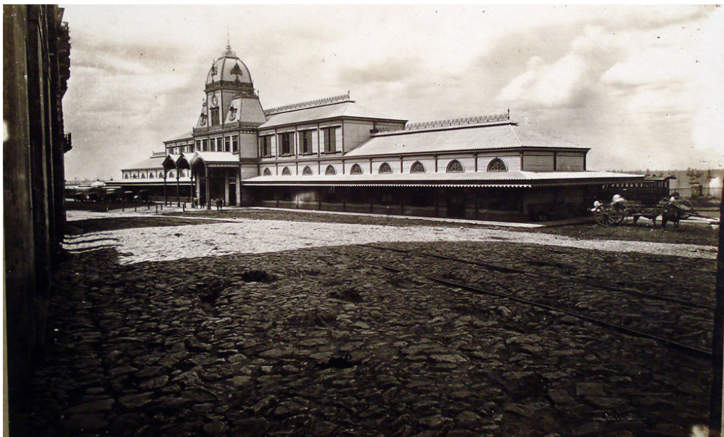
Figure 3–94. Central Station of Buenos Aires and Ensenada Port Railway. Source: AGN
