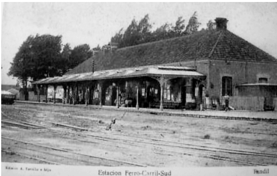
Figure 3–60. Tandil Station platform area (FCS). Source: FMF
