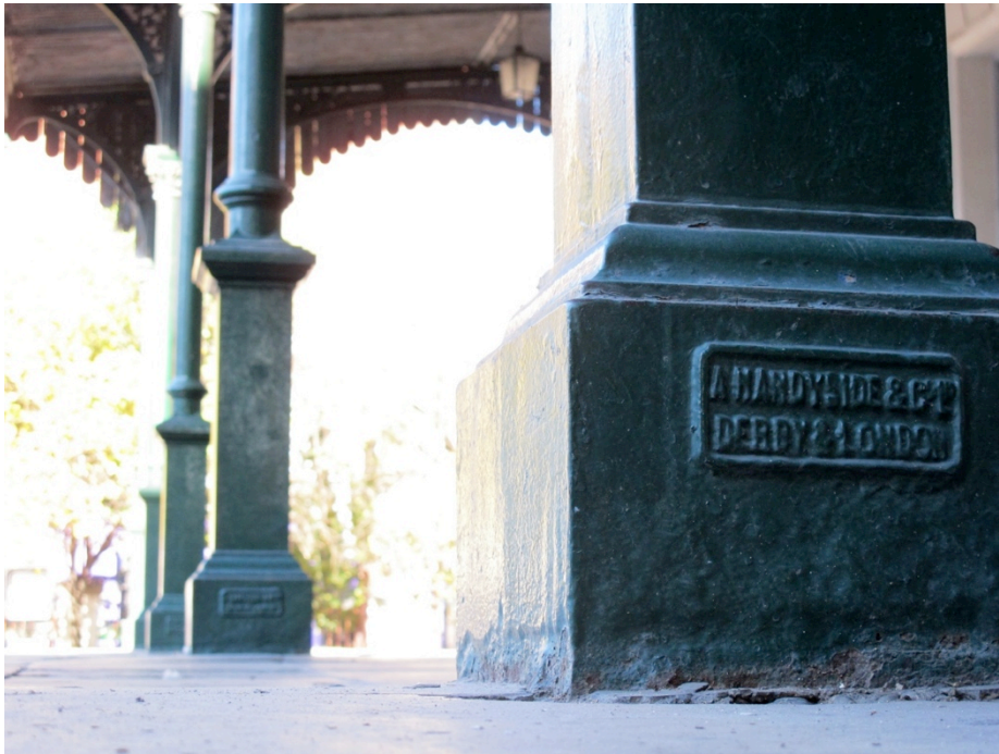
Figure 3–50. Mitre Station. Cast-iron column made by Handyside. Source: Photo Cecilia Laskowski
