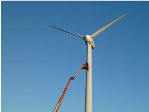
(a) Vestas V27 wind turbine with a hub height of 33.5 m and a 27m rotor diameter
