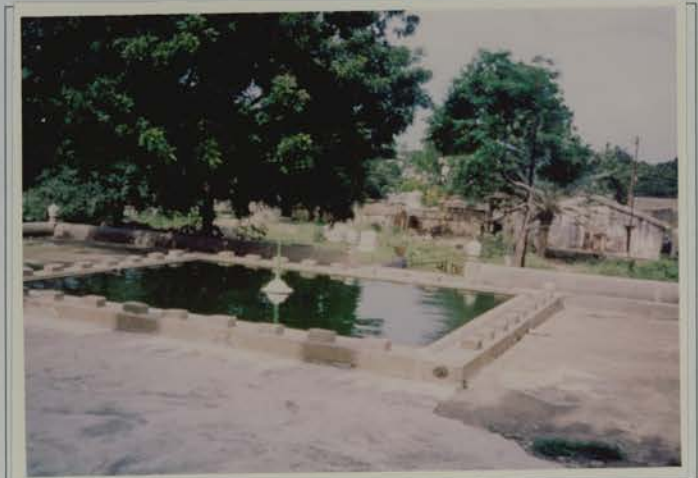
Fig 95 Toli Masjid, Karwan Hauz at garden level
