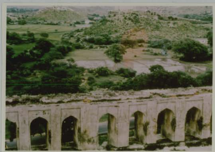
Fig 16 Mosque Pemamati Golconda (View from Baradari)
