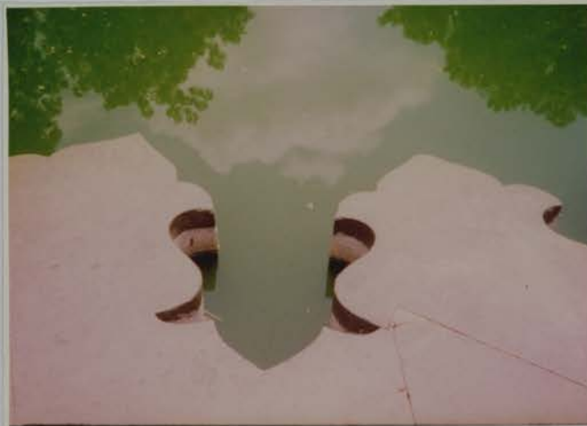
Fig 89 Lal Bagh, Bidar: Detail of water cistern
