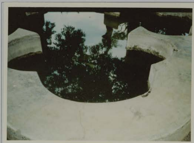
Fig 26 Nagina Bagh Golconda Detail water cistern
