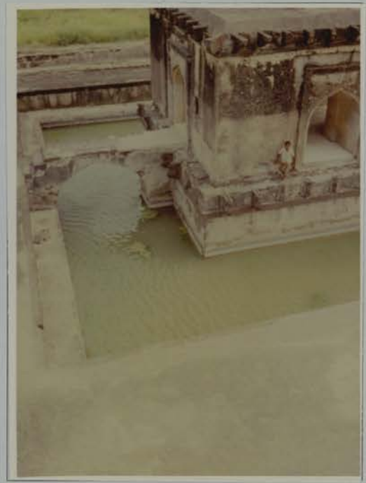
Fig 67 Kumatgi: Water pavilion
