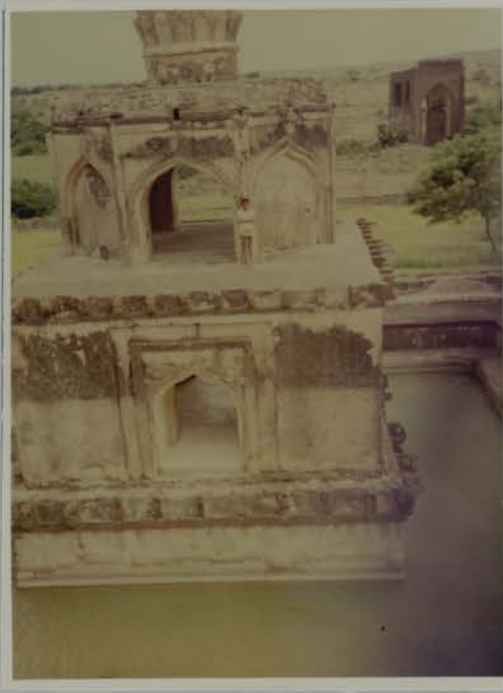
Fig 66 Kumatgi: Water pavilion
