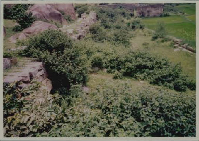
Fig 49 Watercourse to aqueduct
