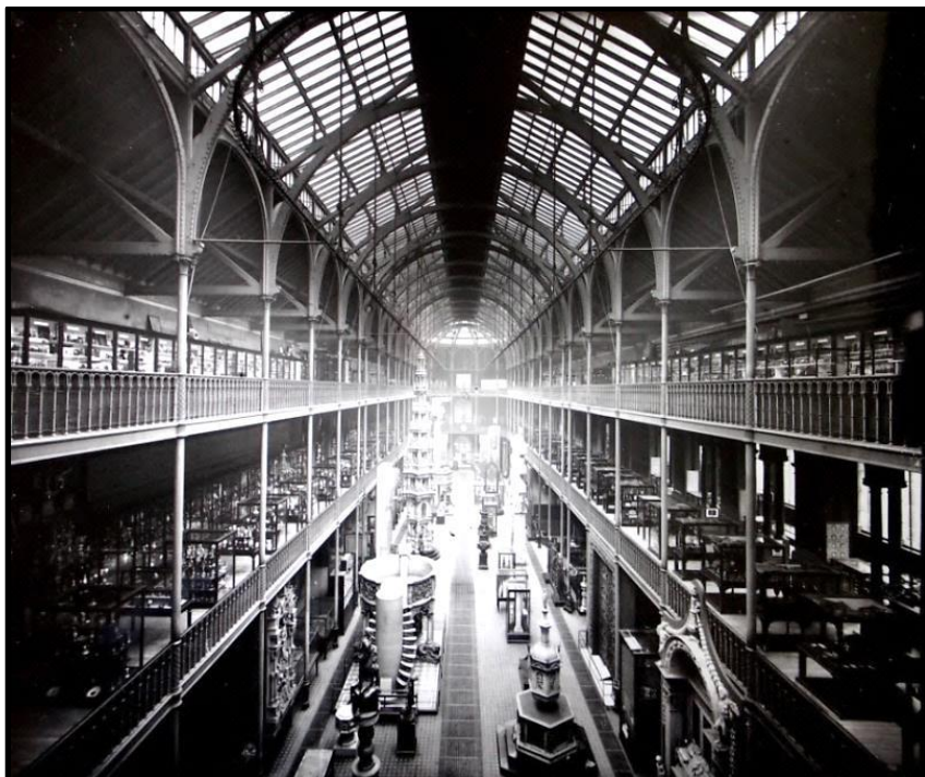
Figure 3.9. Photograph of the Great Hall circa 1900, showing Fowke and Matheson's leitmotif of a central atrium surrounded on two storeys by galleries (GB587/IS.2009.7/9).
