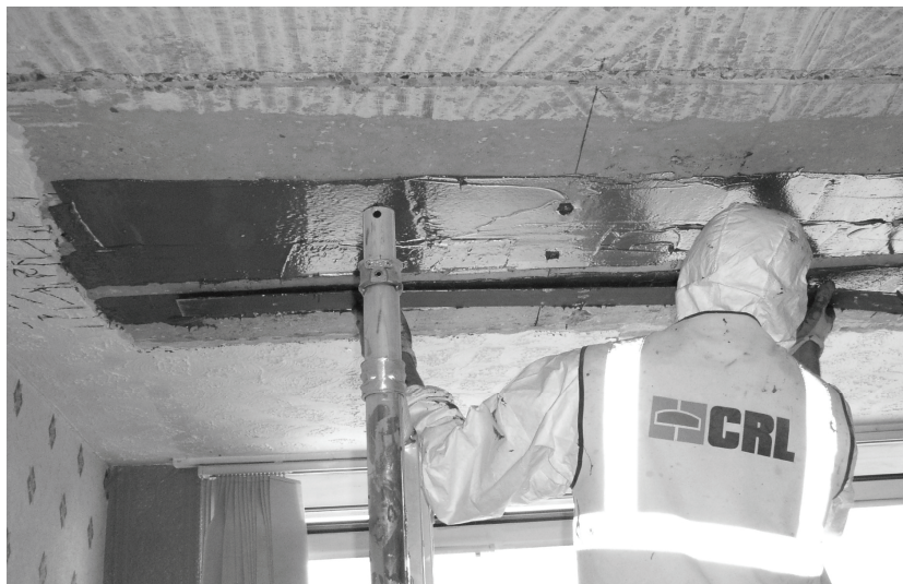
Figure 4: Installing a strengthening plate
