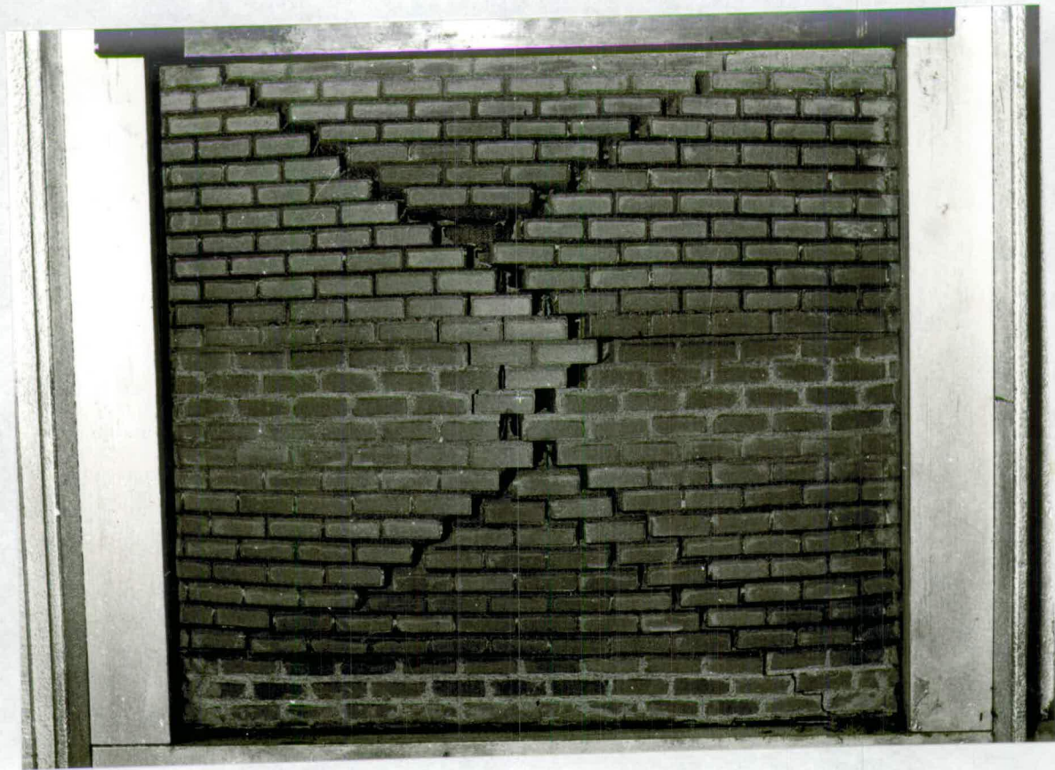
FIG. 5.9 FAILURE OF WALL D2 - 4 SIDES SUPPORTED
