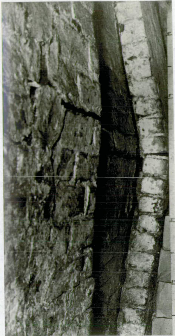
FIG. 4.1 BOND FAILURE WITH LOAD NORMAL TO FACE
