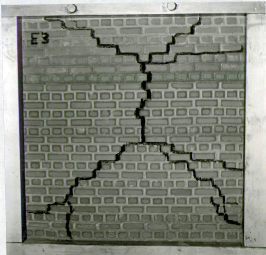
FIG. 5.11 FAILURE OF WALL E3 - 4 SIDES SUPPORTED
