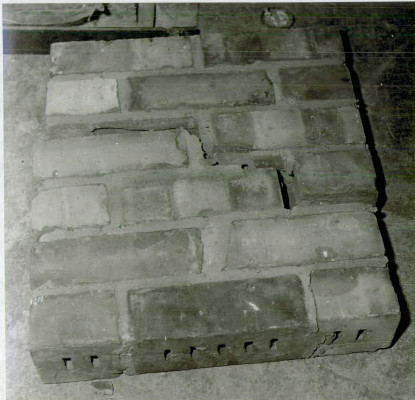
FIG. 7.32 FAILURE OF A WALLETTE OF THE SECOND SERIES
