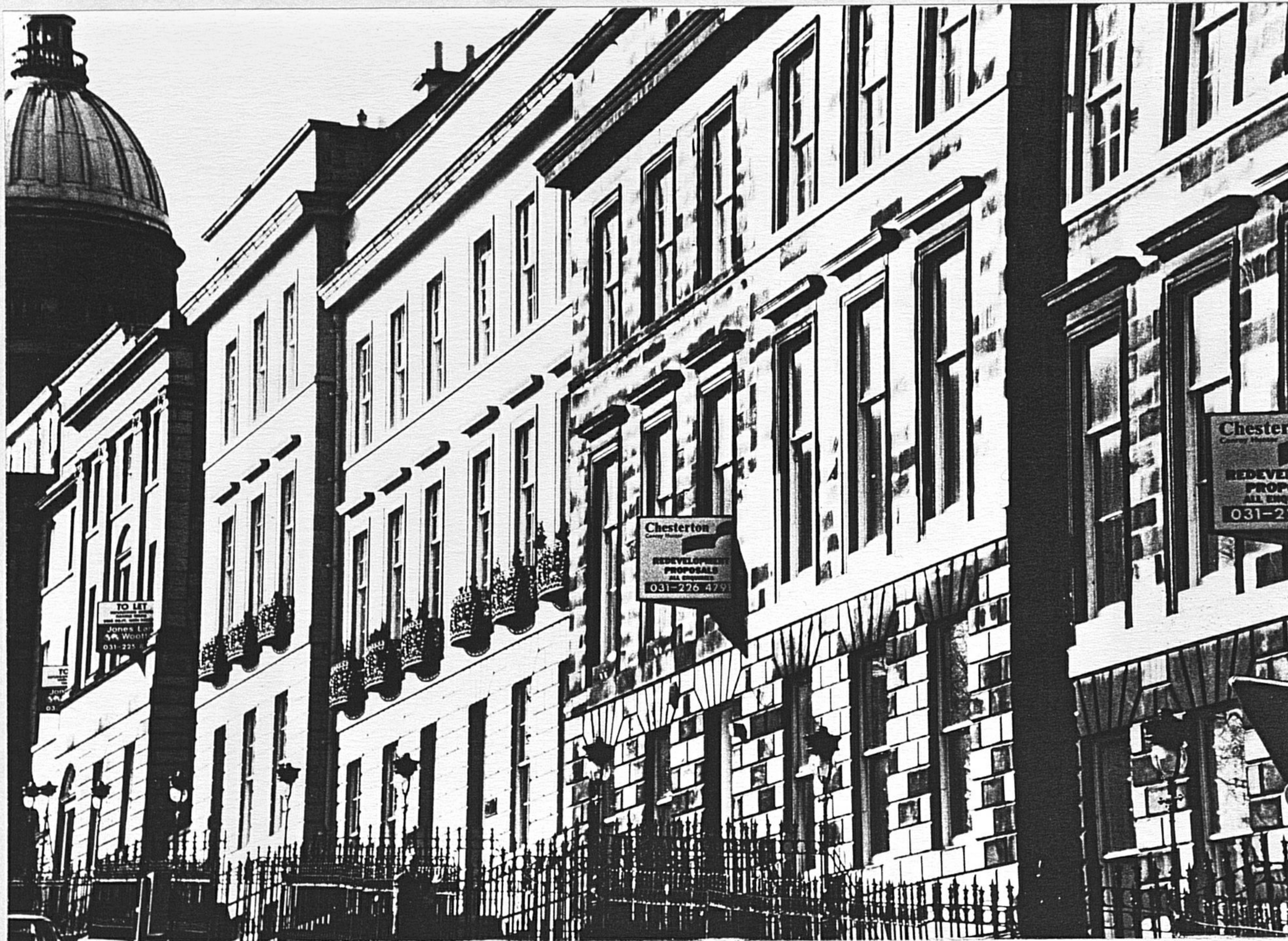
47 New Town Facadism: Offices in Glenfinlas Street, Edinburgh, 1990. The lighter facade on the left of the picture is new, with modern offices built behind.
