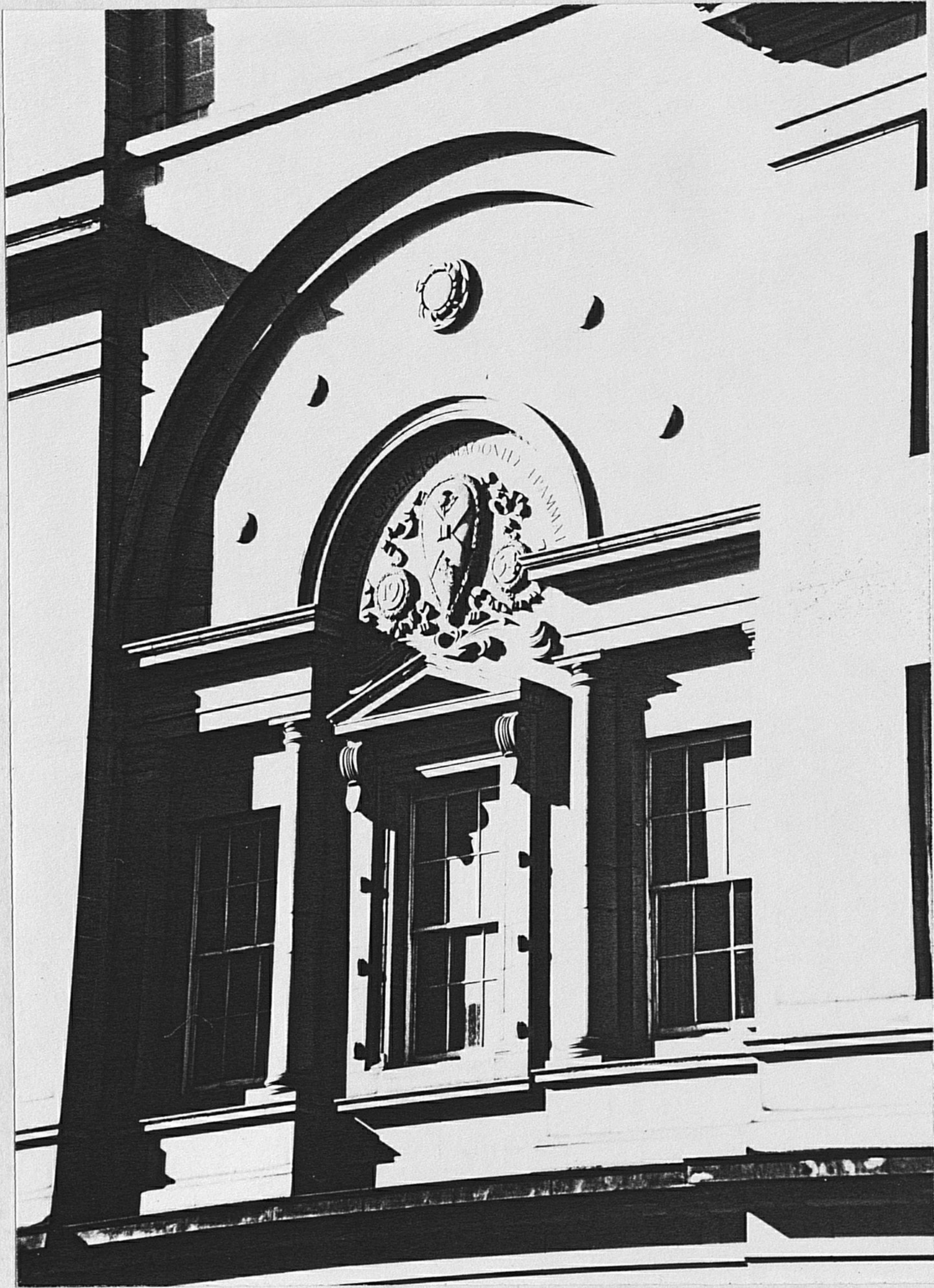
24 Adam House: first floor central windows.
