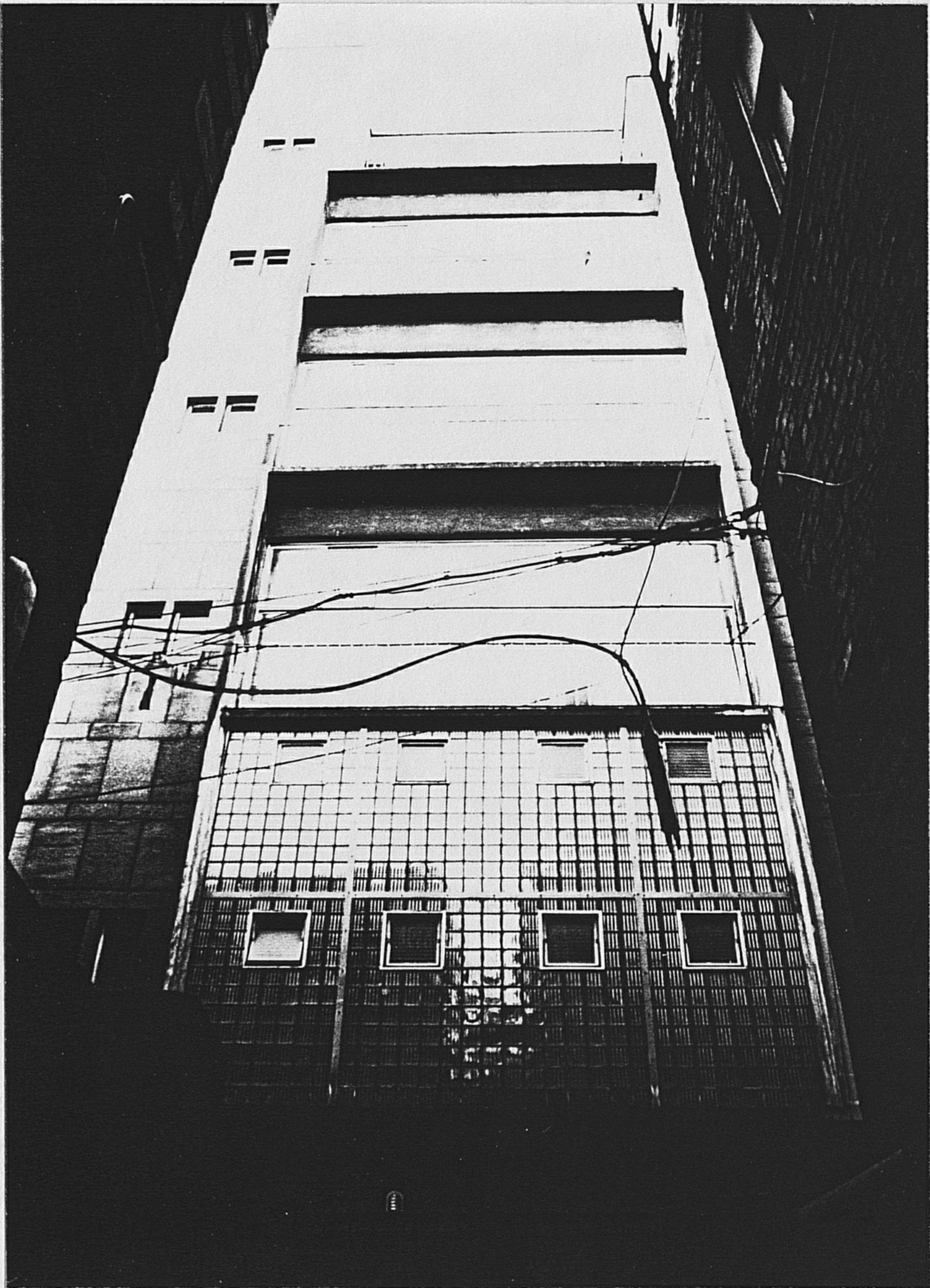
27 Adam House: rear elevation, general view.
