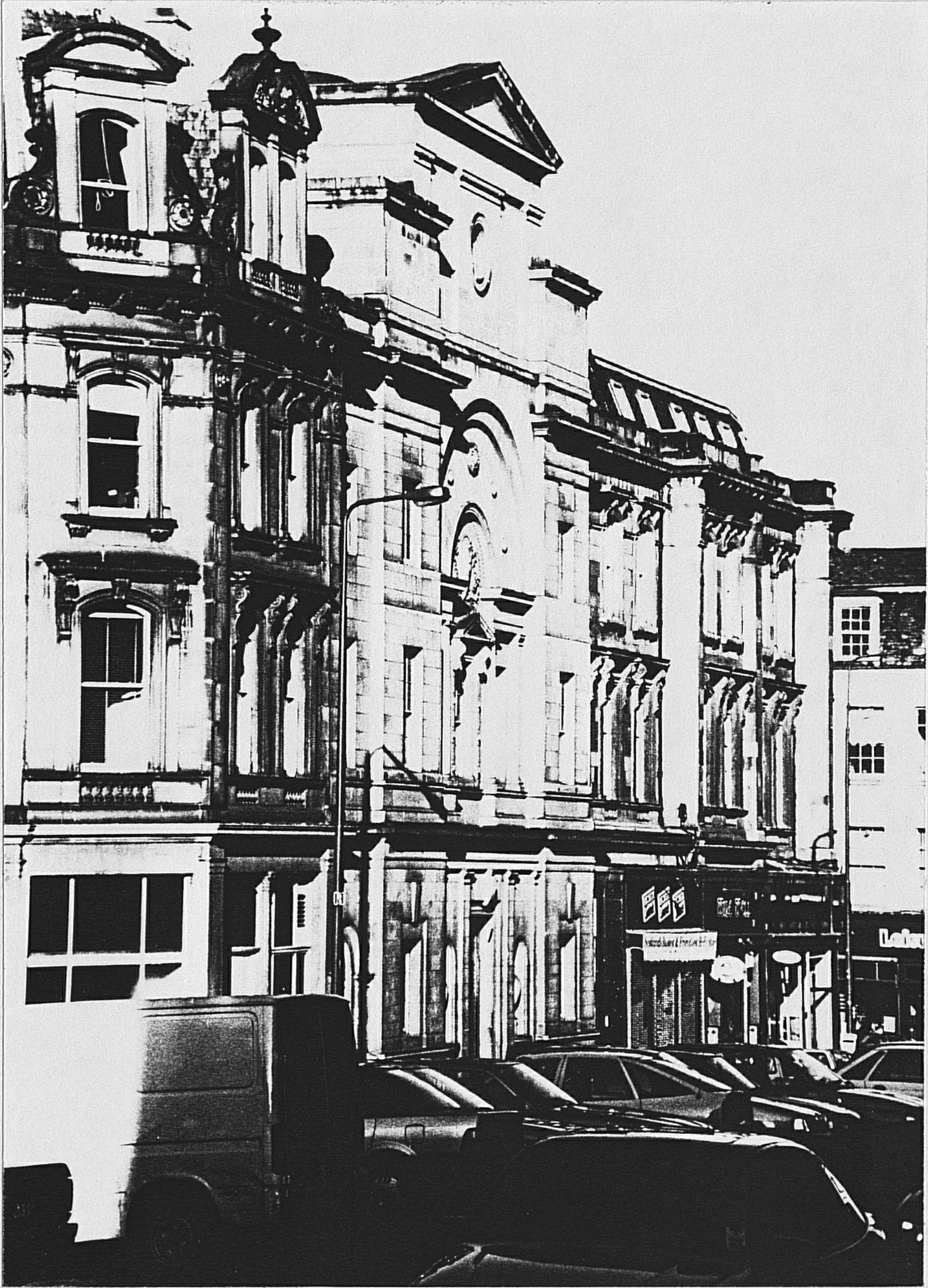
46 Adam House: general exterior view within Chambers Street.
