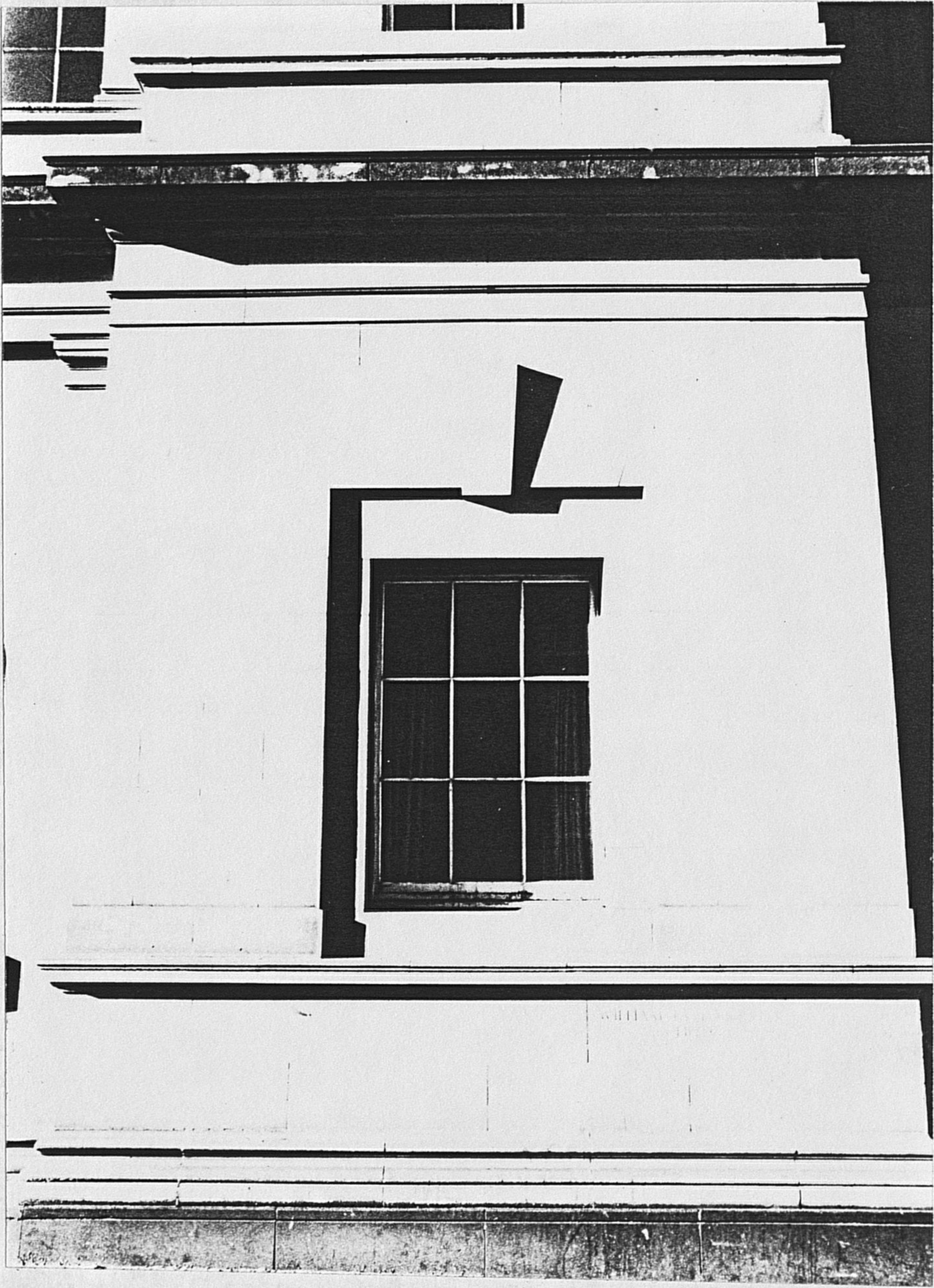
18 Adam House: ground floor side window.
