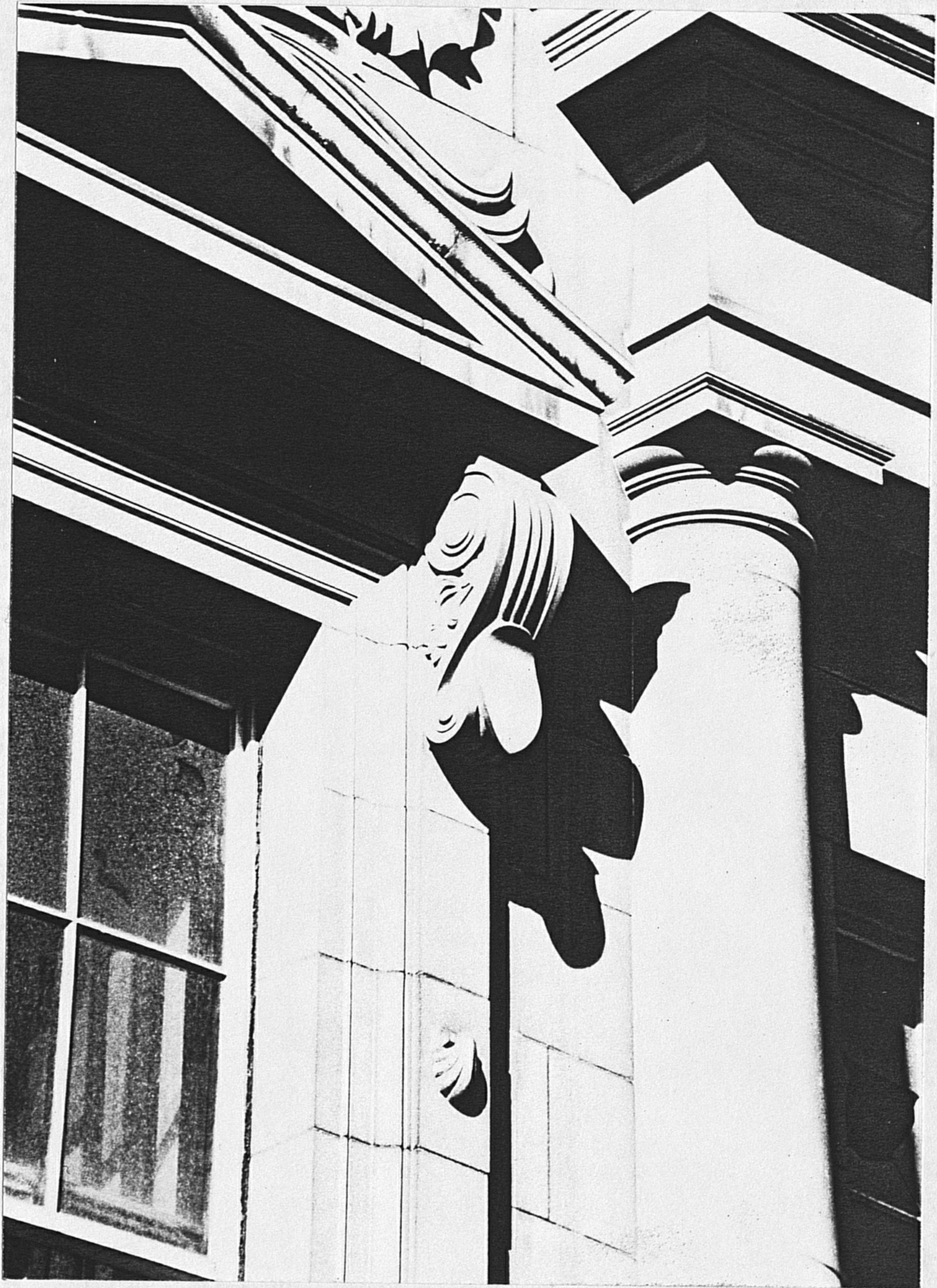
38a Adam House: central first floor window, detail.
