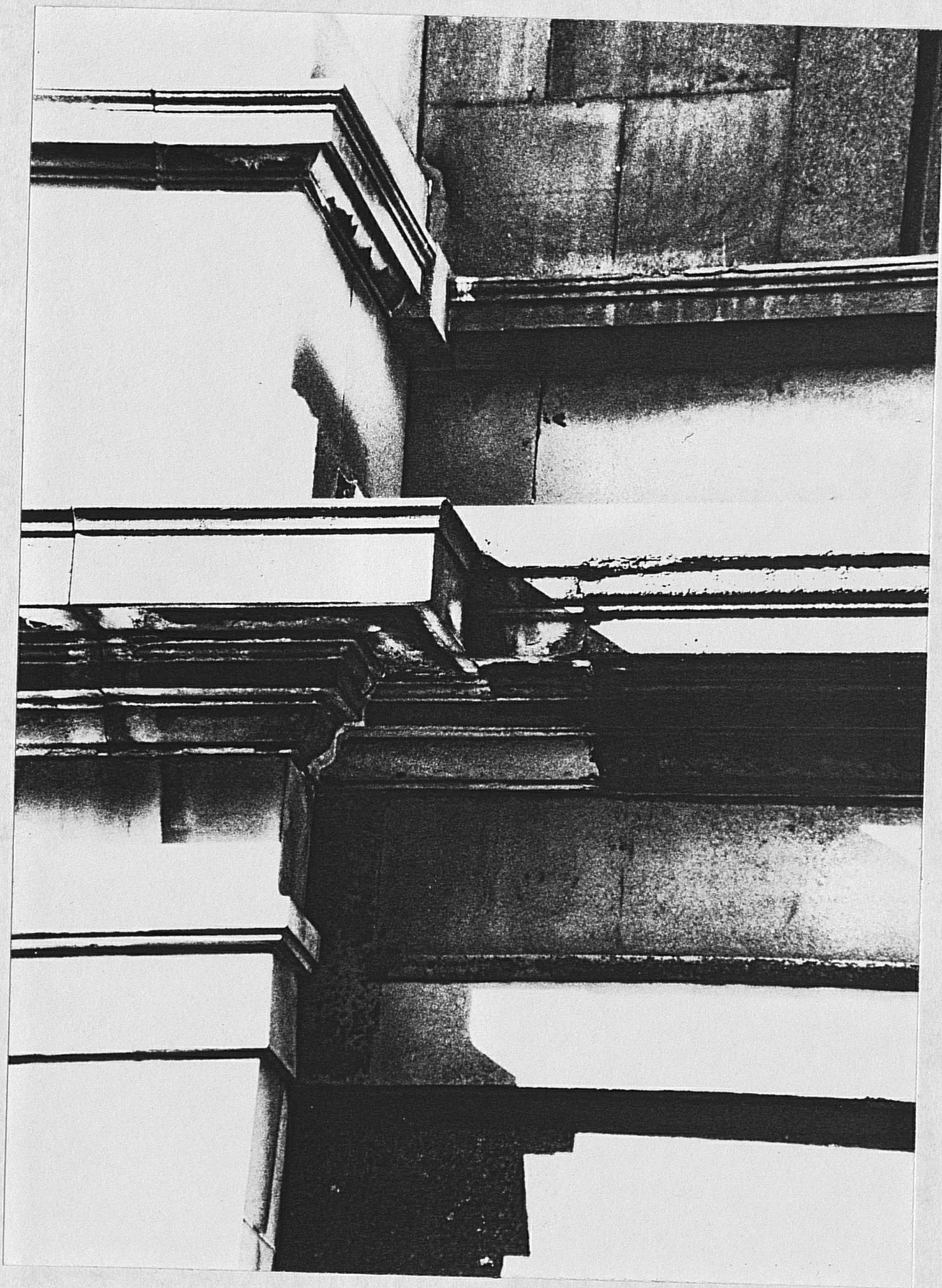
26b Adam House: first floor entablature, detail.
