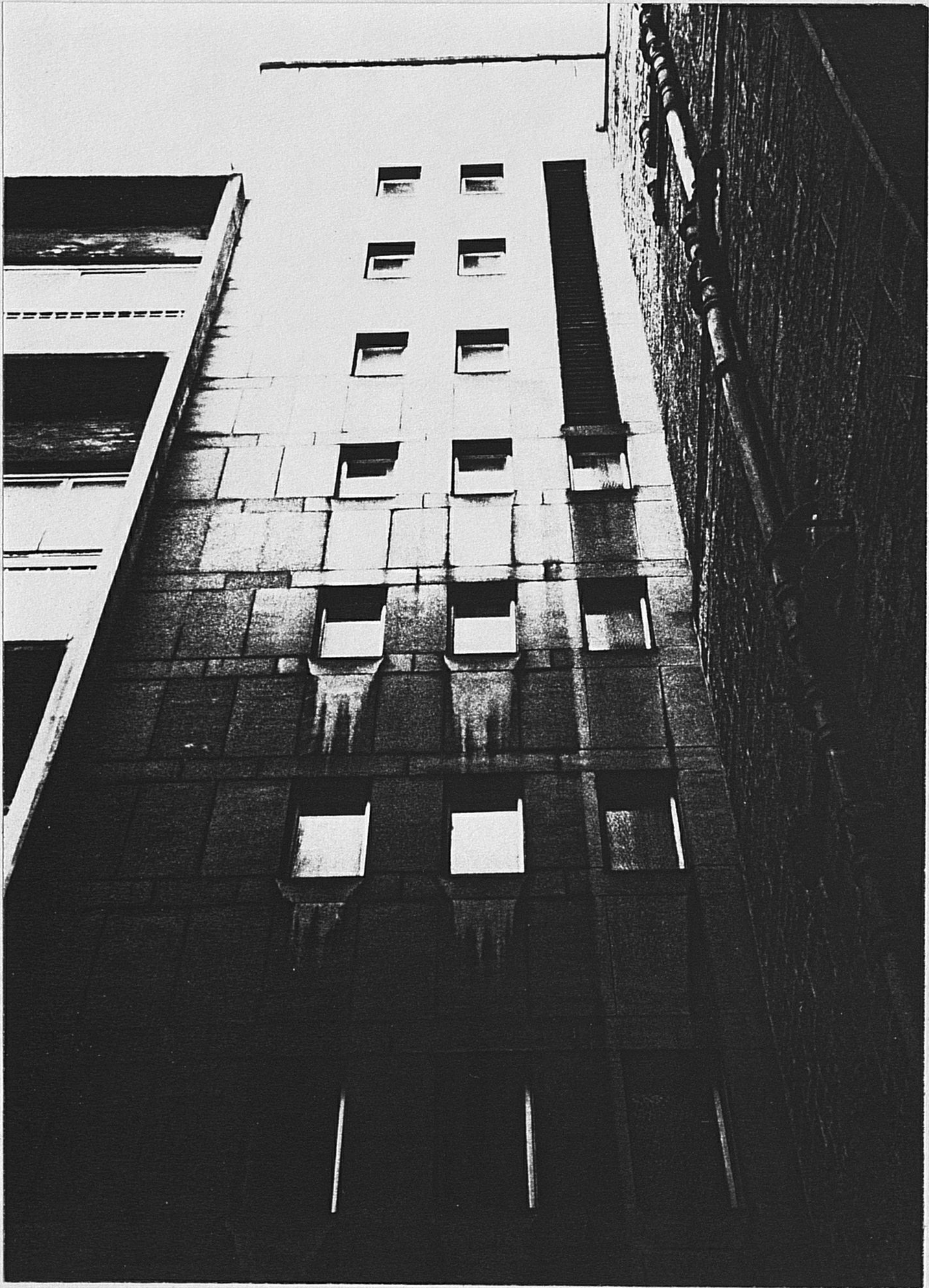
28b Adam House: rear elevation, detail showing concrete panels.
