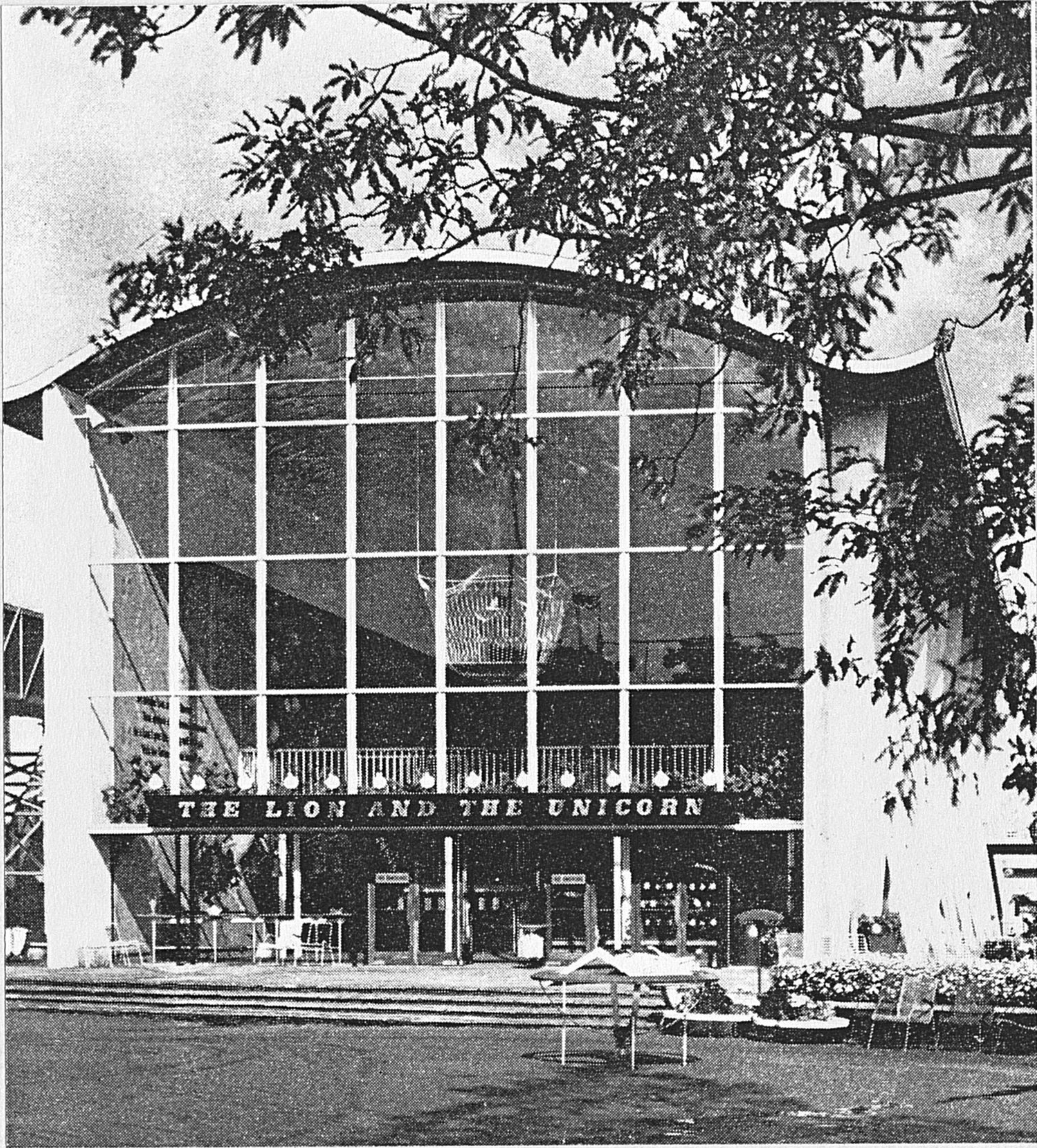
37 R. D. Russell and Robert Goddenn: The Lion and the Unicorn Pavilion, South Bank, 1951, south elevation.
