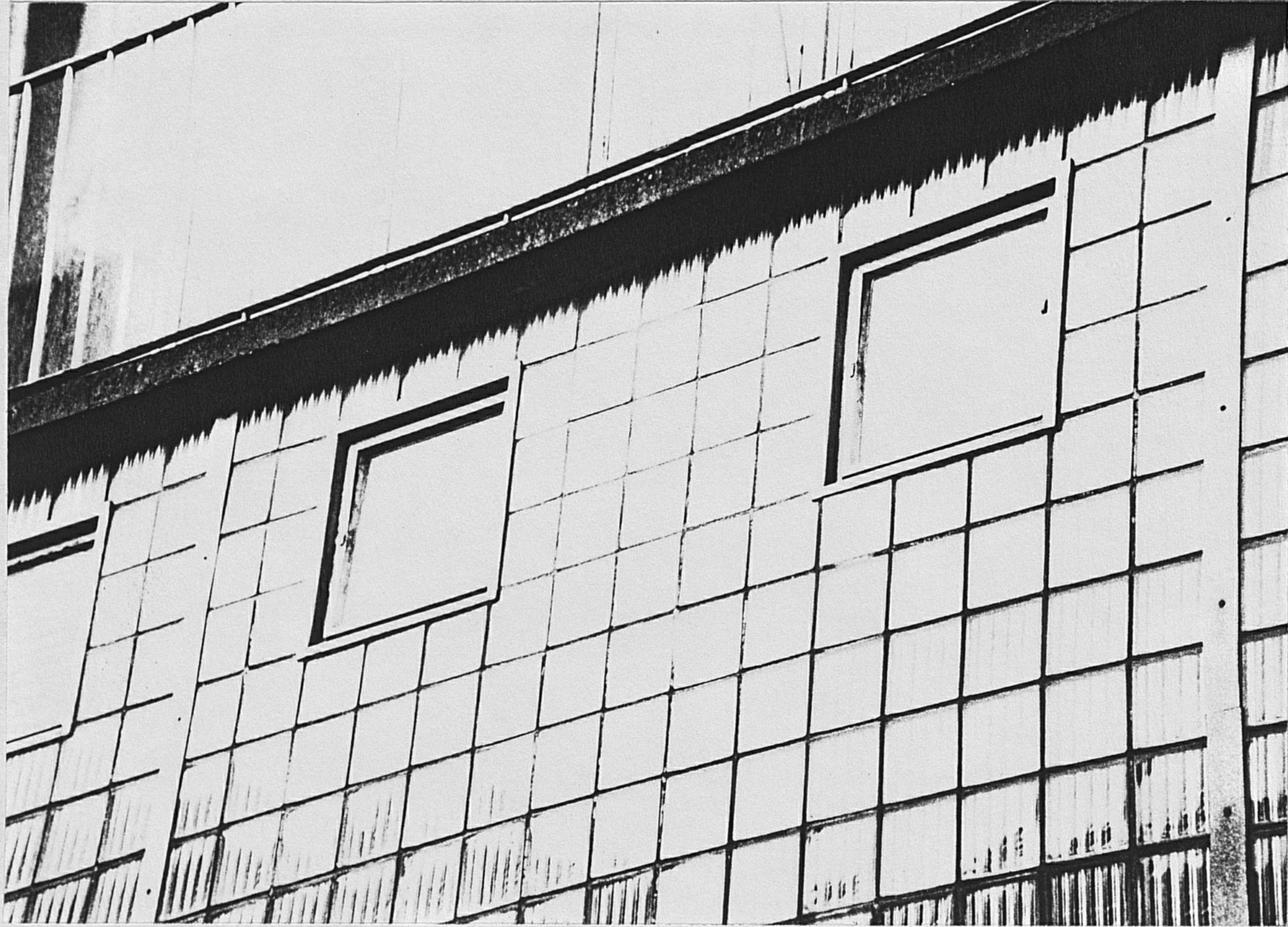
28a Adam House: rear elevation, detail showing glass bricks.
