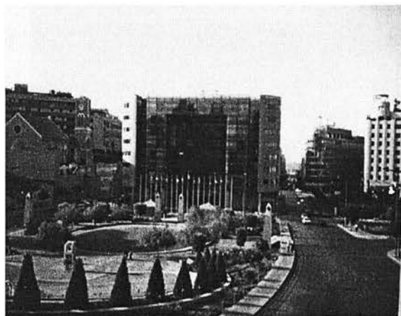
Figure 5-7: Jbran Khalil Jbran park facing the ESCWA building. The public rarely uses this park (source: the author, 2001).
