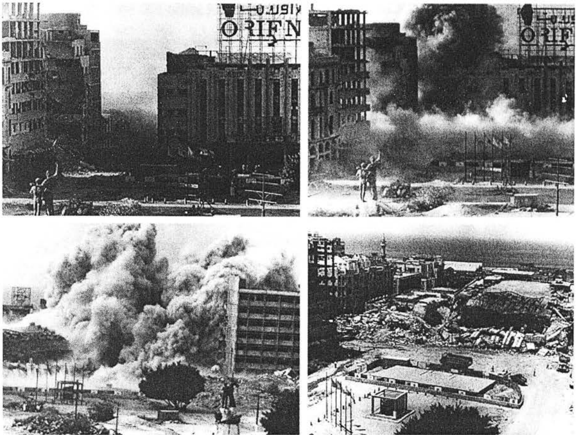
Figure 4-12: The Rivoli building (Orient) in Martyrs' Square, among the buildings marked for demolition, although it was structurally sound (source: Tueni and Sassine, 2000, p.202).
