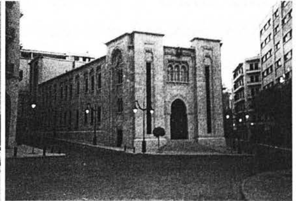
Figure 5-21: The Parliament Building located at al-Nijmeh Square (source: the author, 2002).
