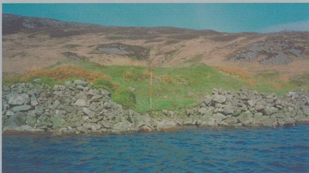
Loch Allalaidh: Walling and boat noost Looking North
