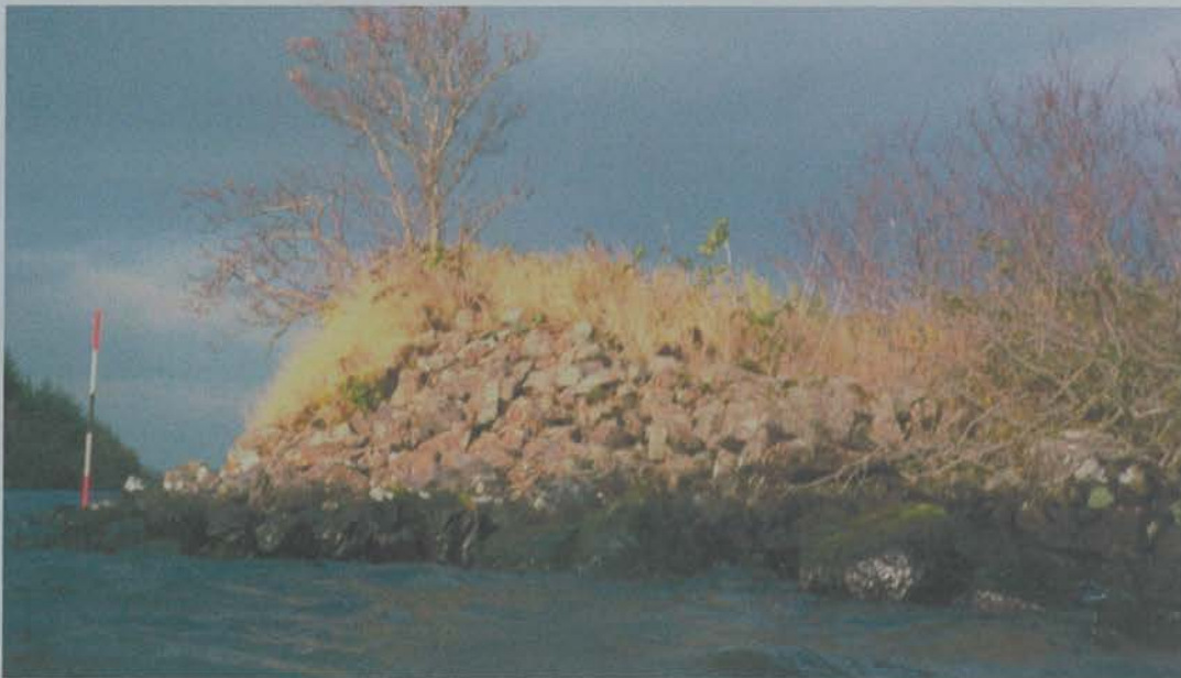
Eilean Ban: Section of walling Looking North
