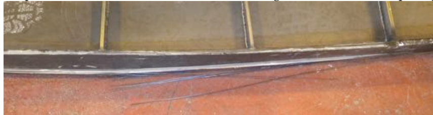
c) CFRP locally damaged on one edge
