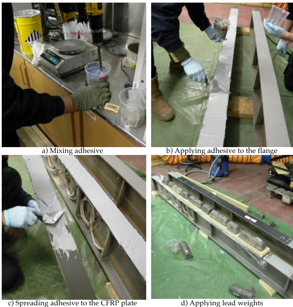
Figure 4-9: Various stages of the CFRP plates strengthening
