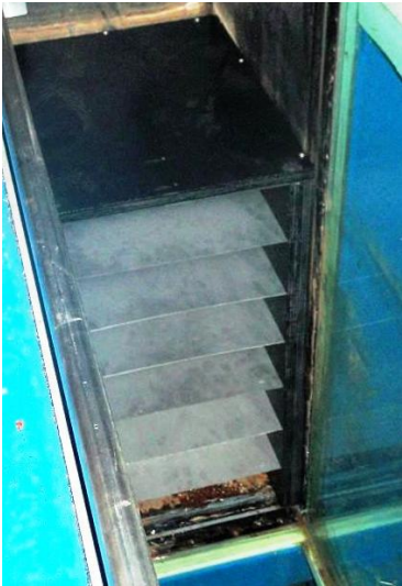
(b) Completed turning vanes installed in the flume
