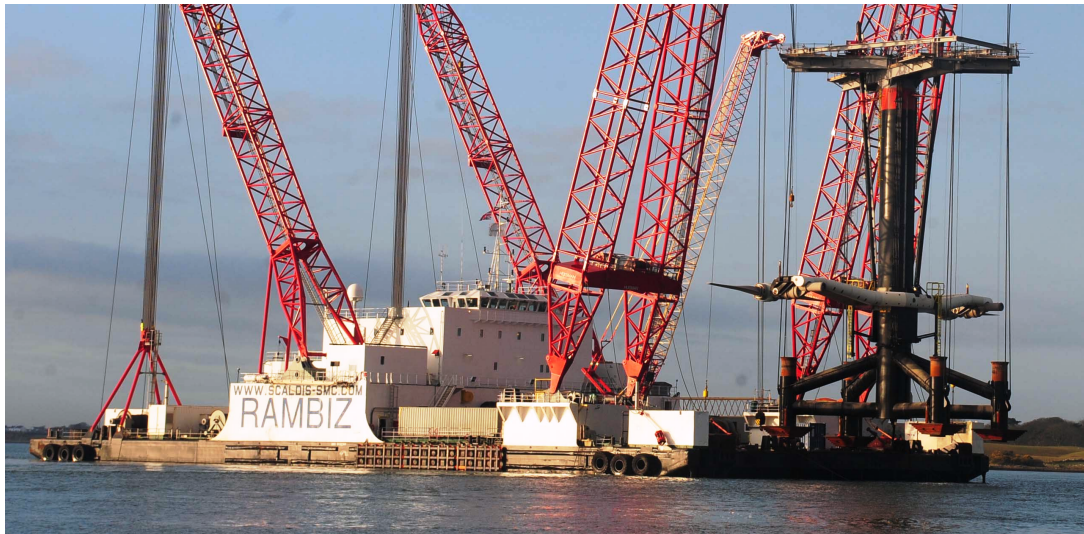
Figure 1.7: Installation of MCT SeaGen jacketed pile foundation (Maritime Journal, 2008)
