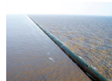
(c) Completion of construction project
