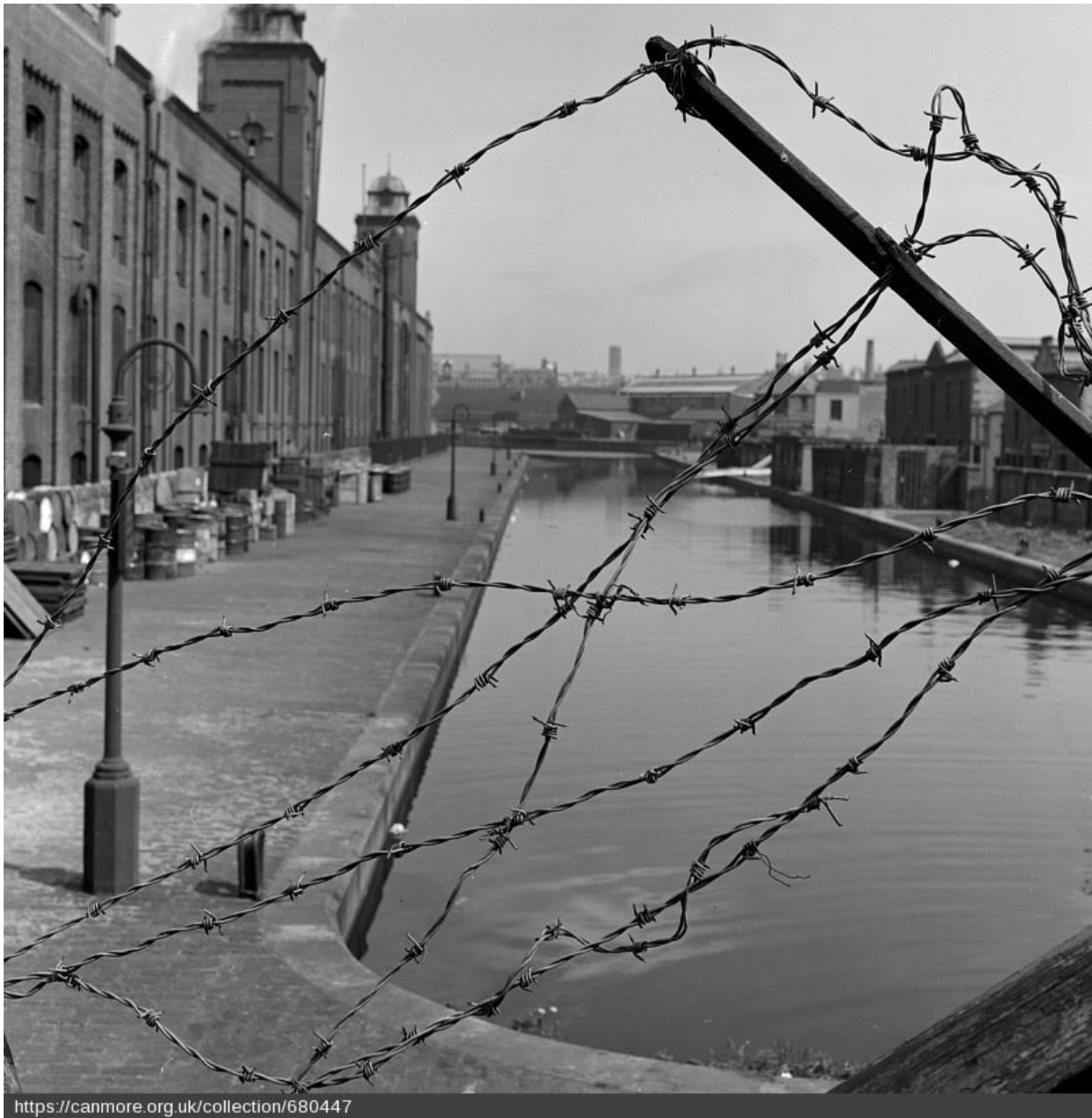
Figure 4. Union Canal and Castle Mills rubber factory ~1957 (Canmore, no date c)
