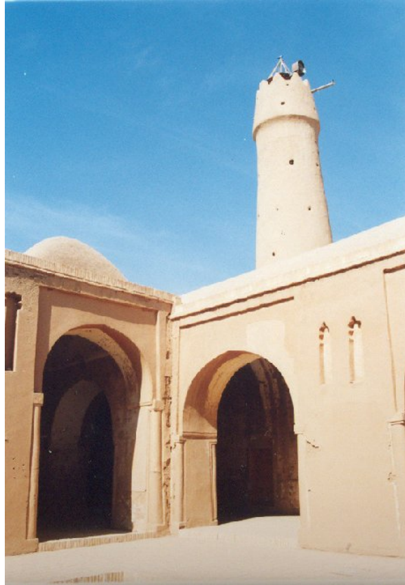
Pl.3.5. Friday mosque Fahraj. View of the minaret.
