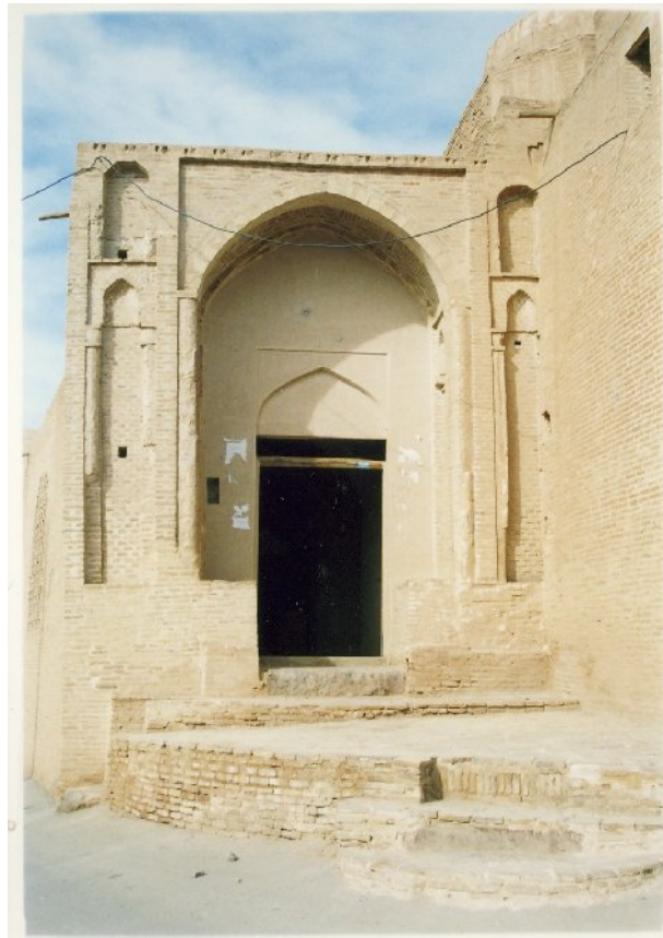
Pl.6.4.Friday mosque, Ardistan. The entrance on the south-west.
