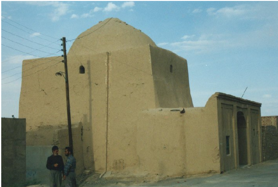
Pl.25.2. Pīr-i Ḥamza Sabzpūsh. The south-east façade.
