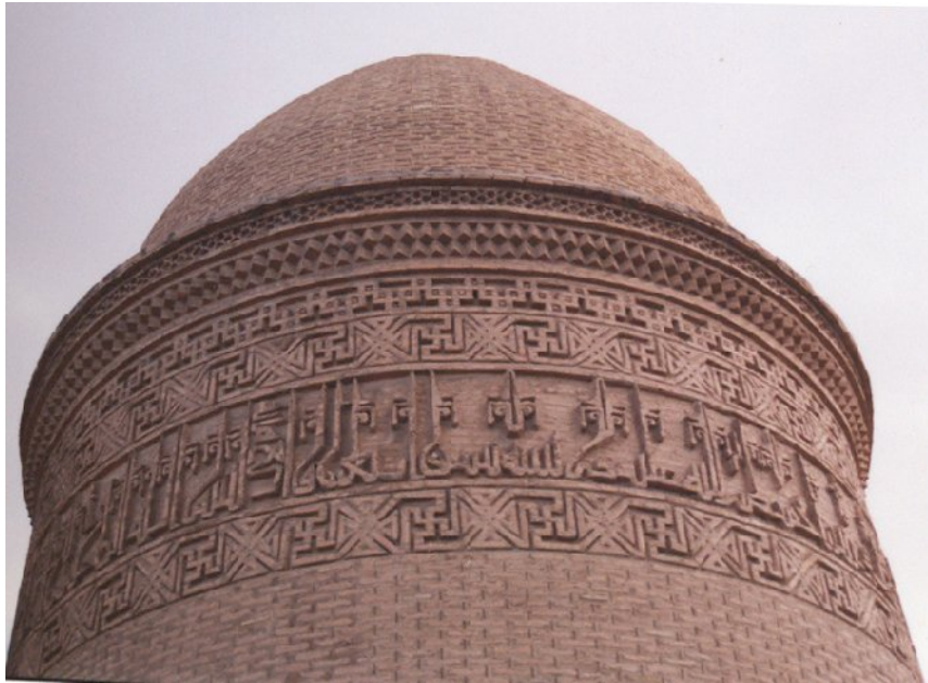
Pl.22.3. Chihil Dukhtarān. Decoration below the roof.
