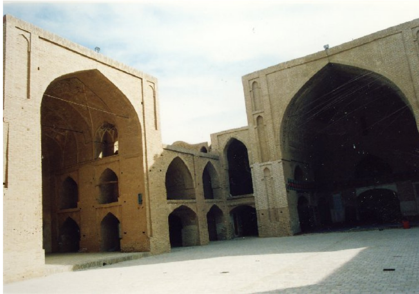
Pl.6.1.Friday mosque at Ardistan. View of south-eastern and south-western iwāns .
