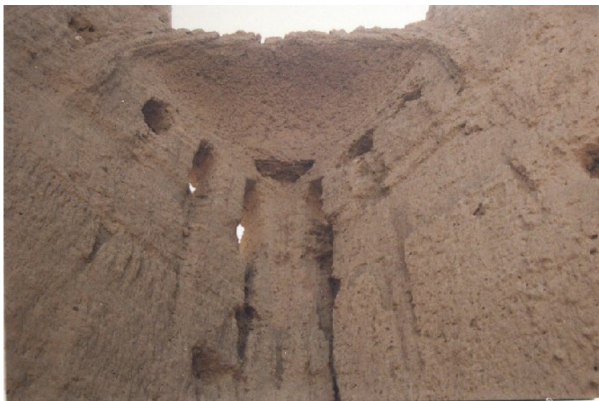
Pl.13.4. Kūshk-i Raḥīmābād, Bam. South-western squinch of the dome chamber.
