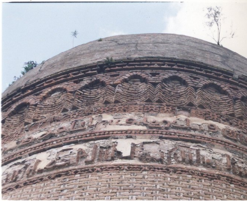
Pl.20.3. Tomb tower at Lājīm. Blind outset arches beneath the roof.
