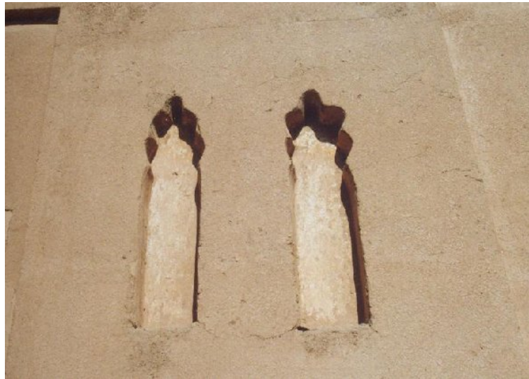
Pl.3.8. Friday mosque, Fahraj. View of blind lobed arch with an ogee apex.
