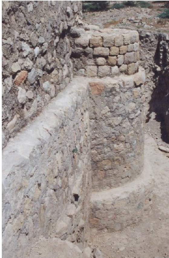
Pl.14.2. Mosque at Bishāpūr. Remains of a round tower.
