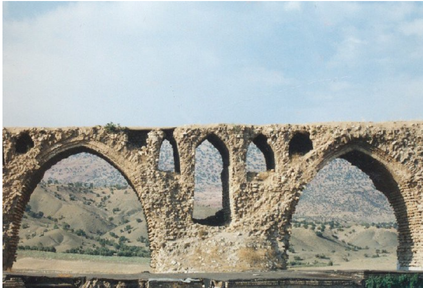
Pl.11.2. Kashkān Bridge. View of two bays.
