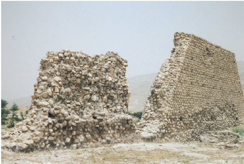
Pl.14.6. Mosque at Bishāpūr. Remains of the northern wall.
