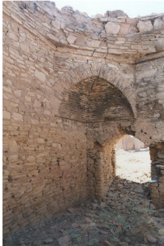
Pl.24.7. Caravansarai at Muḥammadābād. View of a squinch of baked brick.
