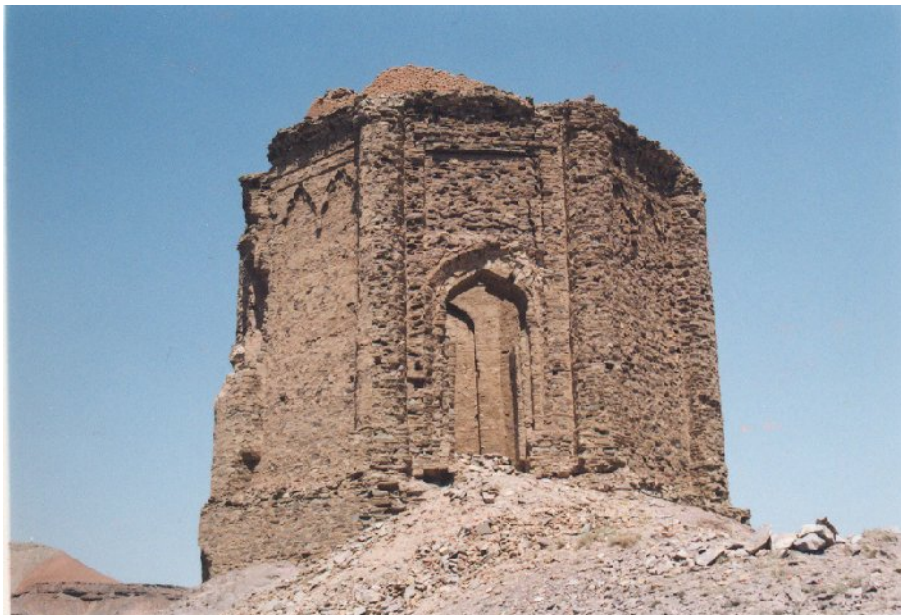
Pl.9.2.Tomb tower, Samīrān. View of doorway.
