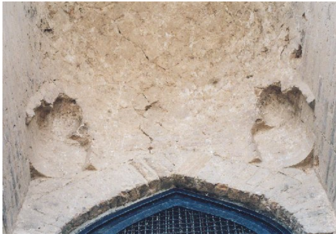
Pl.10.4.Gunbad-i Qābūs. A pair of squinches above the doorway.
