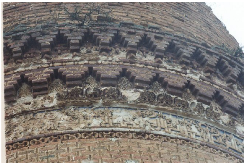
Pl.27.2. Tomb tower at Risgit. Decoration beneath the cornice.
