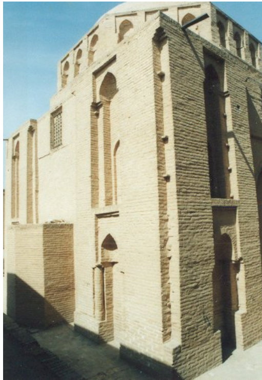
Pl.21.2. Davāzdah Imām. View of south-eastern corner.
