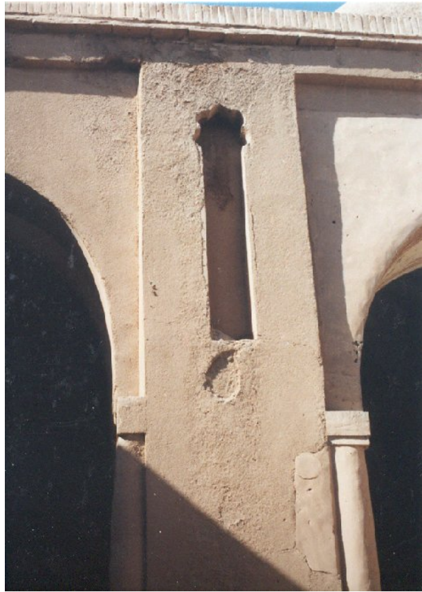
Pl.3.7. Friday mosque, Fahraj. View of blind lobed arch with a pointed apex.
