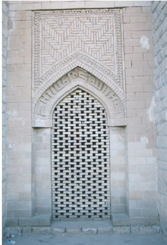
Pl.2.6. Friday mosque, Shūshtar. Exterior façade , grilles of open-jointed brickwork.
