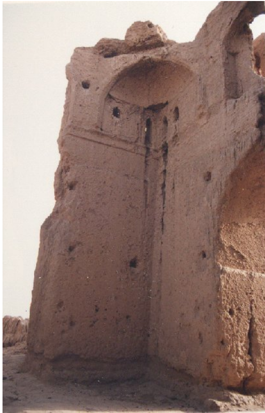
Pl.13.3. Kūshk-i Raḥīmābād, Bam. North-eastern squinch of the dome chamber.
