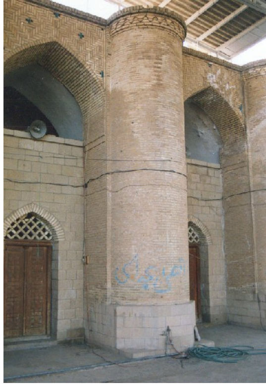
Pl.2.5. Friday mosque, Shūshtar. Exterior façade, projecting semi-circular pier.
