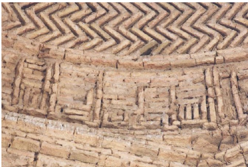
Pl.26.11. Mausoleum at Sangbast. Detail of inscription around the base of dome.
