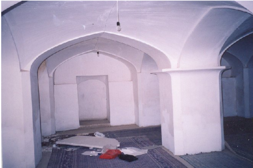
Pl.16.5.Friday mosque, Simnan. Quadrupartite vault of south-eastern basement.
