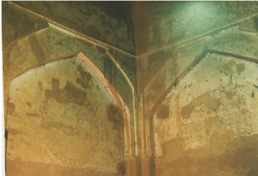
Pl.25.4. Pīr-i Ḥamza Sabzpūsh. View of double reverse broken arch.
