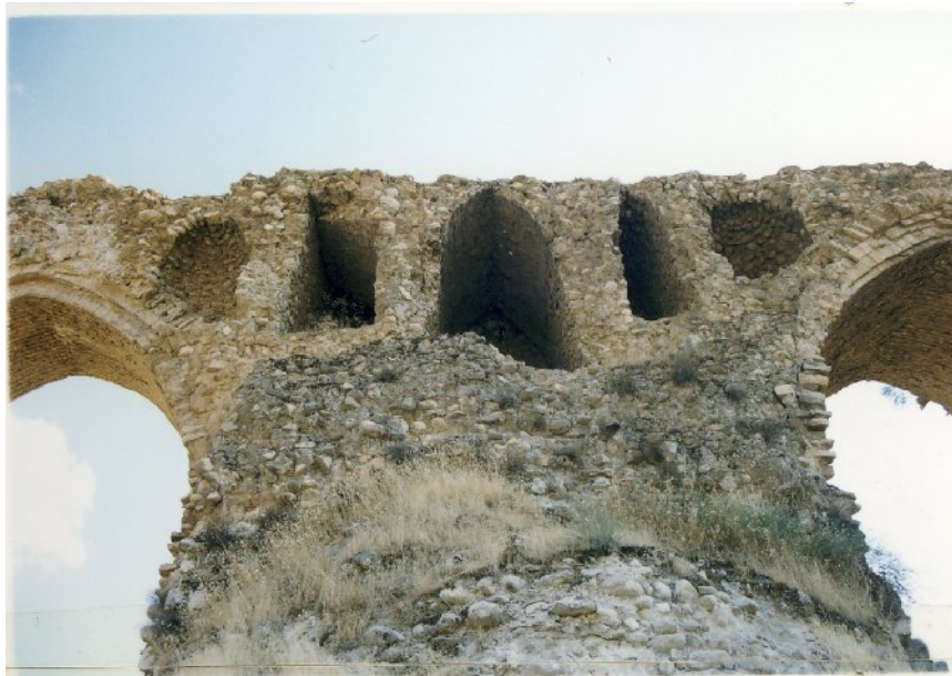
Pl.11.4. Kashkân Bridge. View of openings over each pier.
