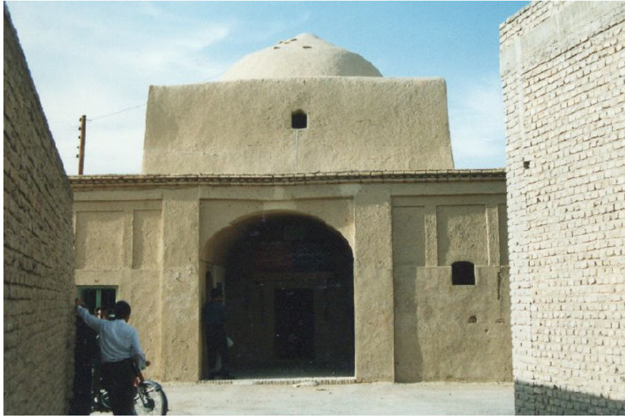
Pl.25.1. Pīr-i Ḥamza Sabzpūsh. The north-east façade.
