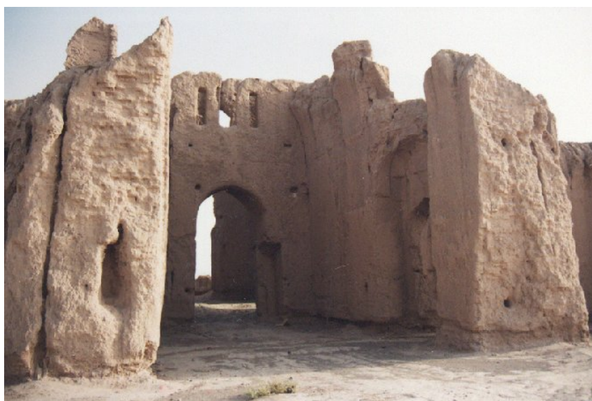
Pl.13.2. Kūshk-i Raḥīmābād, Bam. View of south-western īwān .
