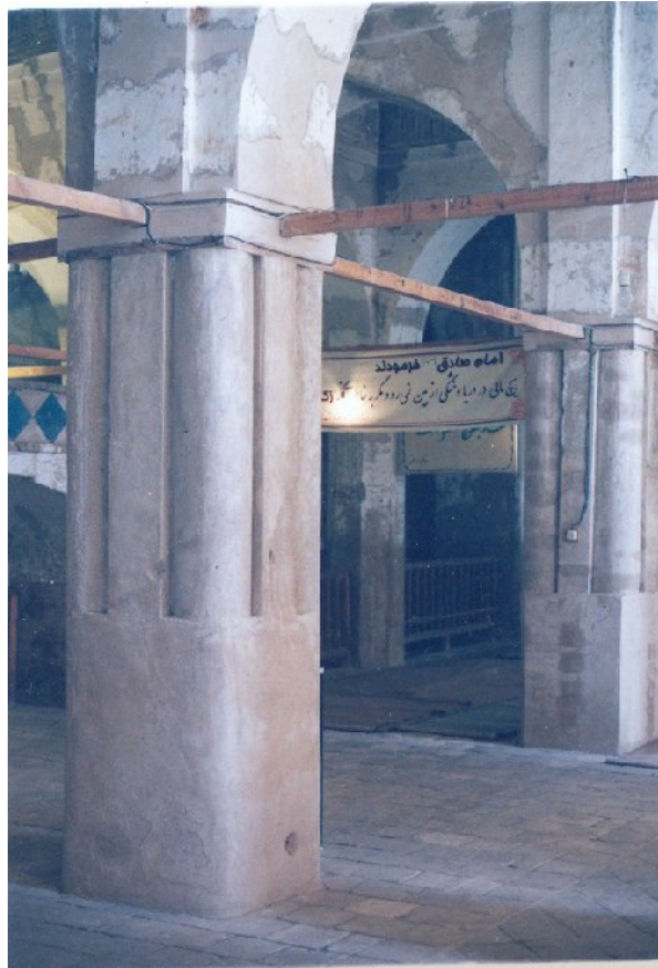
Pl.8.7. Friday mosque, Na'in. A pier with engaged columns.
