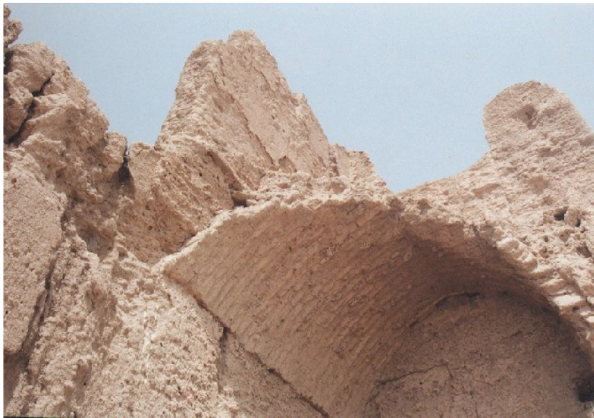
Pl.13.6. Kūshk-i Raḥīmābād, Bam. Remains of a barrel vault on the south-east.
