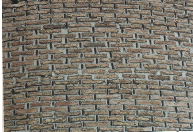
Pl.18.3. Tomb tower at Rādkān West. Vertically impressed joints.
