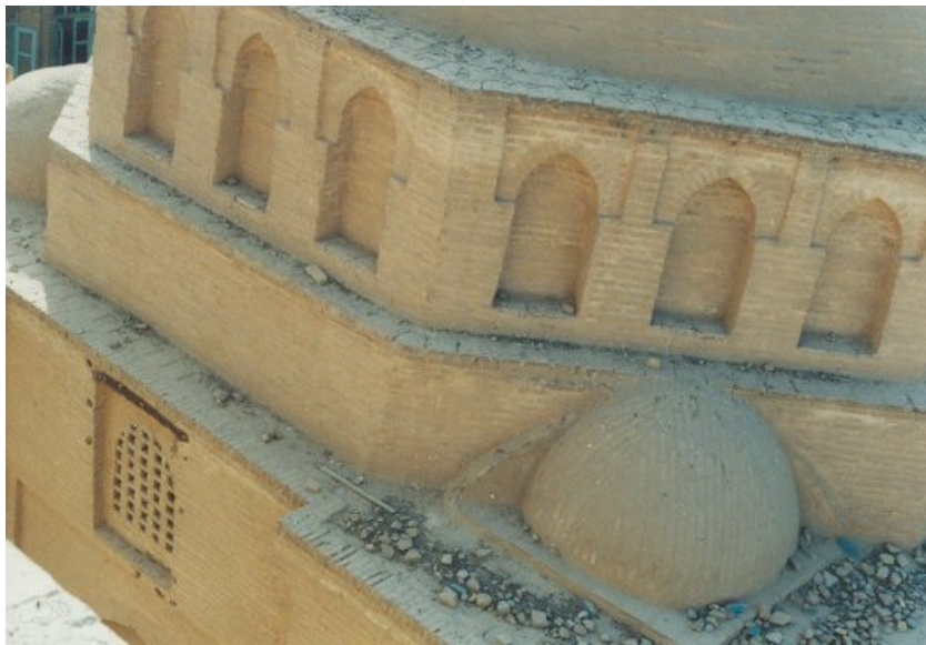
Pl.21.5. Davāzdah Imām. View of a quarter-dome on the roof.
