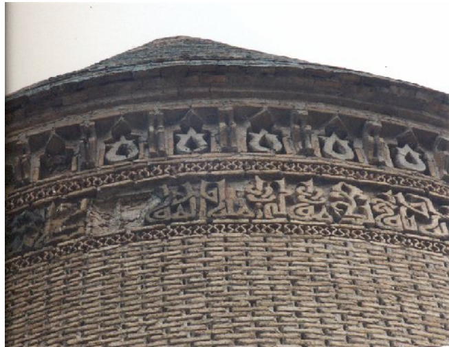
Pl.18.4. Tomb tower at Rādkān West. View of decoration beneath the roof.
