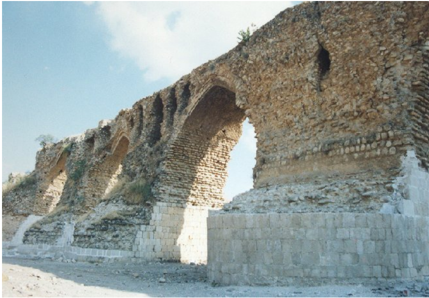
Pl.11.3. Kashkân Bridge. Base of piers.
