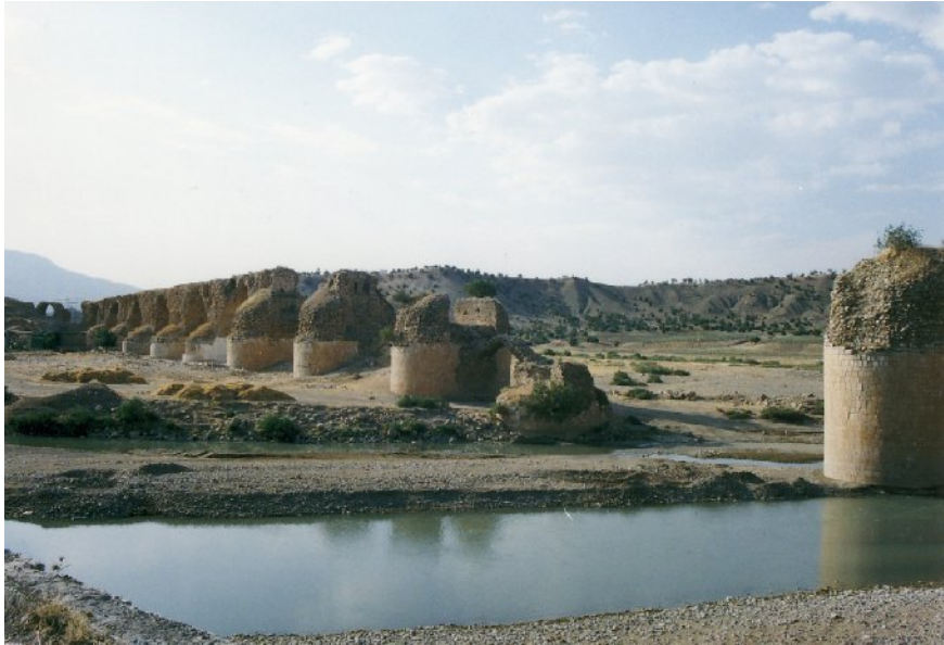
Pl.11.1. Kashkān Bridge. Remains of piers.
