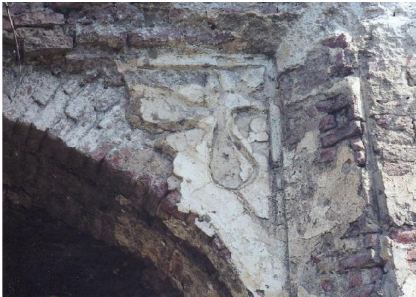
Pl.17.6. Ispī Masjid, Tālīsh. A floral pattern on spandrel of arch.
