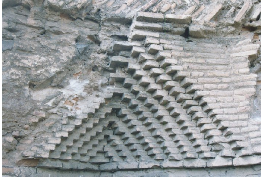
Pl.III.5. Zindān-i Hārūn, near Rayy. View of squinch.
