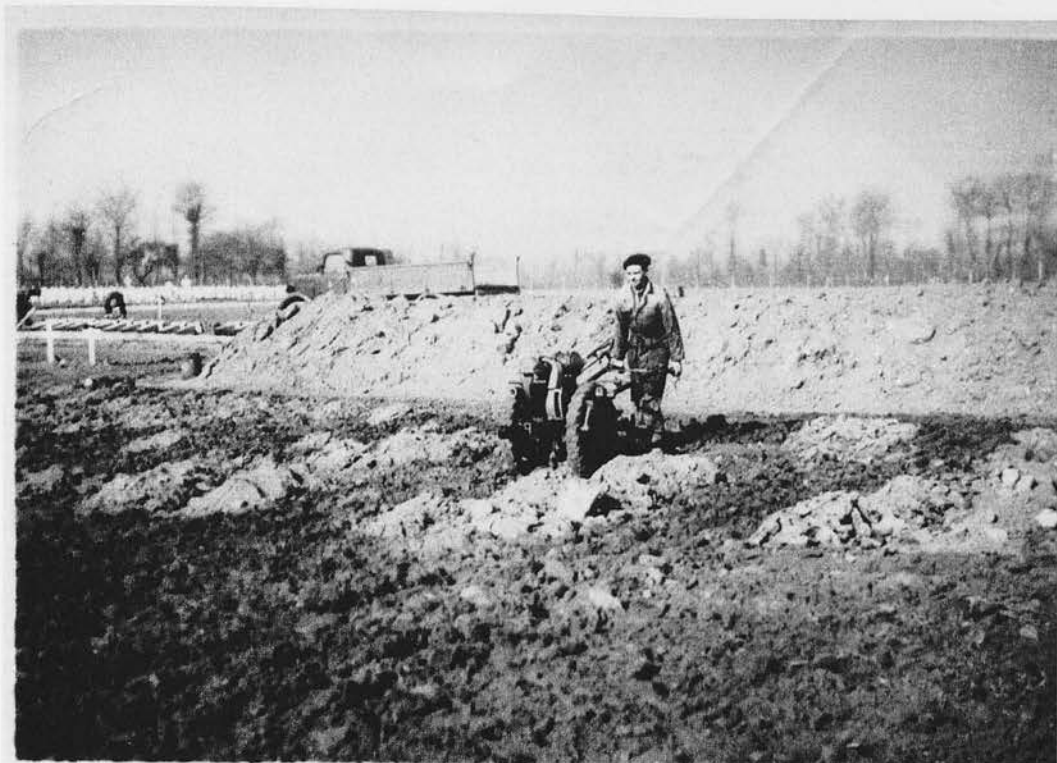
Tilling and levelling the earth.
