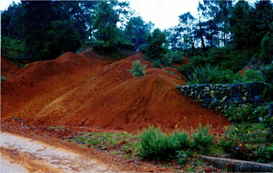
Figure 6.4: Soil erosion around Lago de Zirahuén. Gabions have been put in place in an attempt to prevent further damage. The exposed soil is a distinctive red colour, being highly oxidised.
