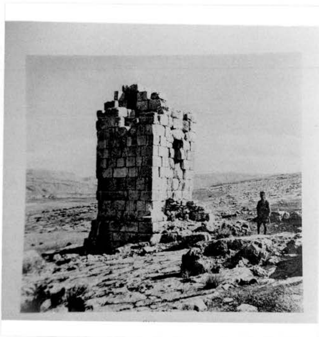
Fig.41. Nourābād: Tower (c. III- I cent. B.C.)
