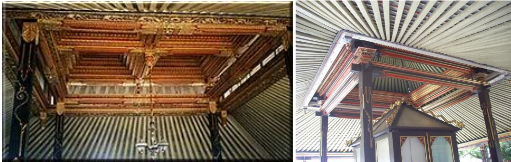
Figure 6.61. The roof structures of Bangsal Witana of the kraton of Yogyakarta (left) and that of the kraton of Surakarta (right). Both of them have tumpangsari and calligraphy ornamented columns. The one of Yogyakarta is more golden in colour while the one of Surakarta is red in colour.
