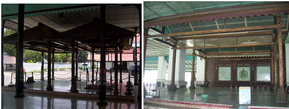
Figure 6.56. Bangsal Pangrawit of the kraton of Yogyakarta (left) and the kraton of Surakarta (right). Both of them have two adjacent roofs and wooden structure.
