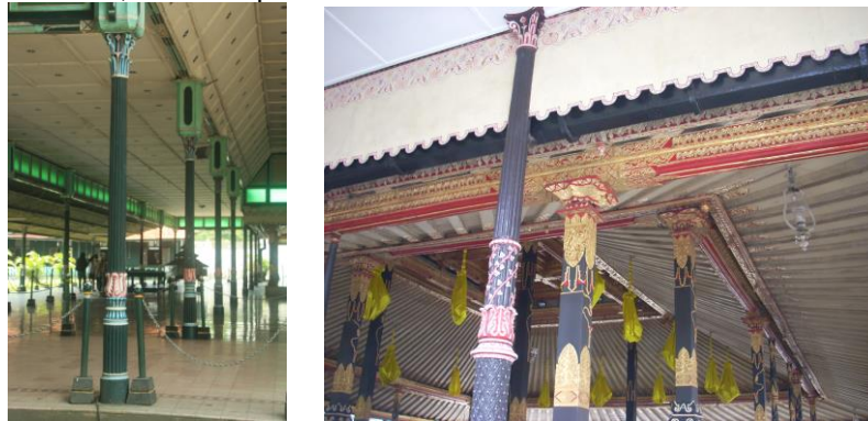
Figure 6.40. The cast iron columns used in the kraton of Yogyakarta. The left image is the columns used in Pagelaran and Sitinggil pavilions while the right image is the column used in Bangsal Kencana, Kedhaton.
