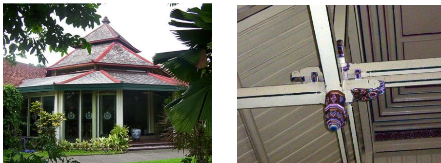
Figure 6.38. Pracimayasa located at the rear of Pura Mangkunegaran, designed by Karsten. The left image is the overall building with three-tiered roof and the right image is one detail of the roof construction.
