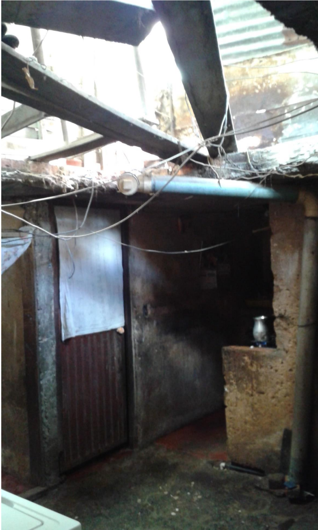
11 – The interior of Vanessa's house. Photograph by the author.
