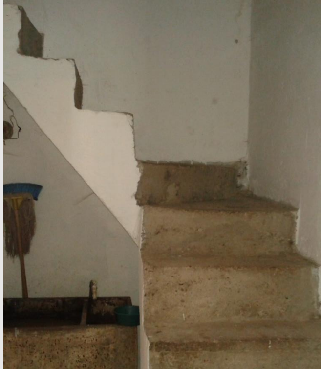
30 – The central stairwell at the foundation. Photograph by the author.
