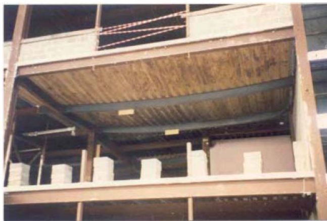
Figure 2.17: Front view of post-test deformation of BS corner test
