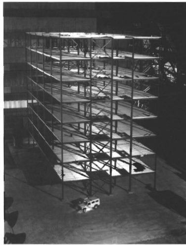
Figure 2.2: General view of Cardington test building (British Steel, 1999)
