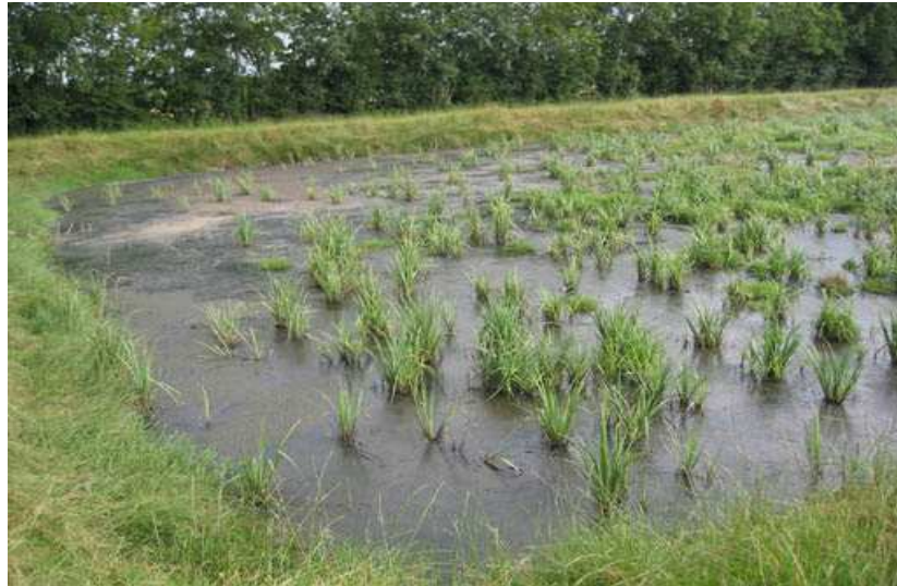
Figure 3-3. Establishment of Carex riparia in an integrated constructed wetland cell (photo from Dr Rory Harrington).
