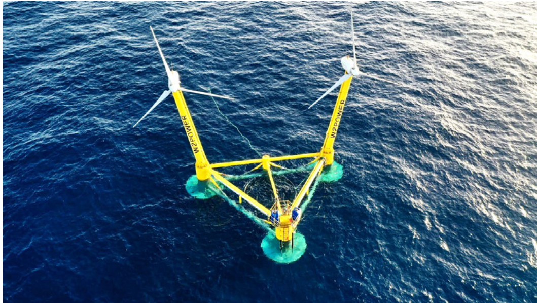
Figure 1.3: The W2Power prototype (i.e. at a scale of 1:6) in the open sea at Plocan in Gran Canaria, November 2022. Photo courtesy of EnerOcean S.L.
