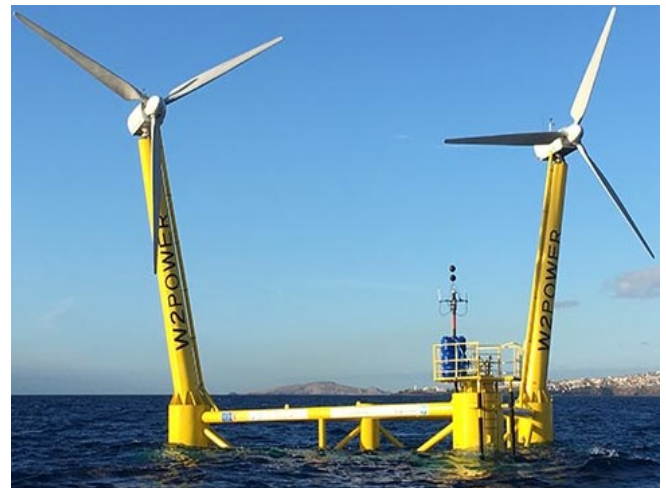
FIGURE 1: W2POWER PLATFORM PROTOTYPE DURING 2019 SEA TESTS. PHOTO COURTESY OF ENEROCEAN.
