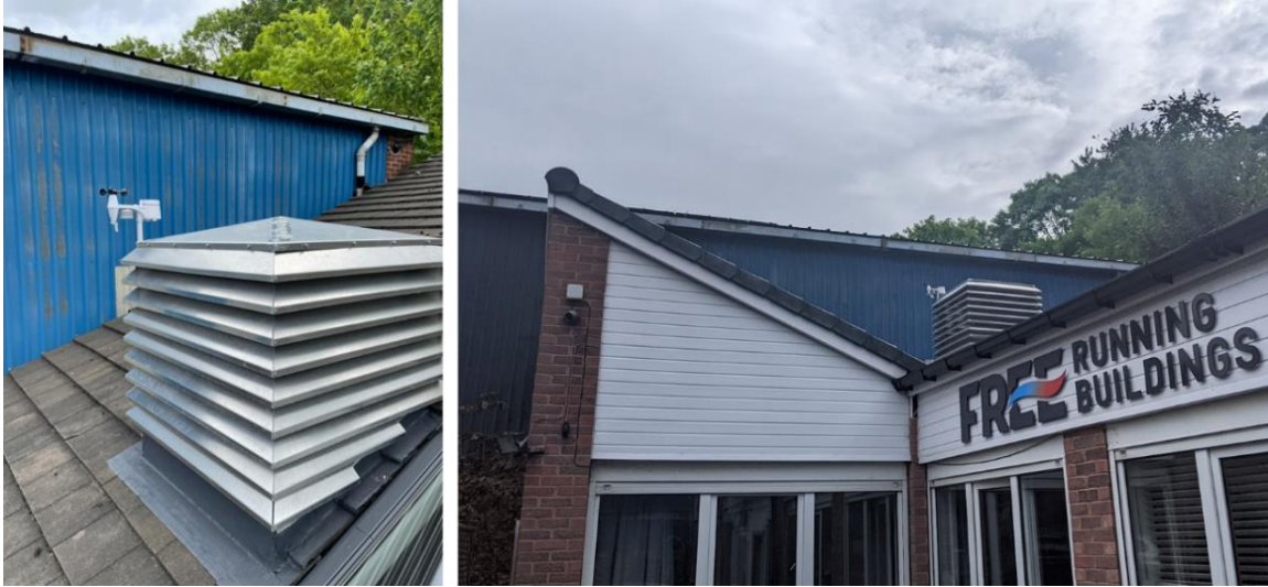
Figure 5-2 - Wind tower installation through the office roof
