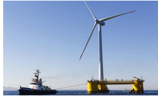
(b) Turbine towing example, Source: WindEurope (OffshoreWIND biz, 2023b)
