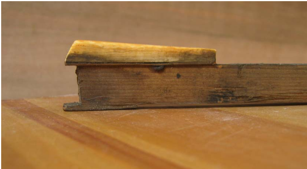
Plate 1143 – The 1704 Keene Spinnet – Shimmed Sharp Block
