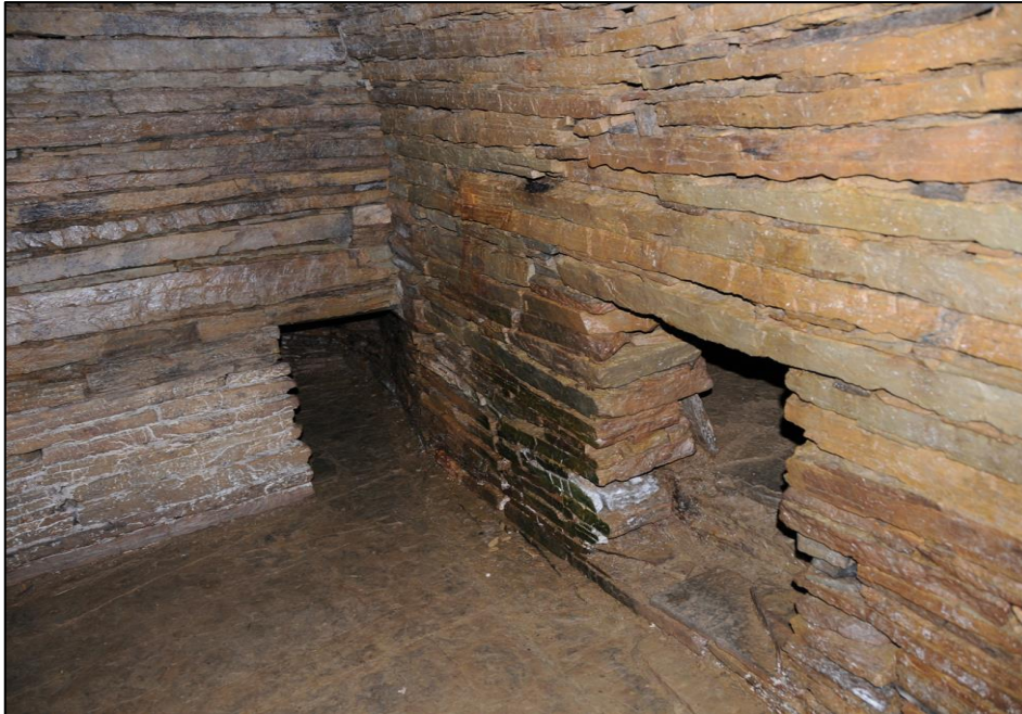
Figure 2.1 (above) Interior of the Neolithic chambered tomb at Cuween Hill, Firth, showing excellent quality stone work constructed of Upper Stromness Flags.
