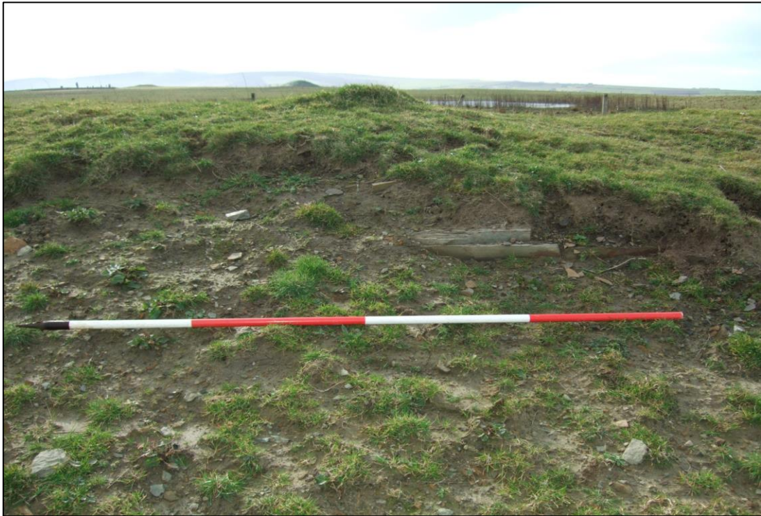
Figure 8.15 (above) Stone core of the Dyke of Sean revealed by erosion and cattle damage.
